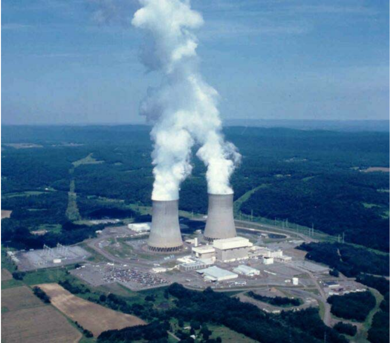
Susquehanna Steam Electric Station, Luzerne County, Pennsylvania
