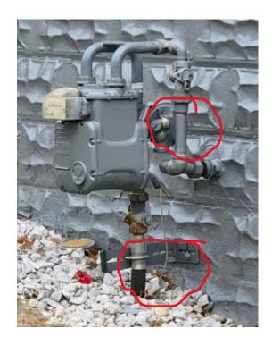
The top circle is the gas pressure regulator – this was the device not placed by the meter at 100 Park Lane
