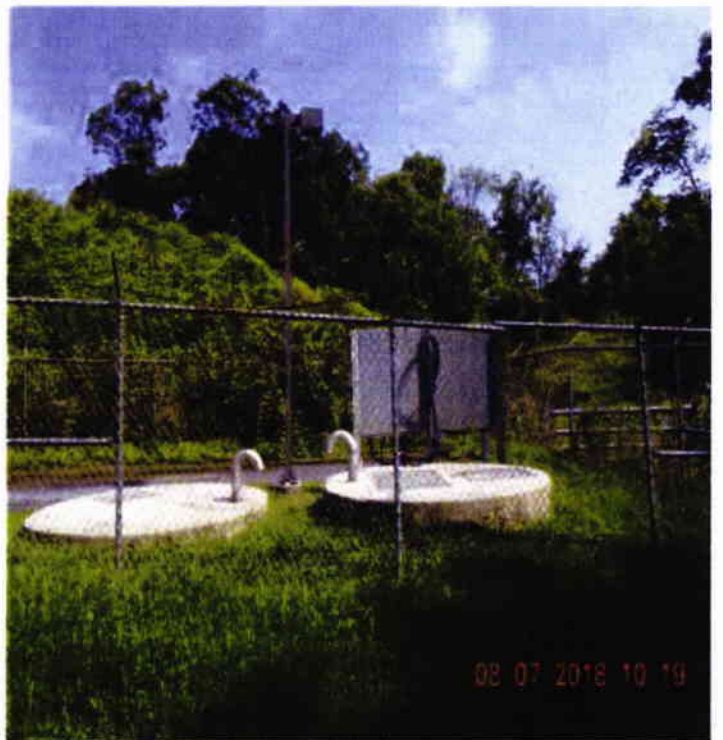
Baumstown Pump Station
