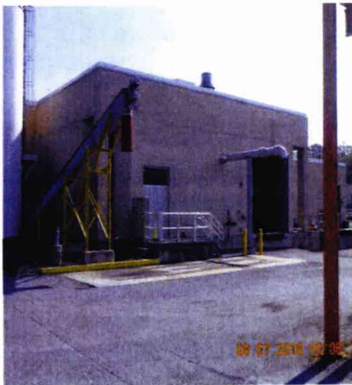
Sludge Drying Building
