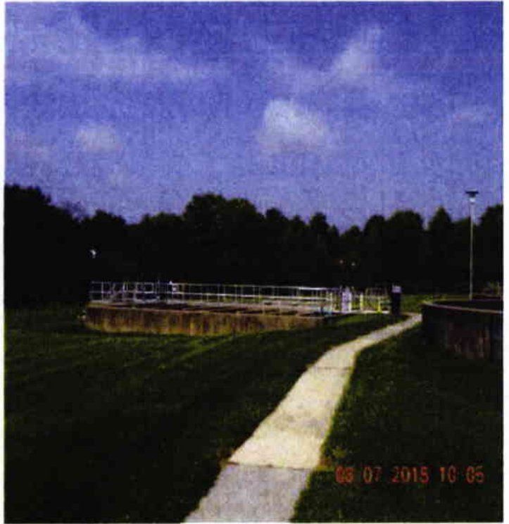
Chlorine Contact Tank
