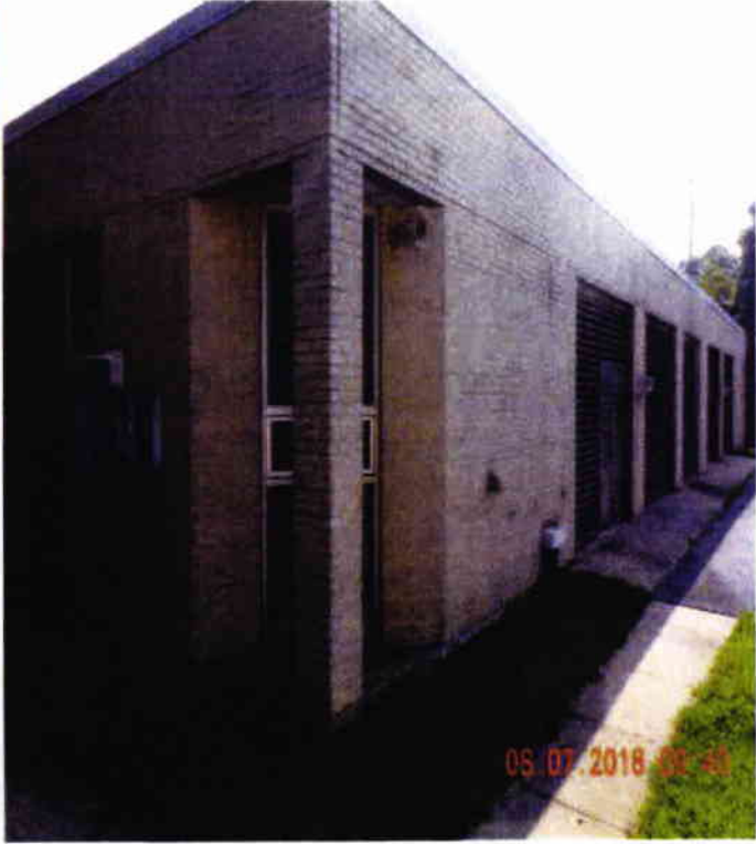
Back-up Power Bldg.
