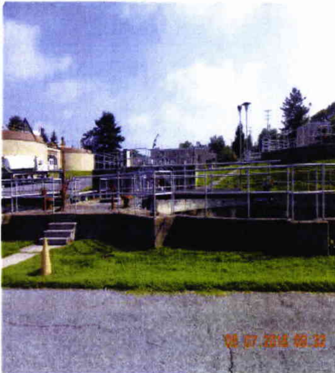
Original Clarifier (not used)
