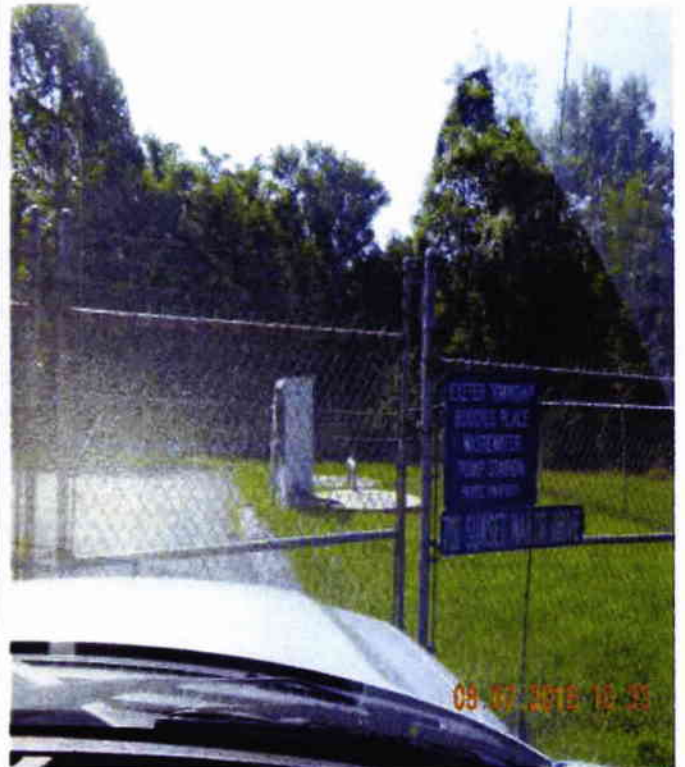
Buddies Place Pump Station
