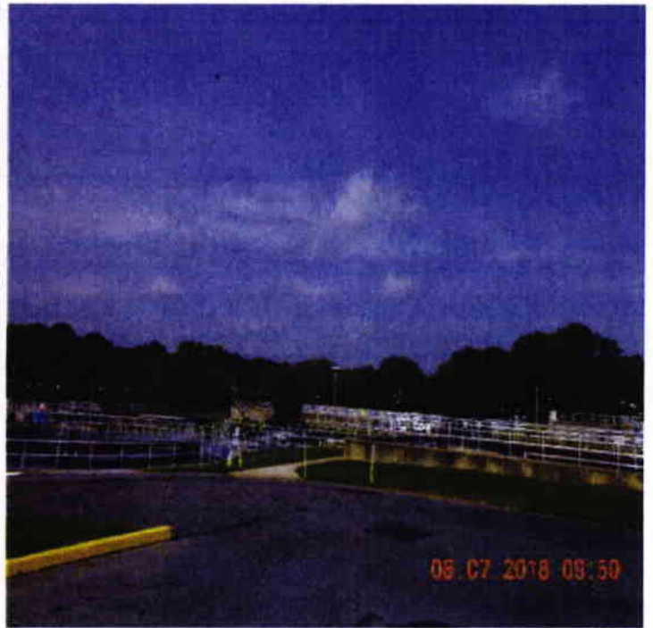
Overview Clarifiers & Diversion Box
