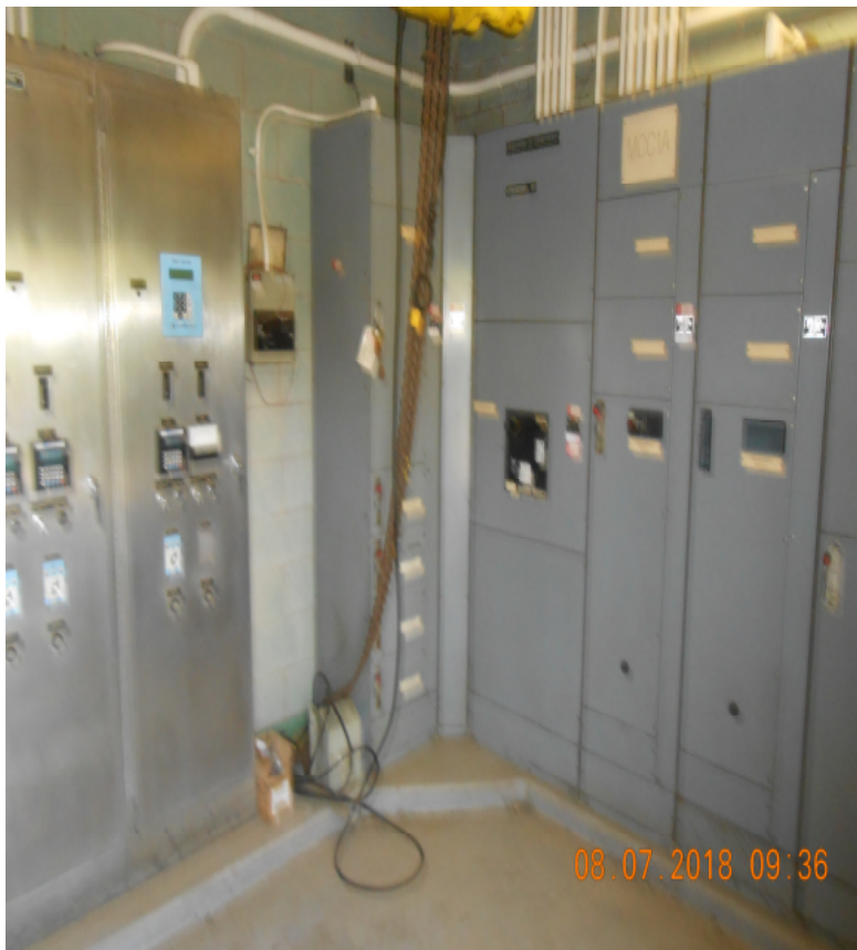
Original Construction – Wet Well Control Panel
