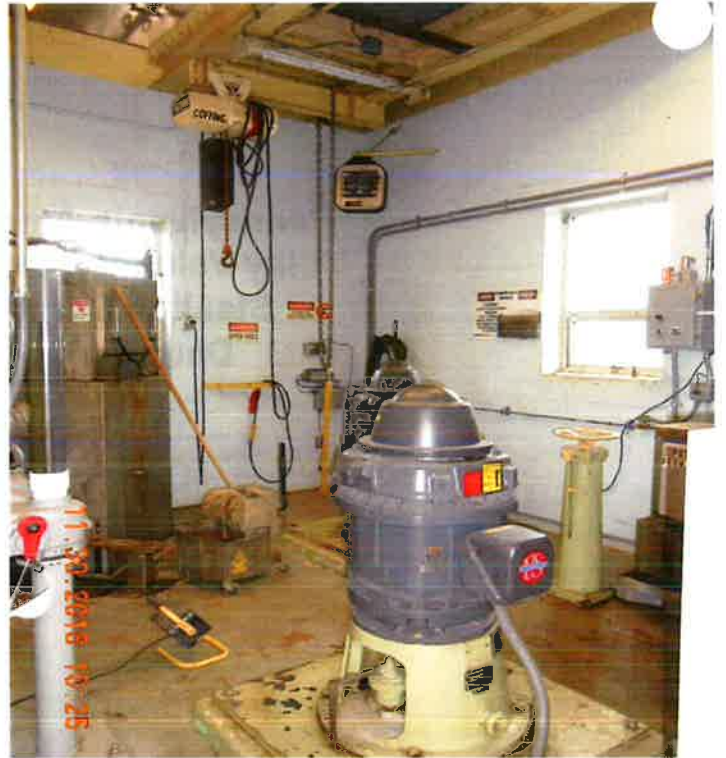
Raw Water Station (1973)
