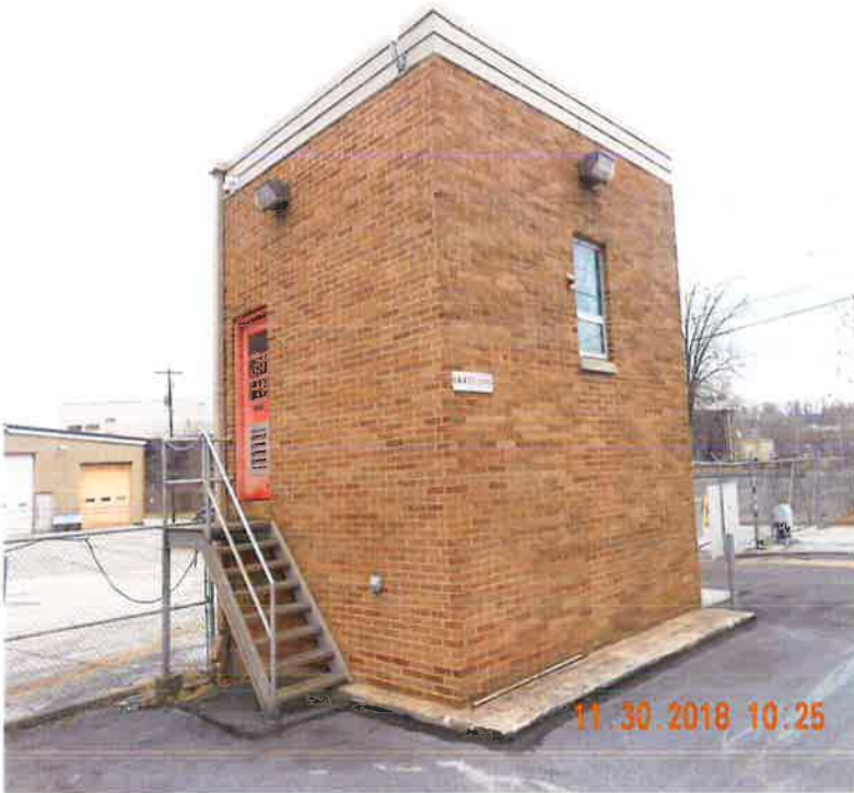
Raw Water Station (1973)
