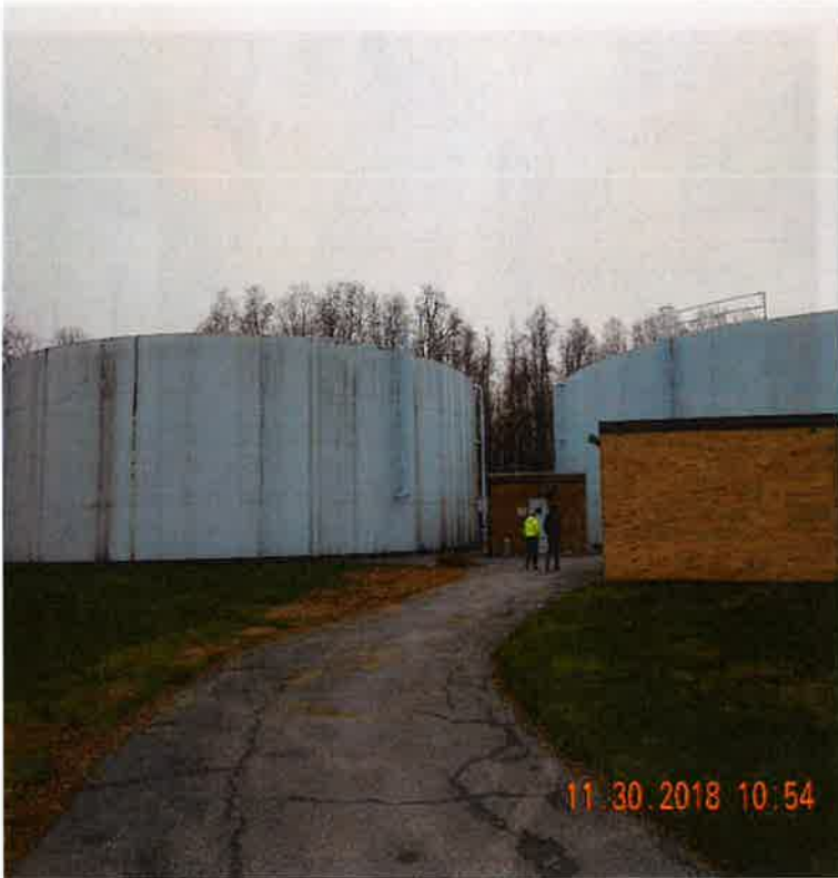
2 Million Gallon Tanks
