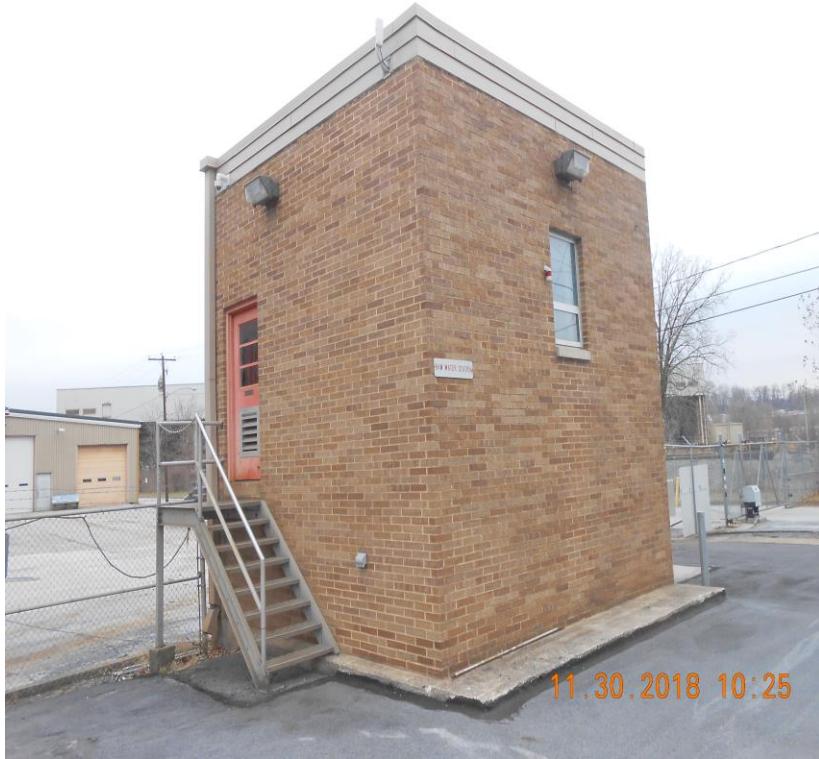
Raw Water Station (1973)
