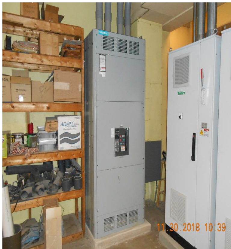
Piping Gallery & Booster Pumps Page 5 of 7
