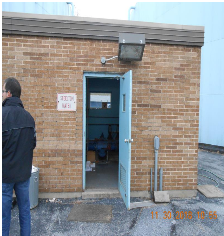
Tank Booster Pump Building
