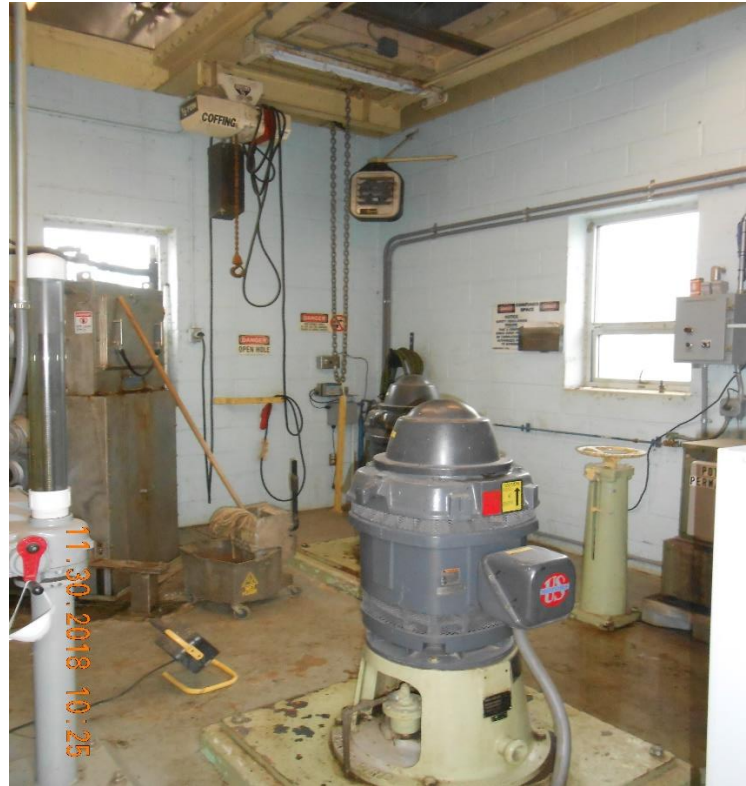
Raw Water Station (1973)
