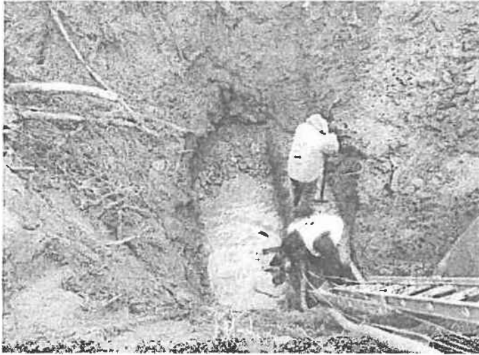
17. The excavation of the 16 inch force main, 02/25/16.
