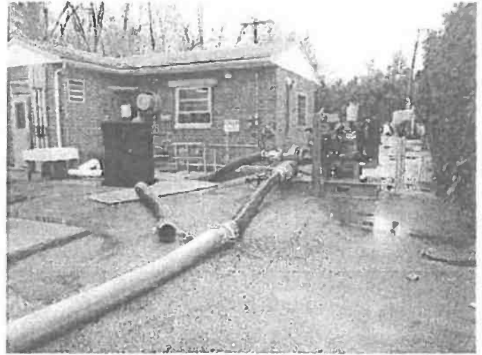
6. The Xylem Pump set up and discharging from the wet well, 02/25/16.
