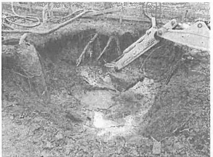
12. The excavation of the 16 inch force main with a back-hoe.
