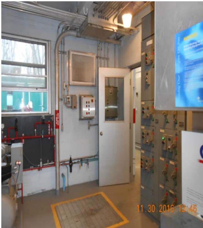
East Norriton Inspections Norris City Pump Station
