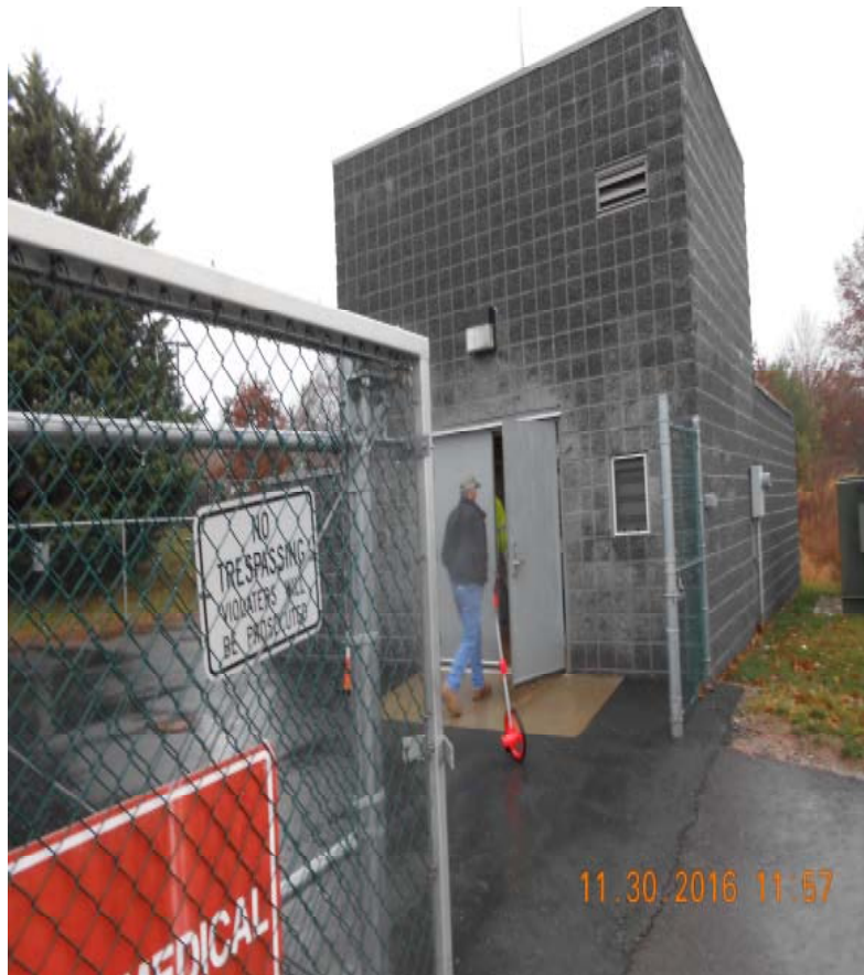
Einstein Pump Station
