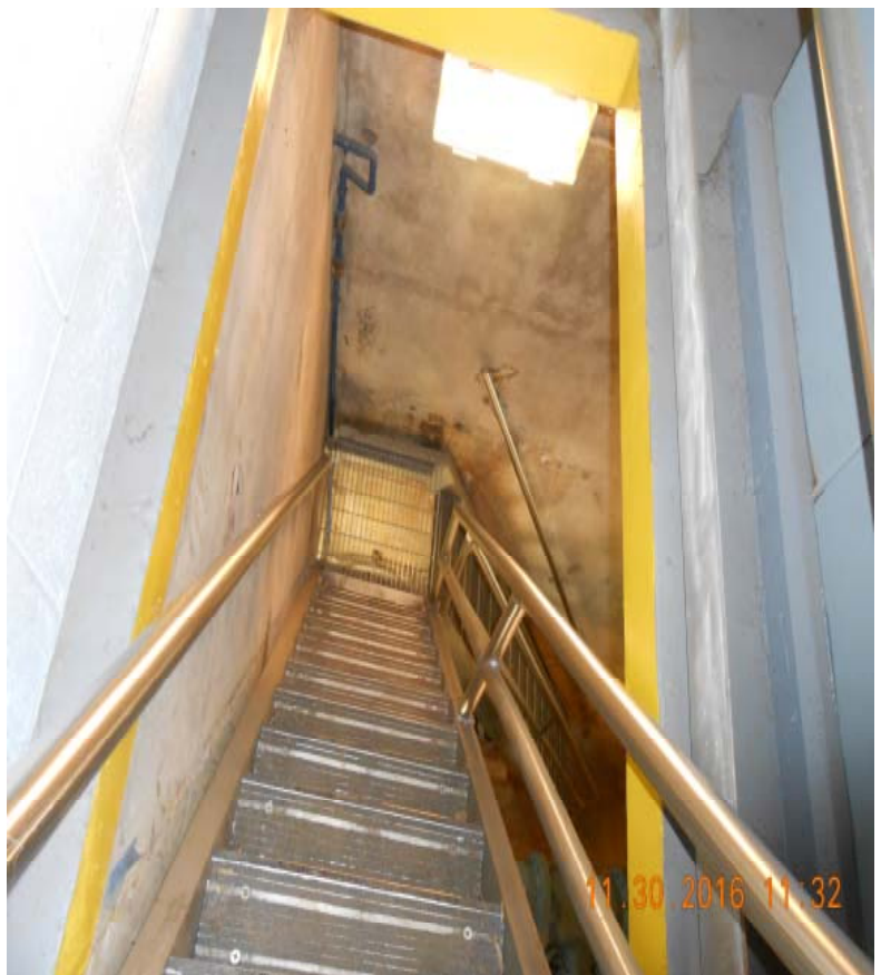
Germantown Pike Pump Station
