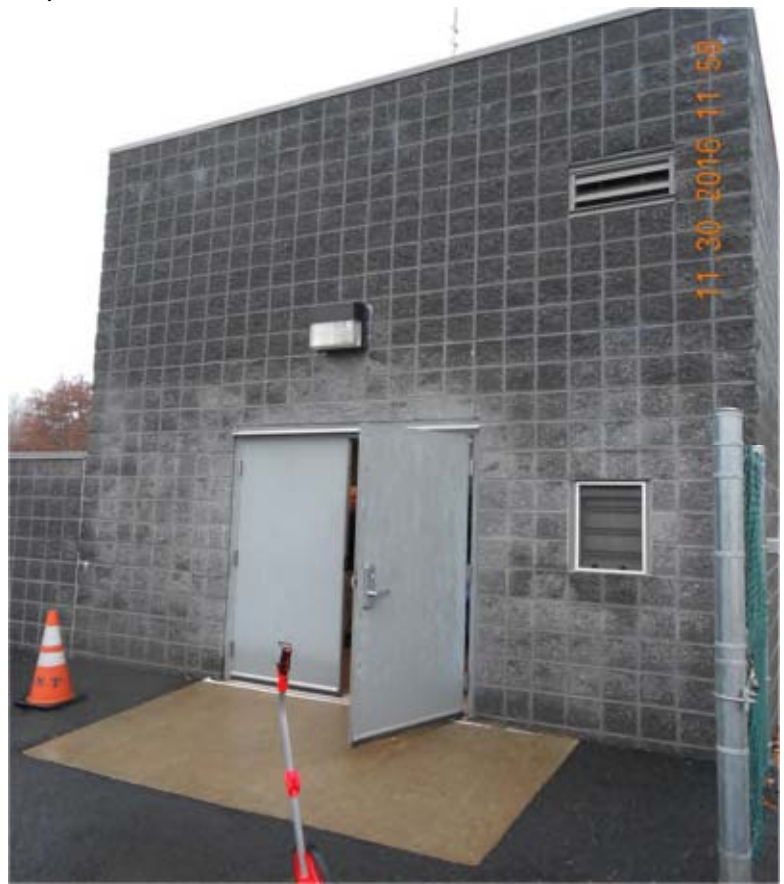
Einstein Pump Station
