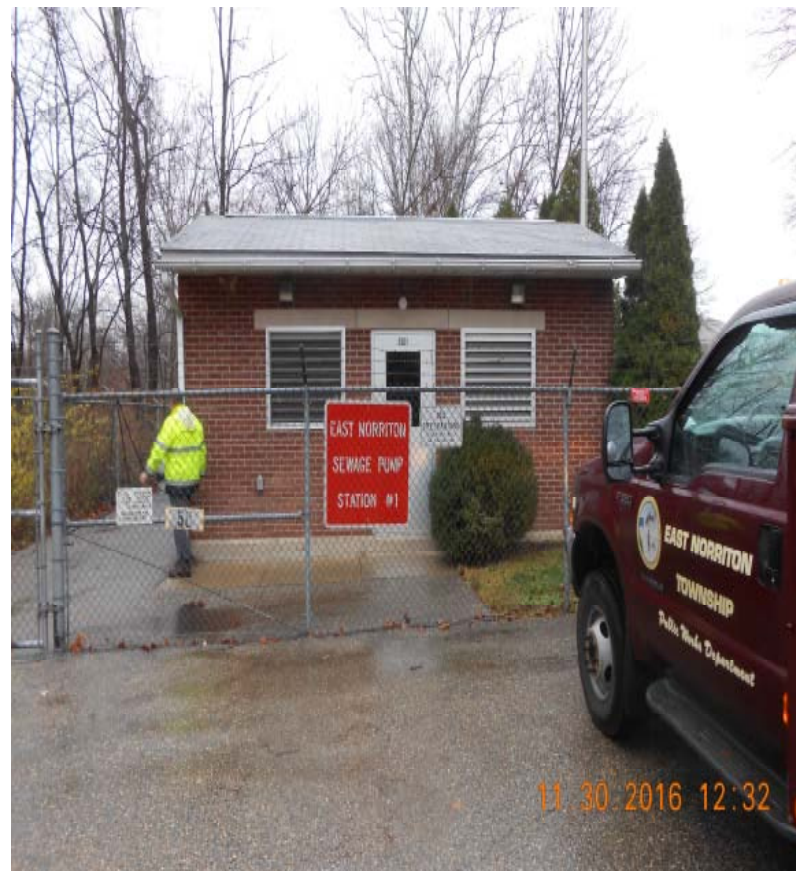
Timberlake Pump Station
