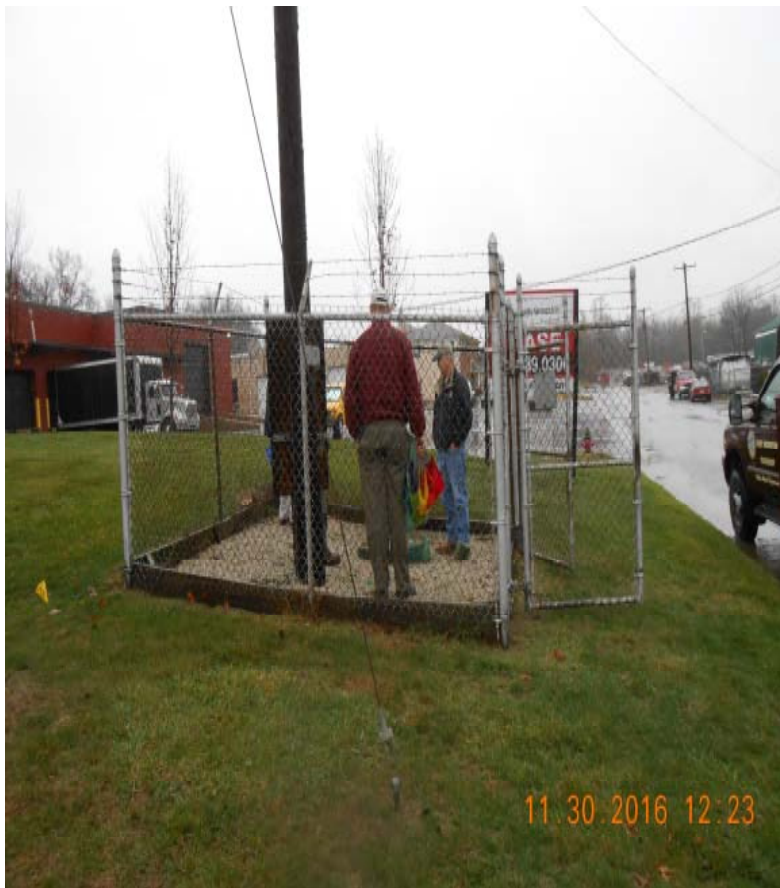
Felton Road Pump Station
