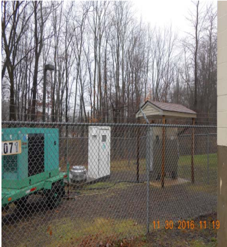
Burnside Ave. Pump Station
