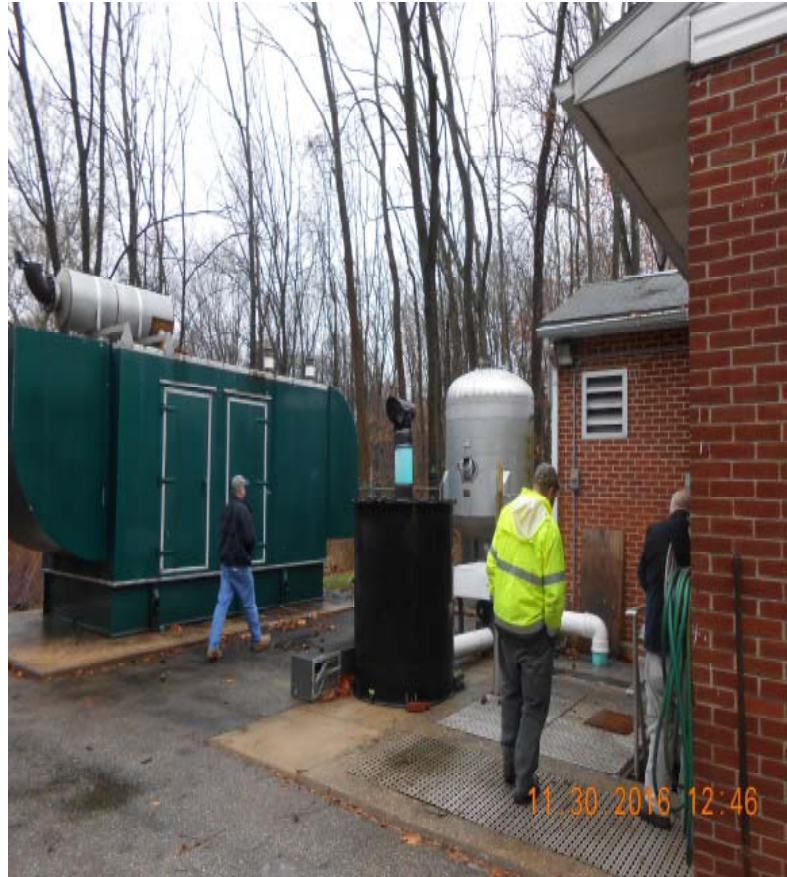
Norris City Pump Station
