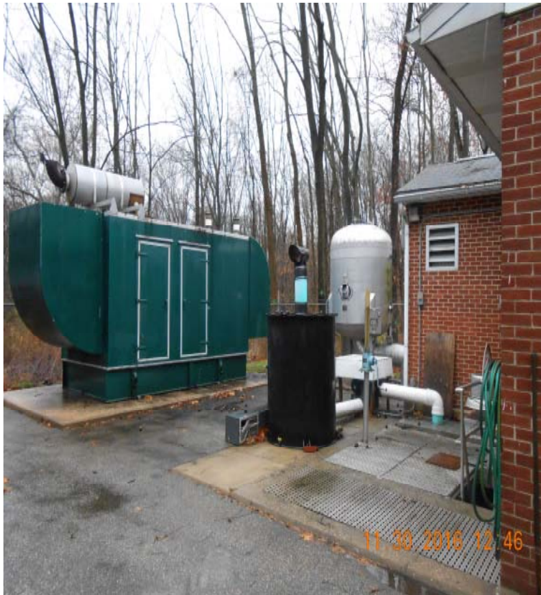
Norris City Pump Station
