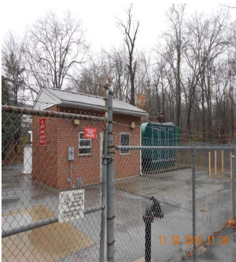
Germantown Pike Pump Station
