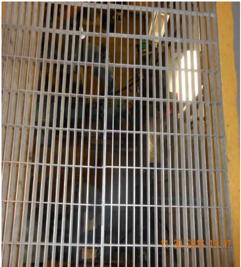
Norris City Pump Station
