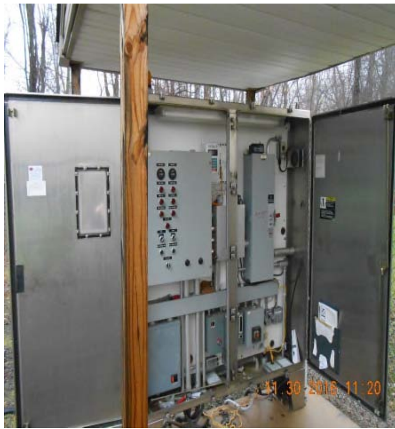
Burnside Ave. Pump Station
