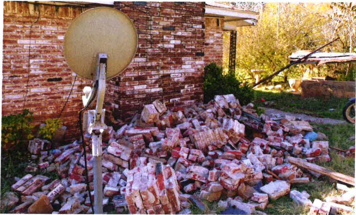
A house in central Oklahoma was damaged by a magnitude 5.6 earthquake on Nov. 6, 2011, that was linked to injection into deep wastewater disposal wells. Credit: Brian Sherrod *USGS*
