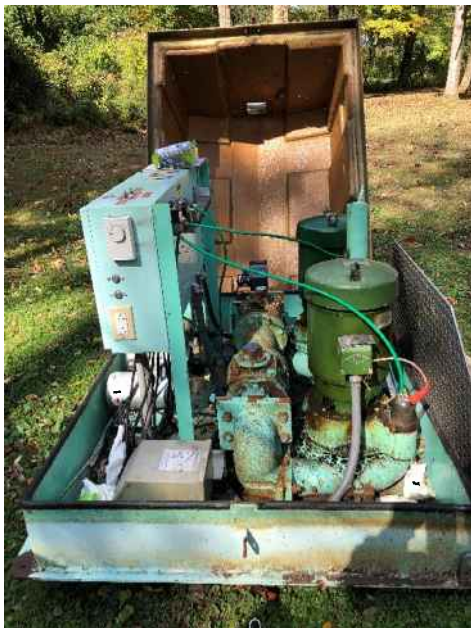
Figure 3 – Elect. Controls and Pumps
