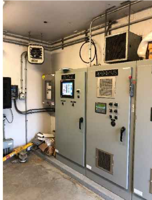
Figure 4 – Pump Controls
