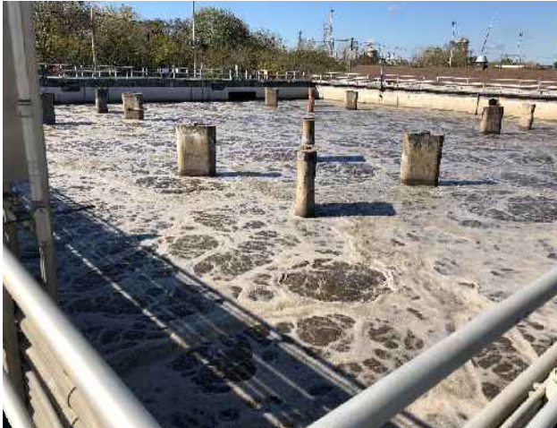
Figure 1 – Aeration Tank
