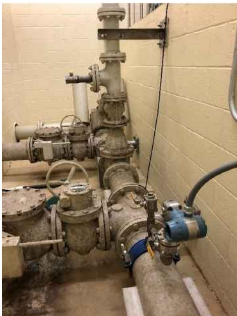
Figure 7 – Discharge Pipe Layout
