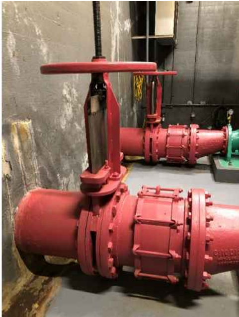
Figure 9 – Pump Gate Valves
