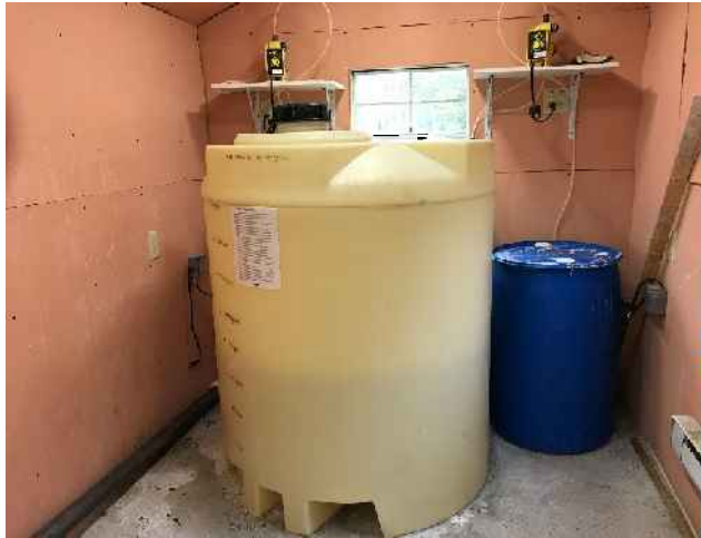
Figure 5 -Liquid Alum Tank
