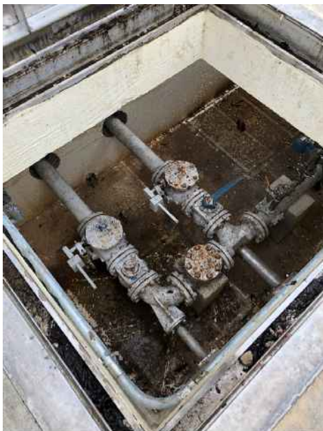
Figure 3 – Valve Vault
