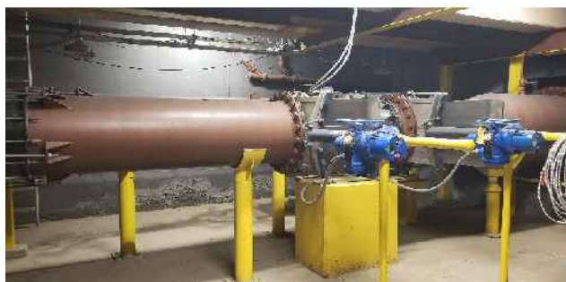
Figure 9 – Knife Gate Valve
