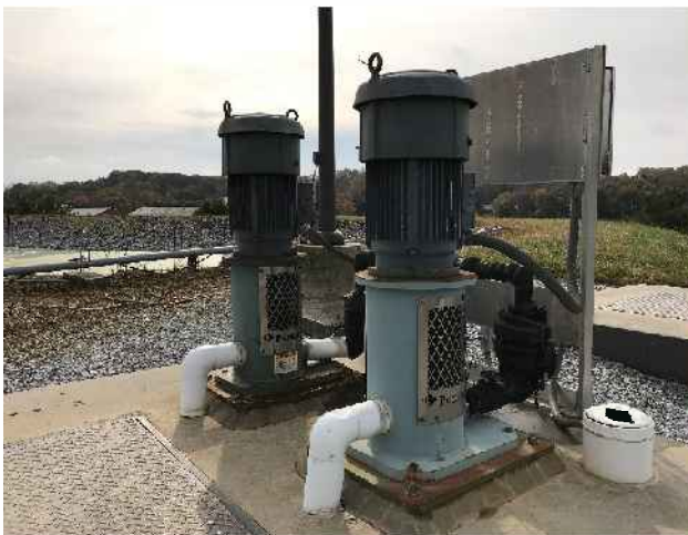
Figure 3 – Drip Irrigation Pumps
