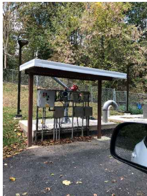
Figure 8 – Elect. Panels with Roof Structure
