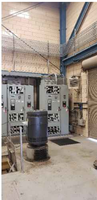
Figure 7 – Pump Motor / MCC
