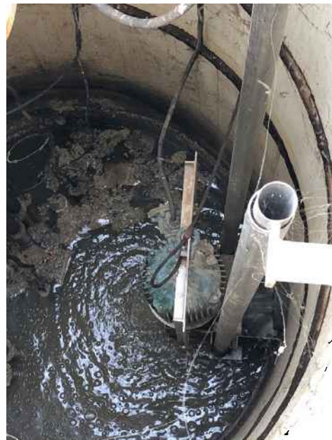
Figure 4 – Grinder in Wet Well
