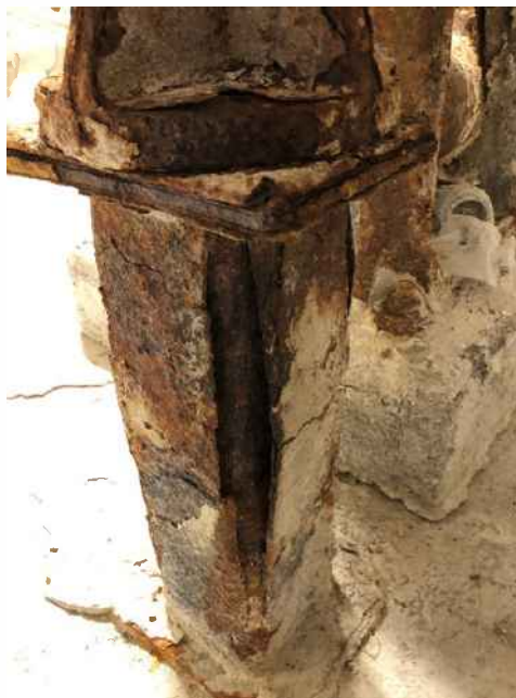
Figure 10 – Corroded Pipe Supports
