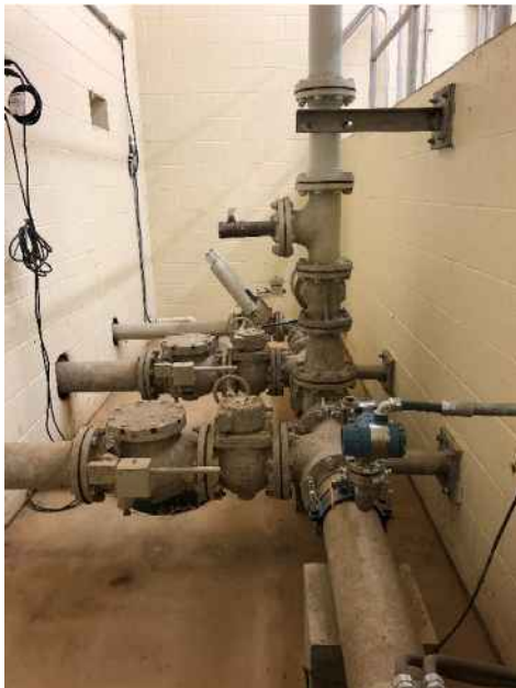
Figure 7 – Discharge Pipe Layout
