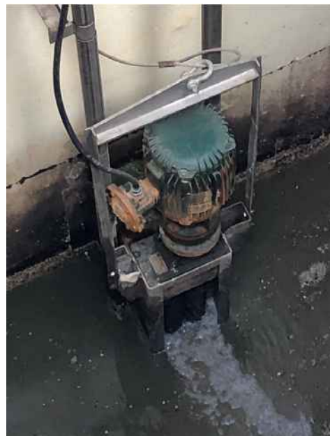
Figure 8 – Grinder in Wet Well
