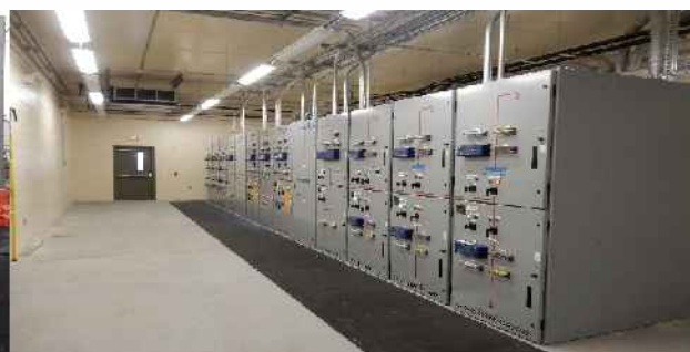
Figure 10 – Plant's Main Incoming Power Switchgear
