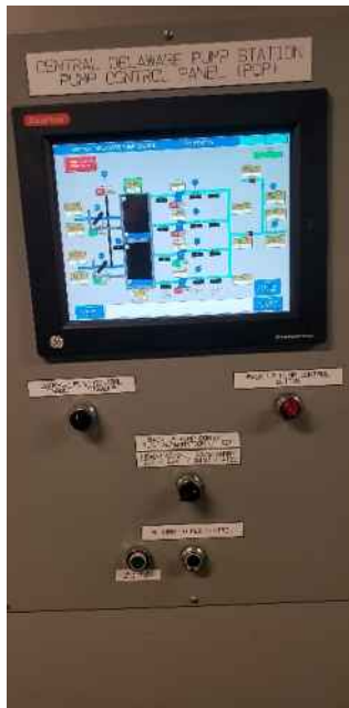
Figure 9 –Pump Control Panel
