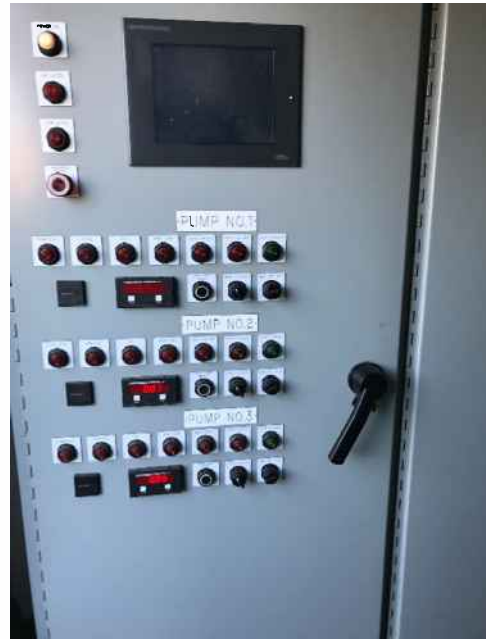
Figure 6 – Pump Control Panel
