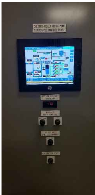
Figure 7 – SCADA / Pump Monitor Display
