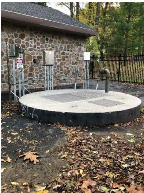
Figure 3 – Top Slab of Wet Well
