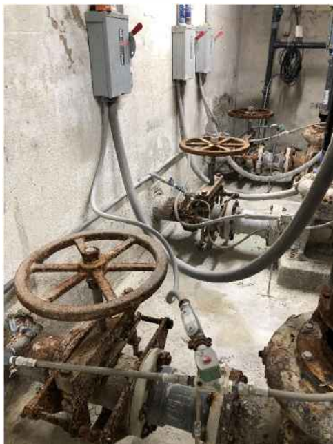
Figure 9 – Pump Gate Valves
