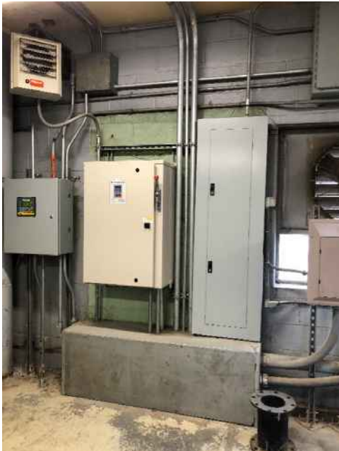
Figure 5 – Pump Controls & Electrical Panel
