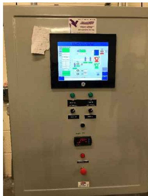
Figure 8 - Drip Irrigation Control Panel
