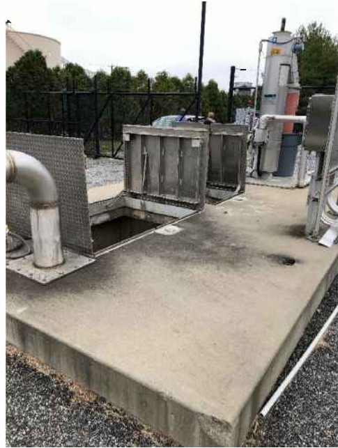
Figure 6 - Pump Wet Well & Valve Pit
