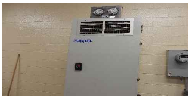
Figure 11 – H2S Removal System
