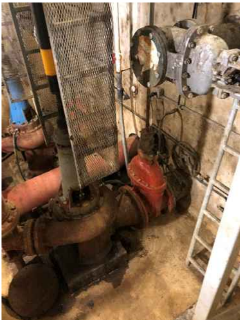
Figure 7 – Pump & gate Valve
