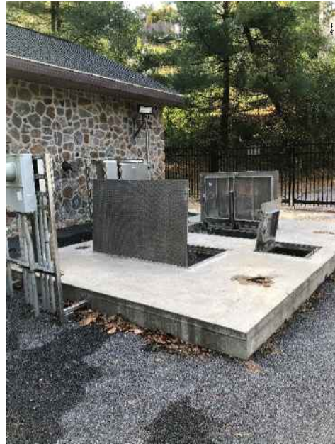
Figure 2 – Top Slab of Wet Well
