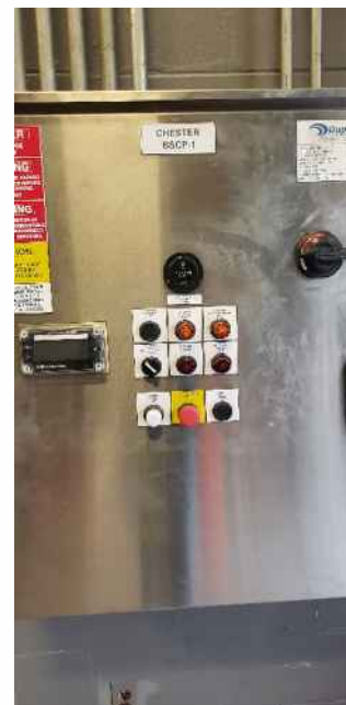
Figure 8 – Bar Screen Control Panel
