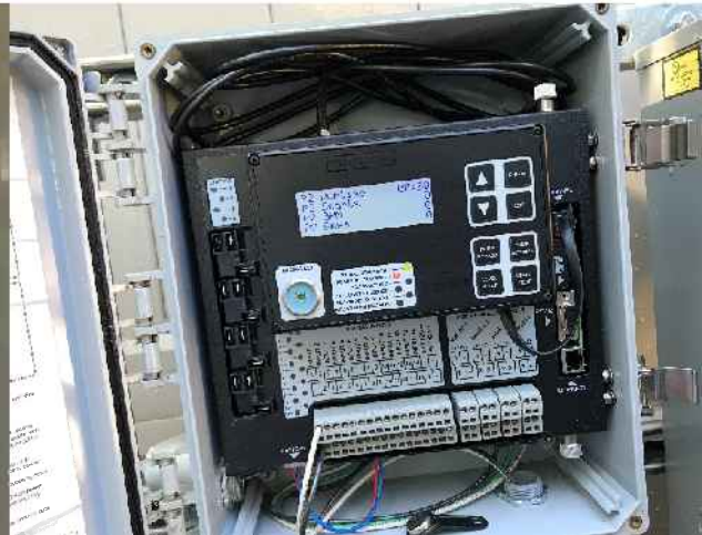
Figure 2 – Omni Site Pump Monitor
