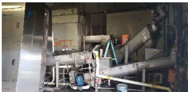
Figure 1 – Bar Screen Discharge
