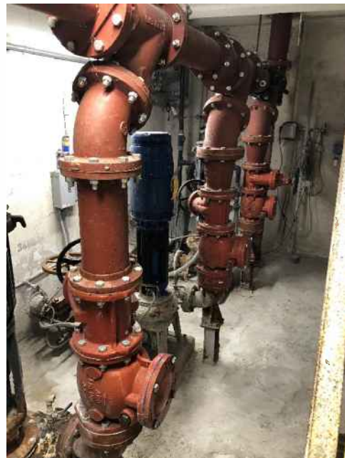
Figure 8 – Pumps & Pipe Manifold
