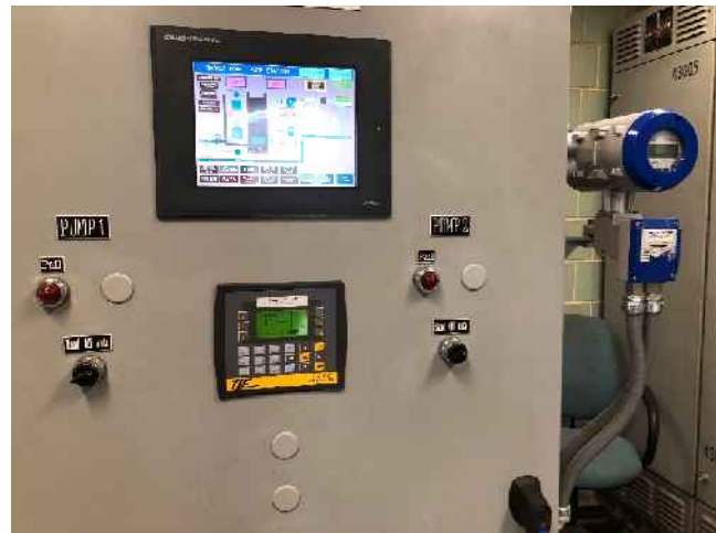
Figure 8 – Pump Control Panel
