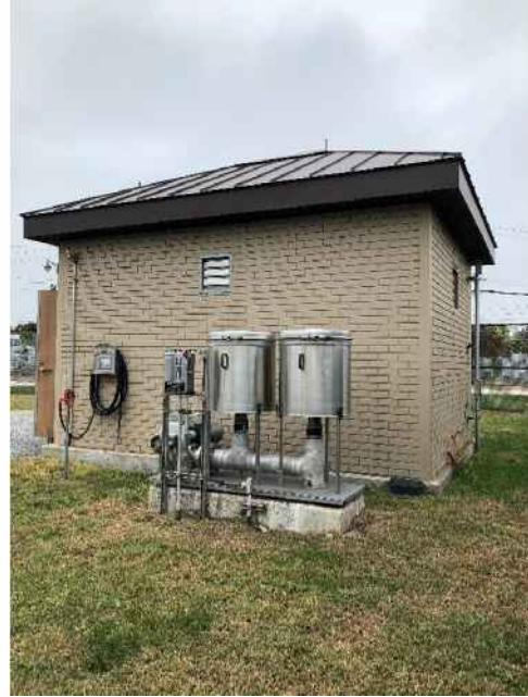
Figure 2 – Odor Controls
