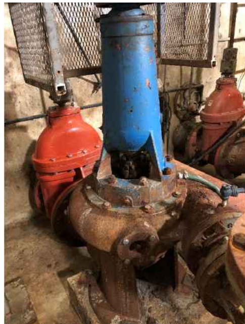
Figure 8 – Pump & Gate Valve
