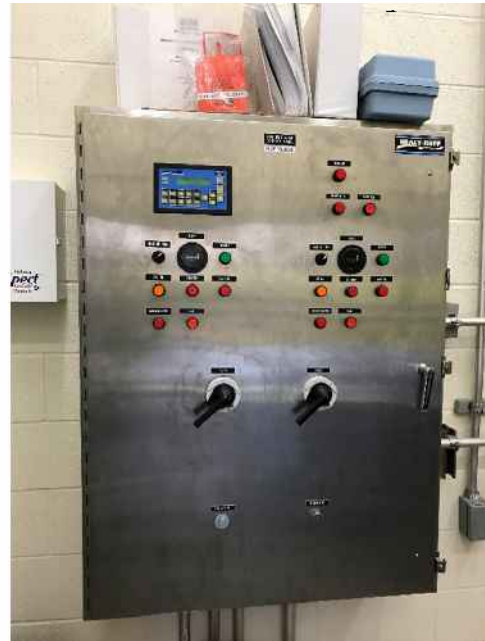
Figure 2 – Pump Control Panel
