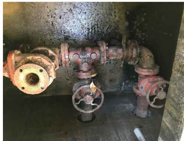
Figure 4 – Gate Valves & By-Pass Connection
