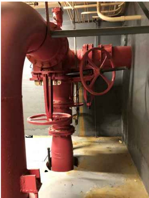
Figure 11 – Discharge Pump
