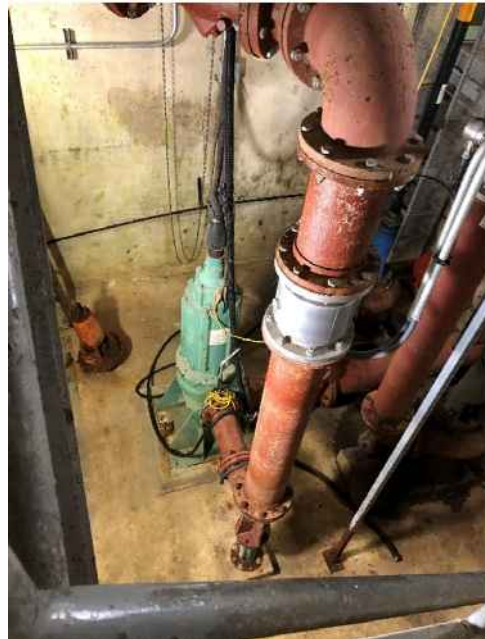
Figure 6 – Dry Pit Dumps
