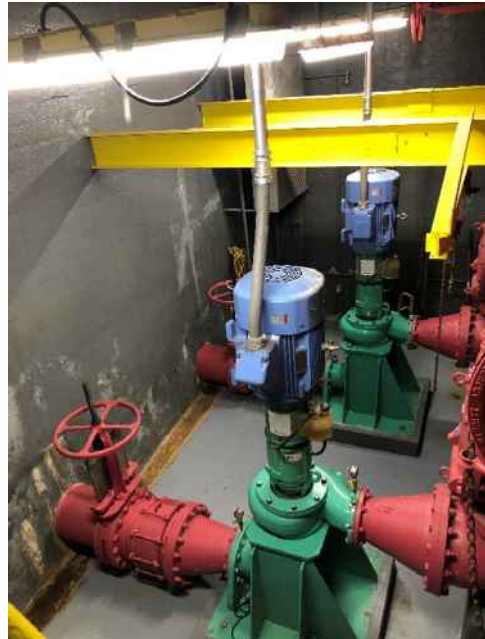
Figure 10 - Dry Pit Pump
