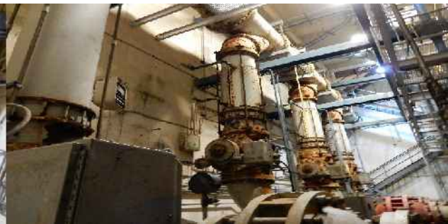
Figure 12 – Discharge Manifold
