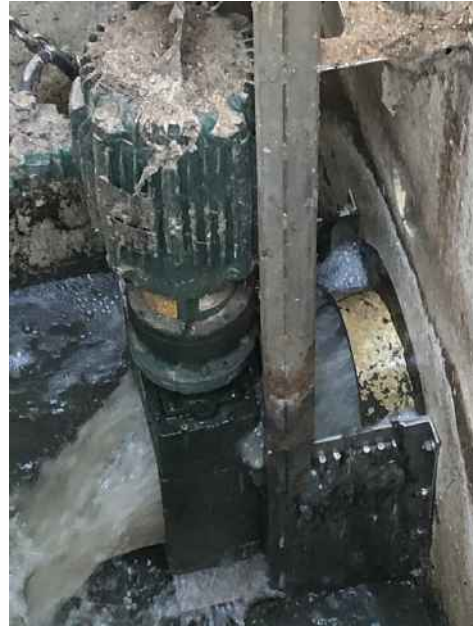
Figure 6 – Grinder in Wet Well
