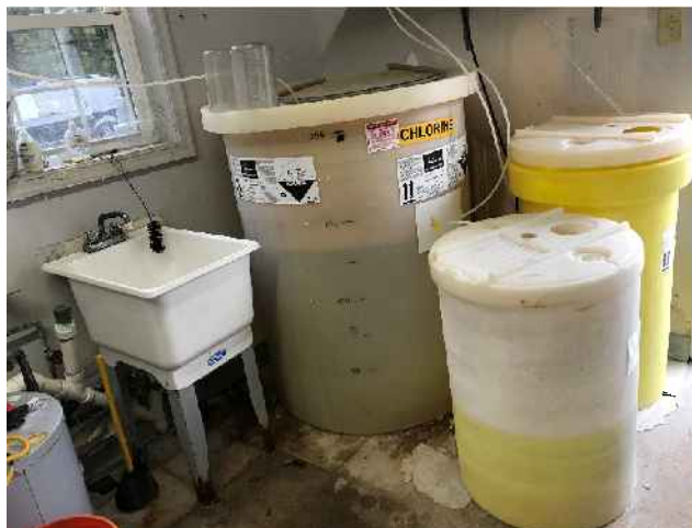
Figure 13 – Sodium Hypochlorite Storage Tank
