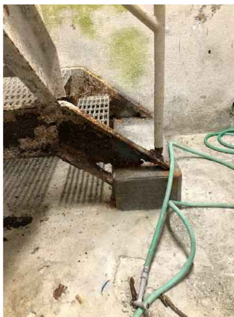
Figure 12 – Corroded Stairs
