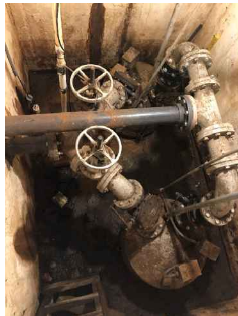
Figure 4 – Ejector Piping and Tanks
