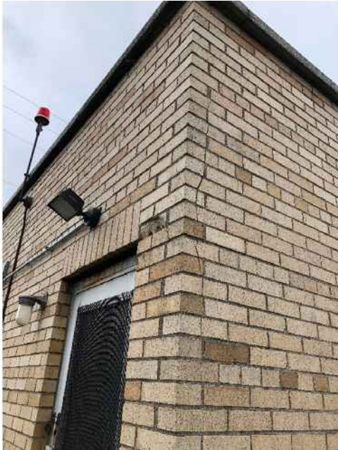
Figure 3 – Crack in Wall
