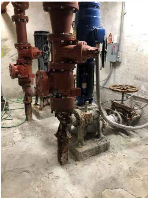
Figure 7 – Pumps in Dry Pit
