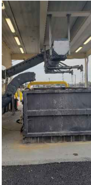
Figure 5 – Screenings Disposal
