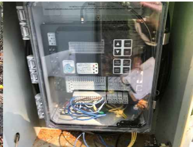
Figure 8 – Omni Site Pump Monitor
