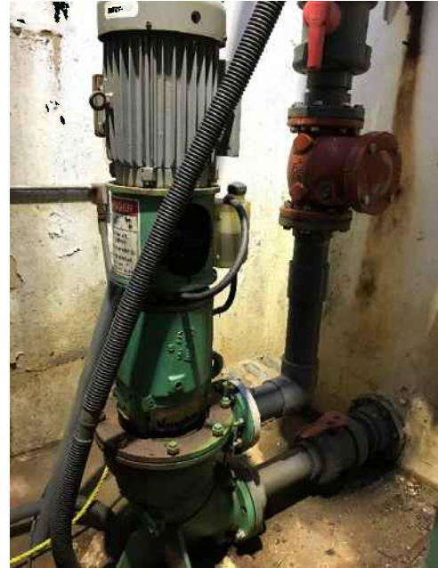
Figure 4 – Pump and Motor in Dry Pit
