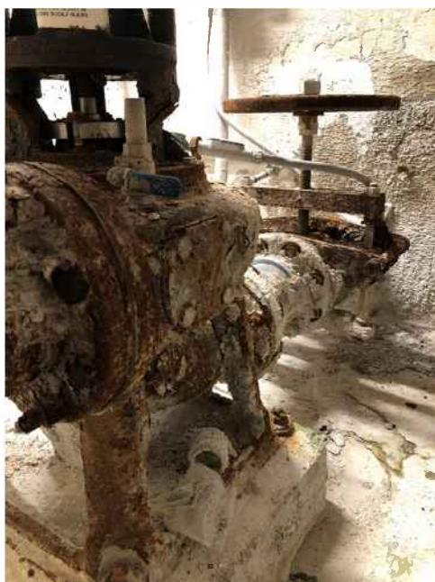
Figure 11 – Corroded Pump Housing
