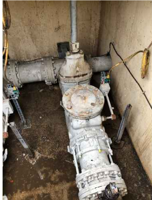
Figure 8 – Check & Gate Valves
