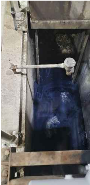
Figure 9 – Ultrasonic Flowmeter
