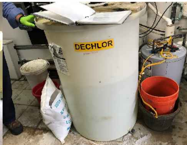
Figure 14 - Sodium Thiochlorite Storage Tank
