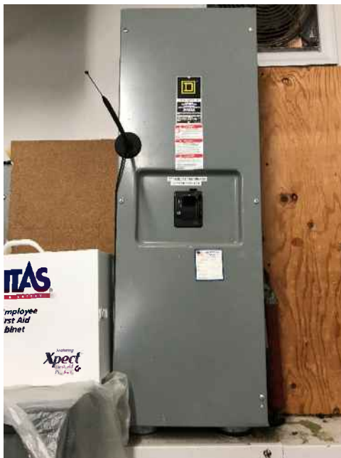
Figure 11 - Electrical Main Panel
