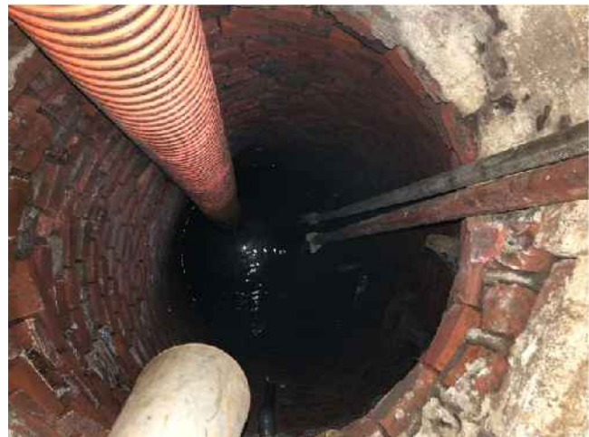
Figure 4 – Manhole & Pump Suction
