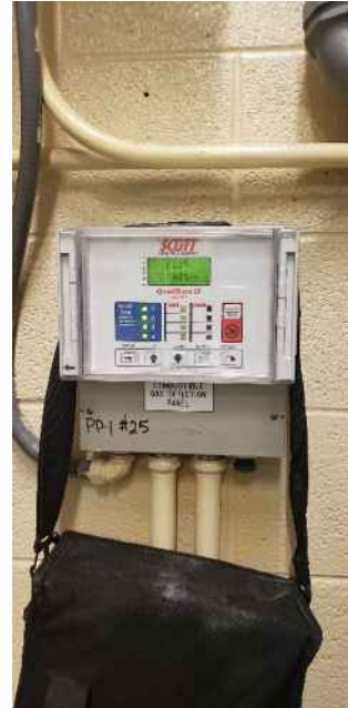
Figure 4 – Gas Detector Panel
