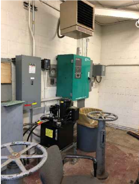
Figure 3 – Electric AC Main, ATS & Grinder Hydraulic Unit
