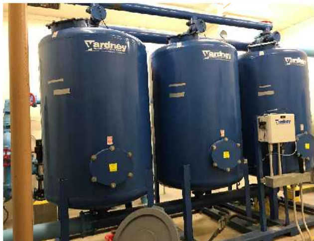
Figure 5 -Sand Filters
