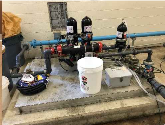
Figure 10 - Drip Irrigation Filters
