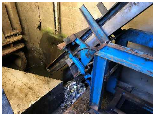
Figure 8 – Influent Chamber, Bar Screen
