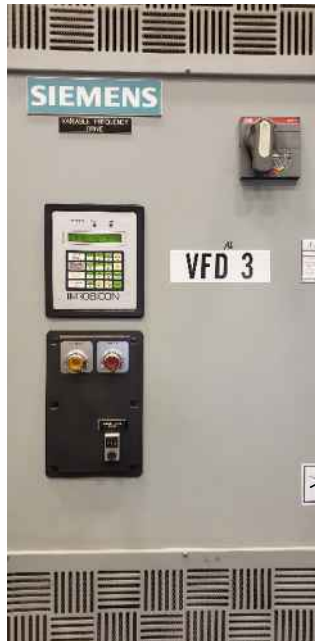
Figure 9 – VFD Controls
