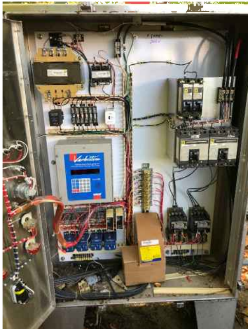
Figure 3 – Pump Control Panel
