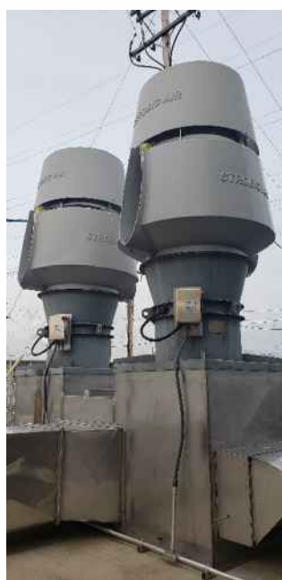
Figure 3 – Odor Control Fans
