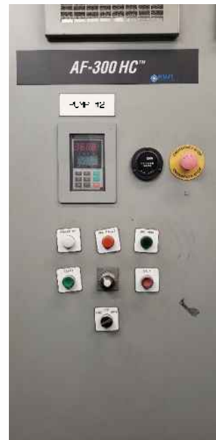
Figure 6 – Pump Control Panel
