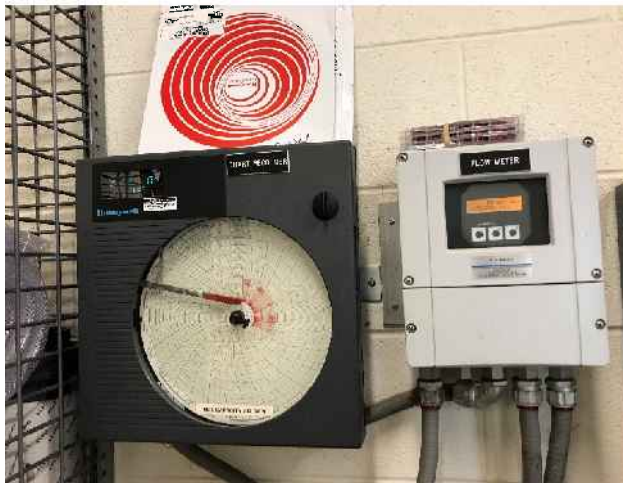
Figure 11 – Flow Meter Readout & Chart Recorder
