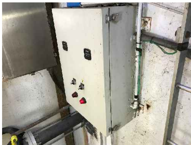
Figure 6 – Pump Control Panel
