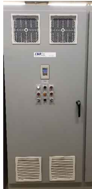
Figure 6 - VFD / Pump Control
