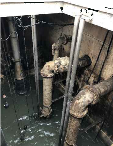
Figure 7 – Pump Wet Well
