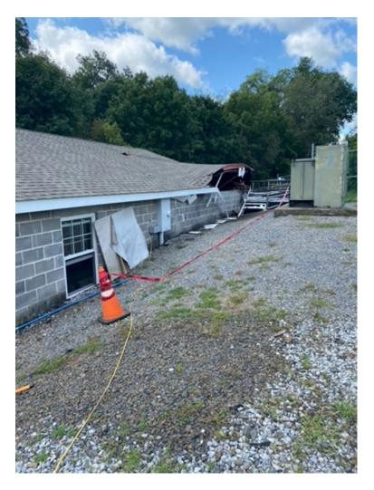
CONTROL BUILDING ROOF DAMAGE DUE TO THE FLOATING OF THE RAPID SAND FILTER TANK / ULTRAVIOLET DISINFECTION SYSTEM IN ABOUT HALF OF THE BUILDING.
