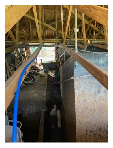
LOOK INSIDE THE CONTROL BLDG. FROM DAMAGED ROOF OPENING. FLOATED TANK IN RIGHT FOREGROUND.
