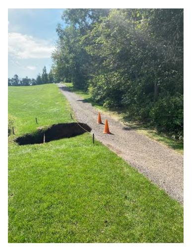
SINKHOLE LOCATION ON GOLF COURSE PROPERTY OVER TOP OF CULVERT. NHSC PROPERTY LINE AT WOODS/FENCE LINE TO THE RIGHT. EARTH WASHED INTO THE COLLAPSED CULVERT SUBSTANIALY BLOCKING IT.
