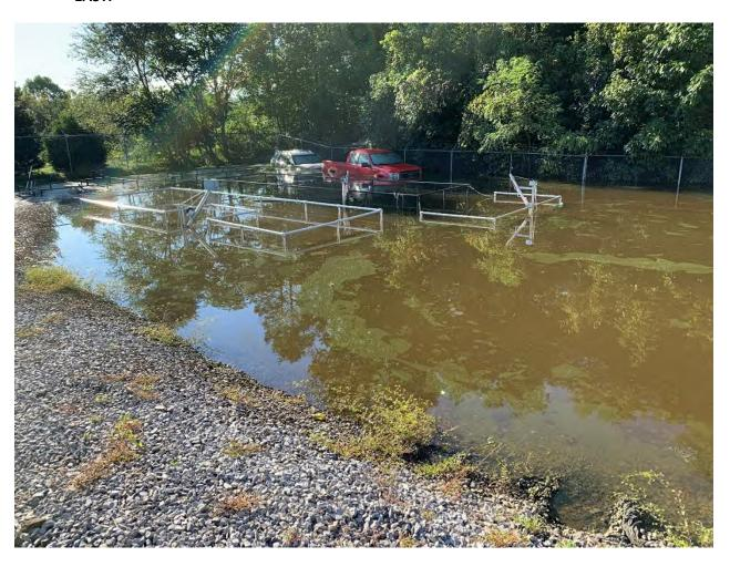
SUBMERGED WASTEWATER TREATMENT PLANT VIEW FROM SOUTHEAST SIDE OF PLANT LOOKING IN A SOUTH EASTERLY DIRECTION. GOLF COURSE CARTWAY BERM NEAR CULVERT SINK HOLE IN BACKGROUND (BEHIND WHITE CAR).
