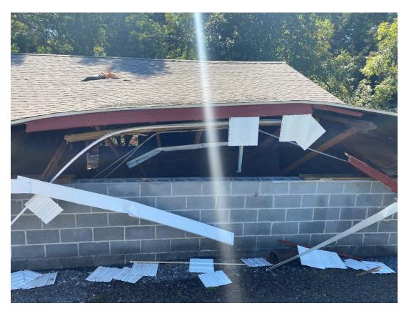
RAISED UP ROOF TRUSSES AND ROOF RESULTANT FROM TANK FLOATING IN THE CONTROL BUILDING.
