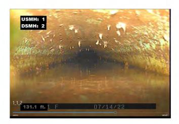
7-14-22 Discharge pipe belly between point of compliance sampling point and manhole on east side of WWTF plant site
