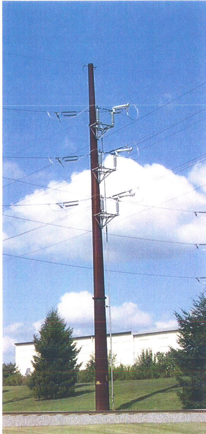
FIGURE 3 PROPOSED 138/69 kV SWITCH STRUCTURE APPROXIMATE HEIGHT – 65'
