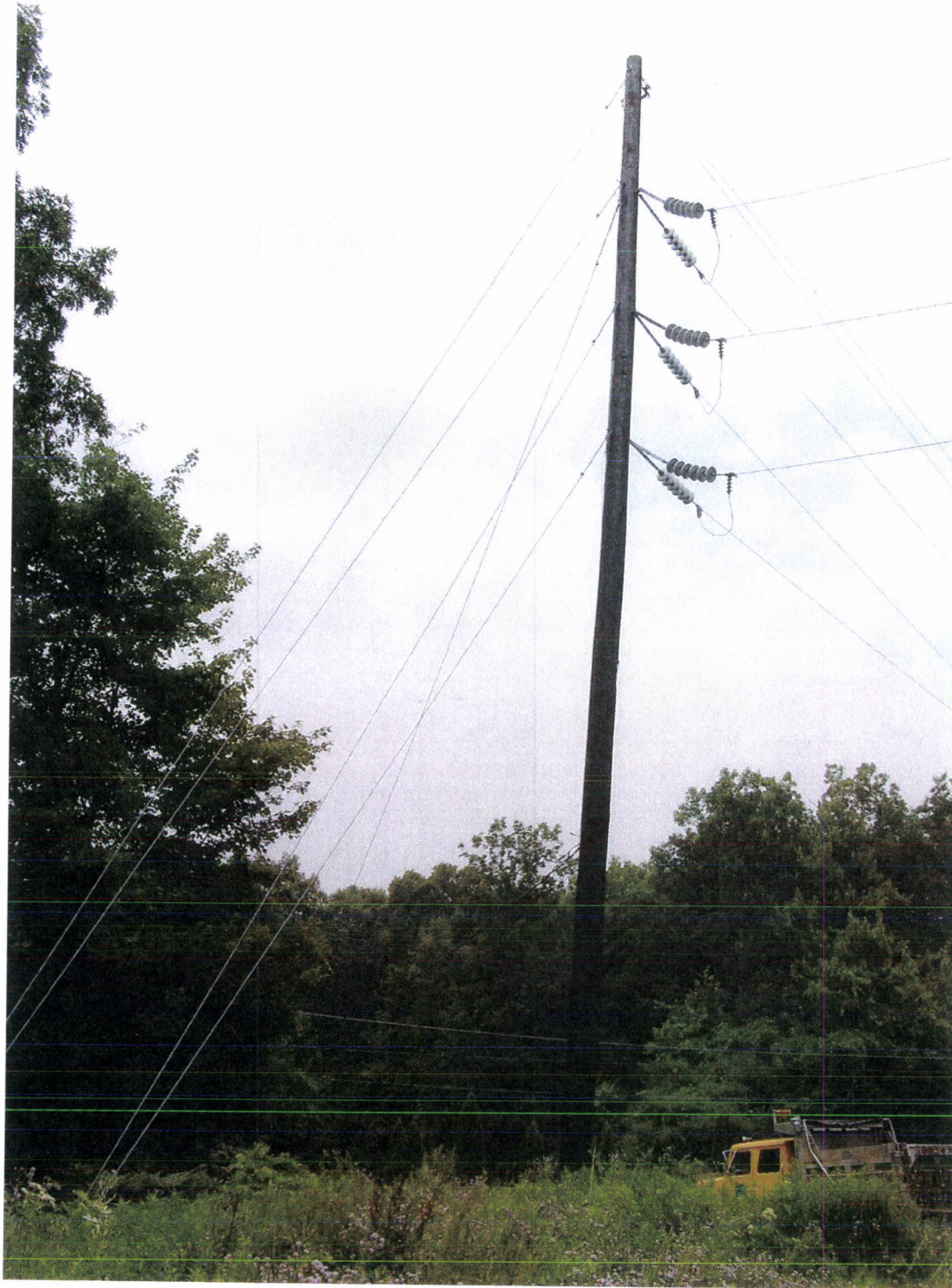
FIGURE 1 – PROPOSED 138/69 kV ANGLE STRUCTURE
