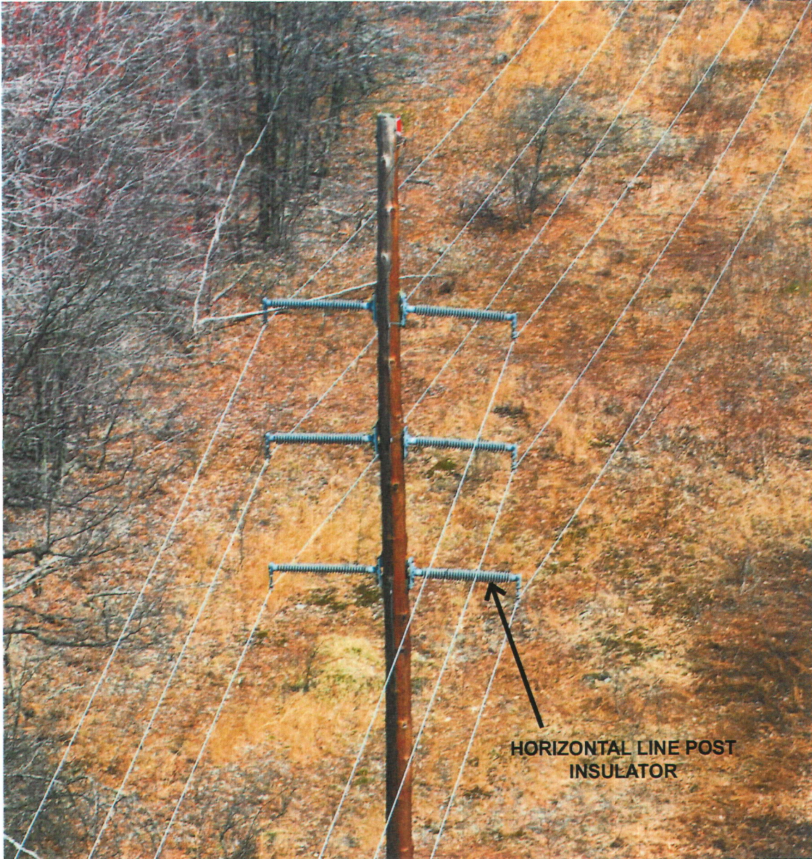
FIGURE 2 – TYPICAL HORIZONTAL LINE POST INSULATOR CONFIGURATION
