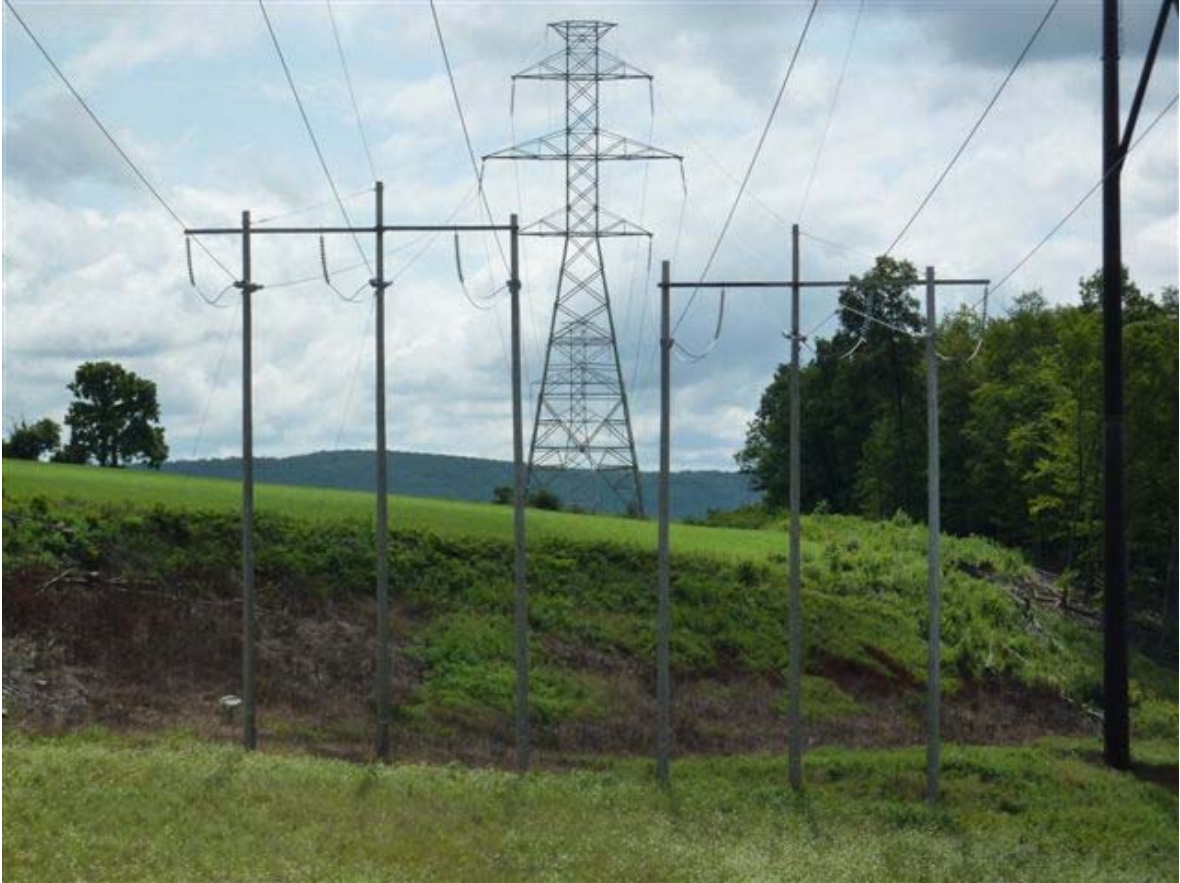
Figure 2: Structure to be Replaced
