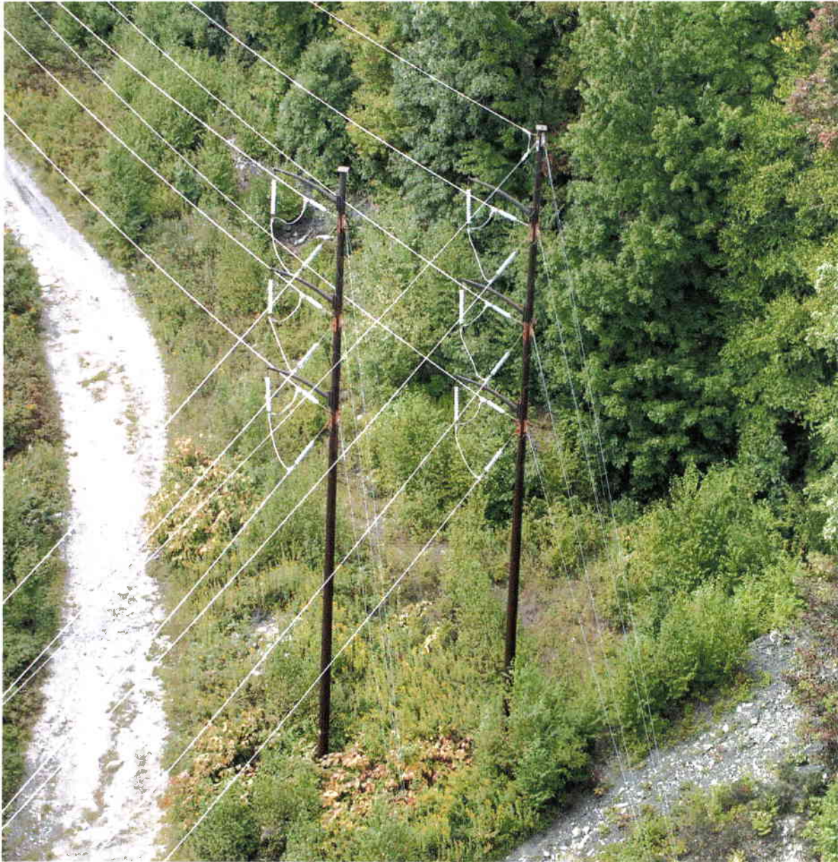
FIGURE 5-2: Double Circuit 138/69 kV Two-Pole Angle Structure
