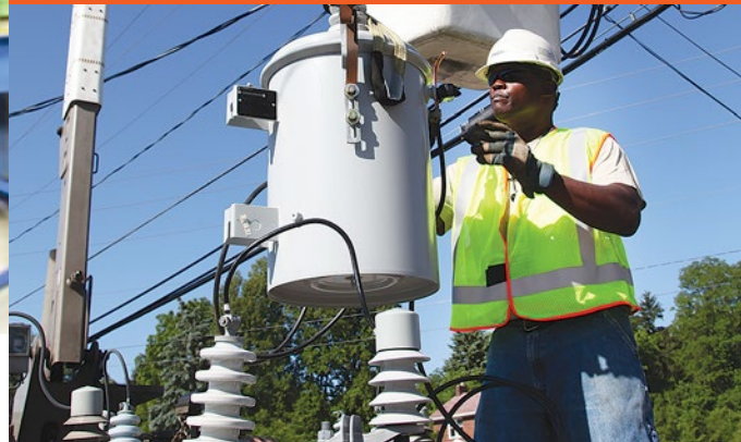
Left: New low-pressure turbine rotors were installed to improve the reliability and efficiency of Unit 1 of our Beaver Valley Power Station in Shippingport, Pa. Below: An Ohio Edison crew member replaces a three-phase power bank as part of a service upgrade for a commercial customer in Akron.
