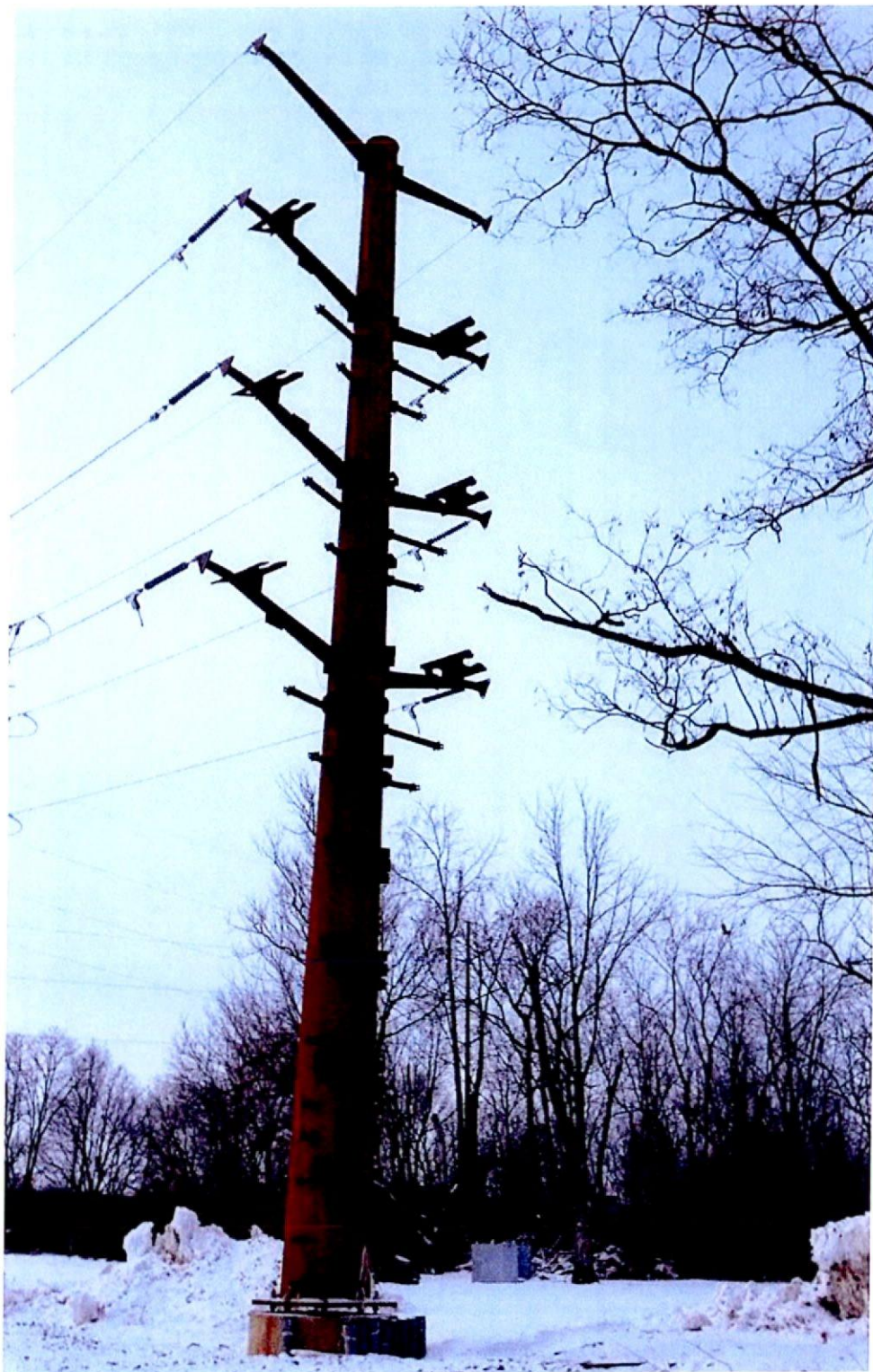
Attachment 2 – Typical 138 kV Terminal Pole
