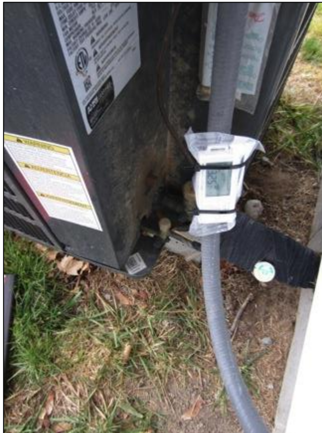
Figure 29. Motor Logger on Electric Conduit to Condenser
