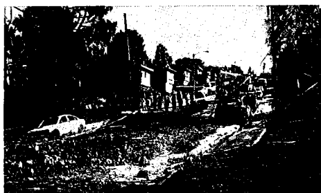
Aftermath of 2010 San Bruno, California Pipeline Explosion
