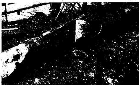
Remnants of a defunct gas pipeline
