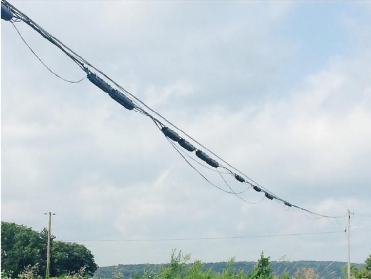
P. The picture at left from Monroe County shows a single cable that has become so damaged there are at least 10 splice boxes on a single span of a few hundred feet. Each splice box covers a portion of damaged or defective cable. Each of the numerous thin wires would have been installed in response to a separate customer complaint of either no dial tone or static on the line. Rather than replacing this
