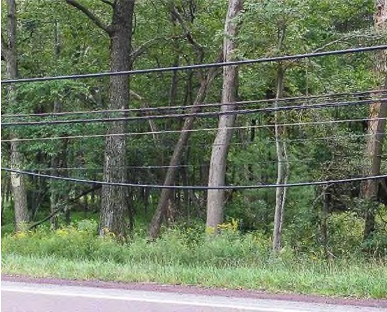
within easy reach of pedestrians, vehicles, and even children. Sagging cables also threaten the integrity of the conductor inside the cables, as strain is placed on the thin conductor which is improperly bearing the weight of the cable. The accompanying pictures show VZPA cables that are sagging perilously close to the ground. The picture at left from Luzerne County shows a VZPA cable that is only 3 or 4 feet above the ground. The picture below from Centre County shows a
