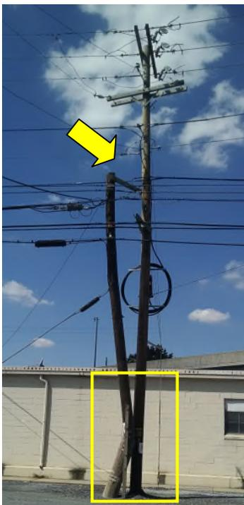
D. In the picture below left, an old double pole in Cumberland County has broken. The blow up shows that the base of the pole is being held together by a wooden post. The top of the old pole apparently is kept upright by a single brace to the newer pole (yellow arrow).
