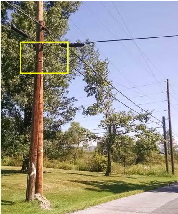
A. **Dangerous Double Poles.** The picture at left from Chester County shows two sets of double poles (one in the foreground and one in the background). The old pole in the foreground is clearly marked with an "X" indicating it is to be removed. This pole is so bent that it is tied to the new pole at the top to keep it from falling over (see blow-up below of area outlined in yellow). It appears that VZPA's facilities are the only ones still attached to the old poles.
