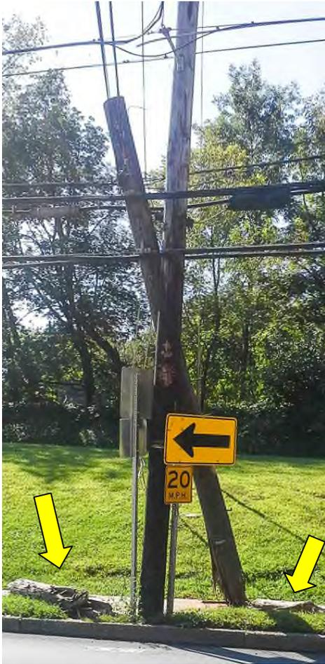
B. Double poles are not only unsightly, they also pose a hazard to line workers who must climb poles to work on the lines and other equipment. Having two poles in such close proximity reduces worker maneuverability (which can be essential when an animal or insect infestation or other hazard requires the worker to move quickly to avoid harm).
