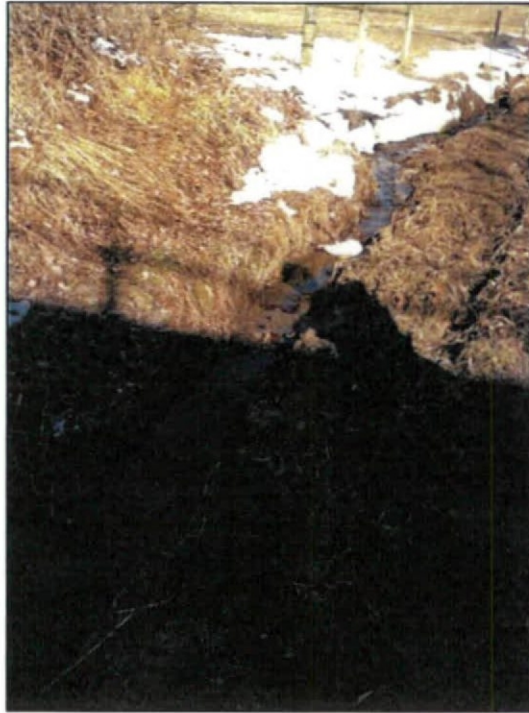
Photo 5 – Stream approaching underpass. Looking north from north side of underpass.
