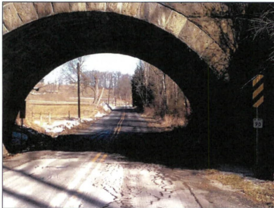
Photo 10 – View of rise in roadway approximately 560 feet north of underpass. Northbound approach to underpass looking north.
