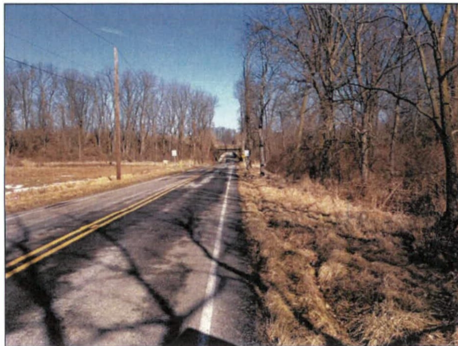
Photo 8 – Approach view of underpass from south looking north.
