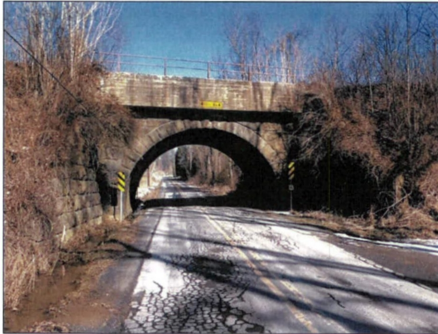
Photo 1 – Northbound approach to underpass looking north
