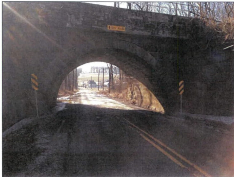
Photo 6 – Southbound approach to underpass looking south
