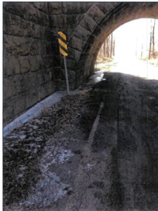
Photo 2 – East side of underpass from the north
