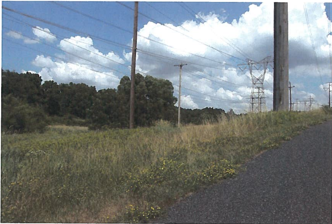
VIEW FACING EAST ALONG THE CORRIDOR, FROM THE WEST END, AS SEEN FROM THE WALKING TRAIL PATH THAT CROSSES OVER THE EASMENT AREA NEAR THE WEST END.
