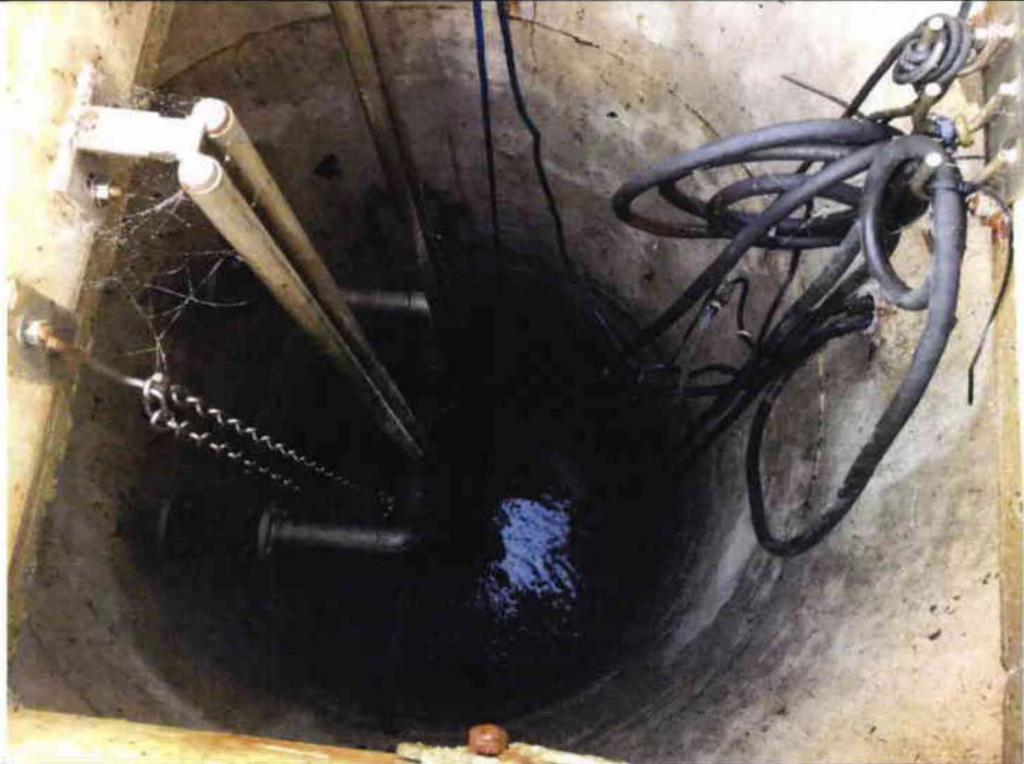
2 Pump Station #15 – Wet Well Interior.
