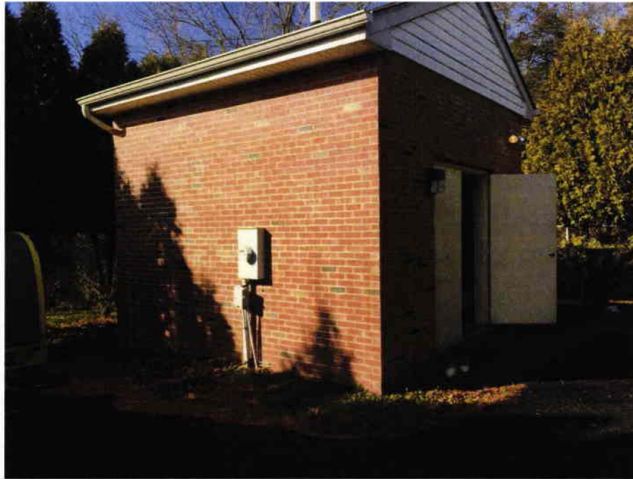
3 Pump Station #13 – Building Exterior.
