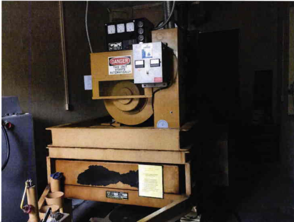
2 Pump Station #5 – Building Interior.
