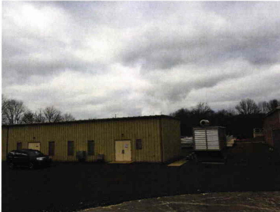
15 Blower Building and Generator
