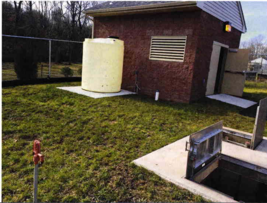
3 Pump Station #20 – Building Exterior.
