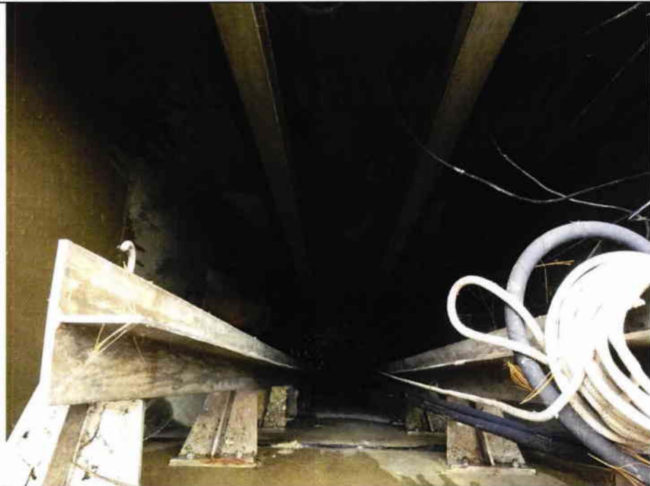
2 Pump Station #7 – Wet Well Interior.
