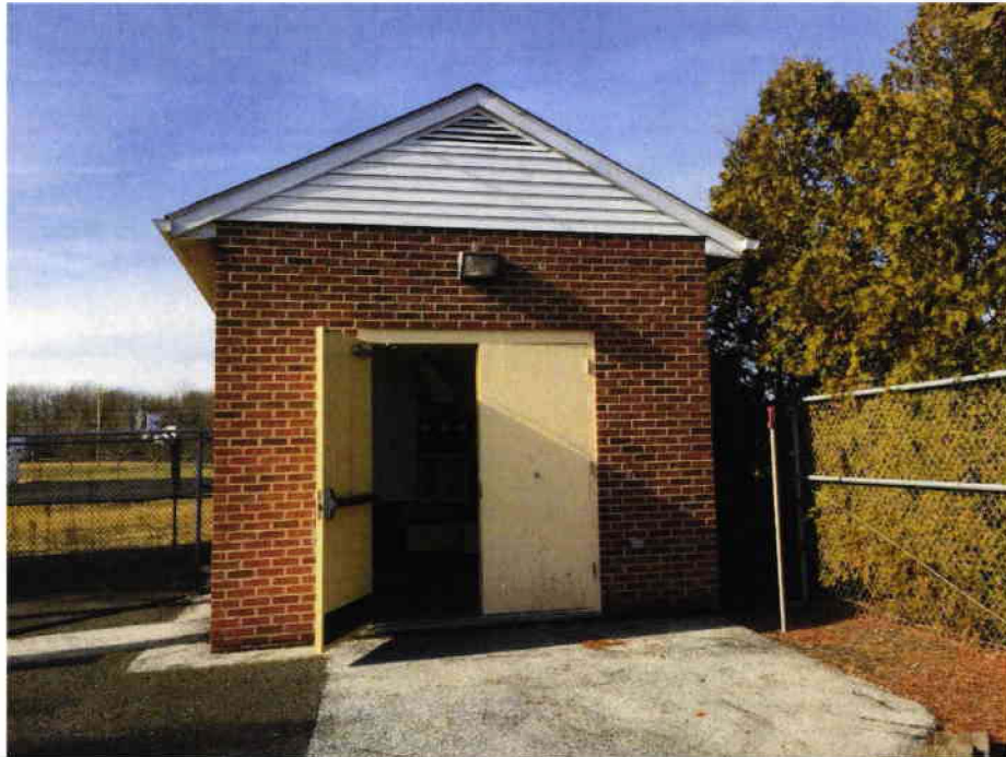
3 Pump Station #2 – Building Exterior.
