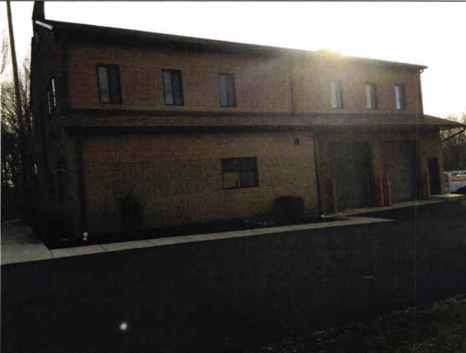
34 Office Building Exterior
