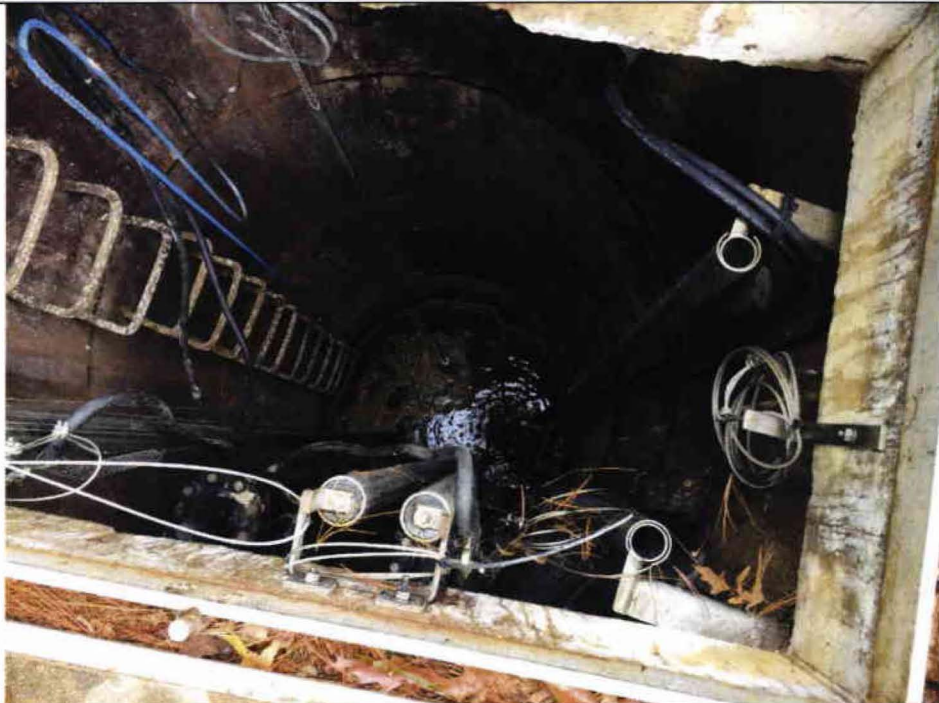
2 Pump Station #4 – Wet Well Interior.
