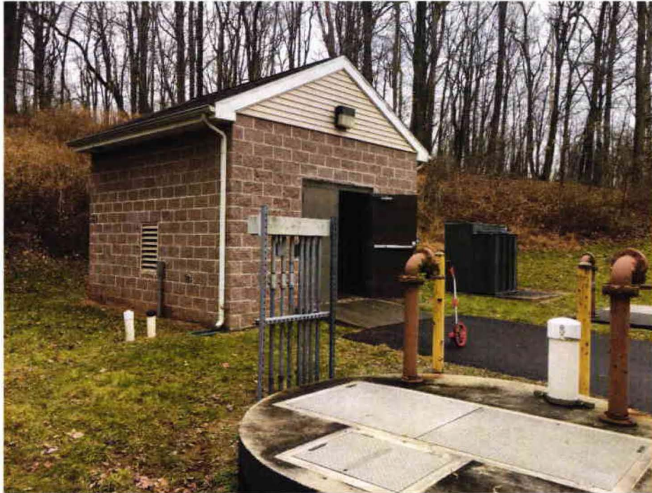
1 Pump Station #17 – Overall Site.
