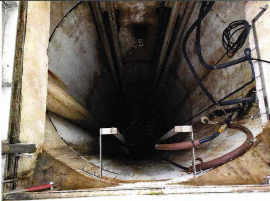
2 Pump Station #12 – Wet Well Interior.
