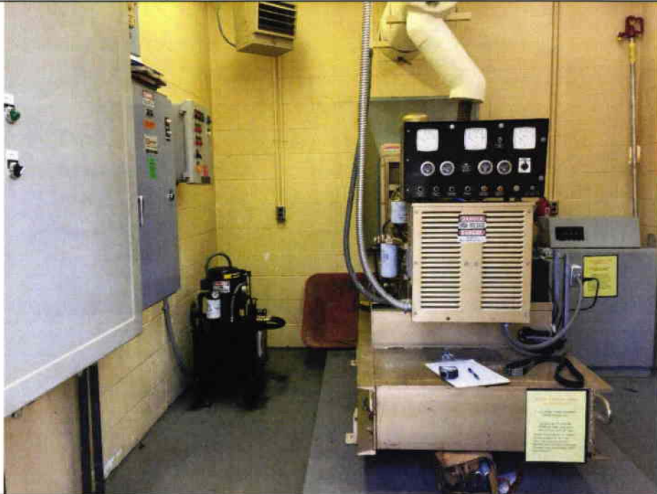
4 Pump Station #2 – Building Interior.
