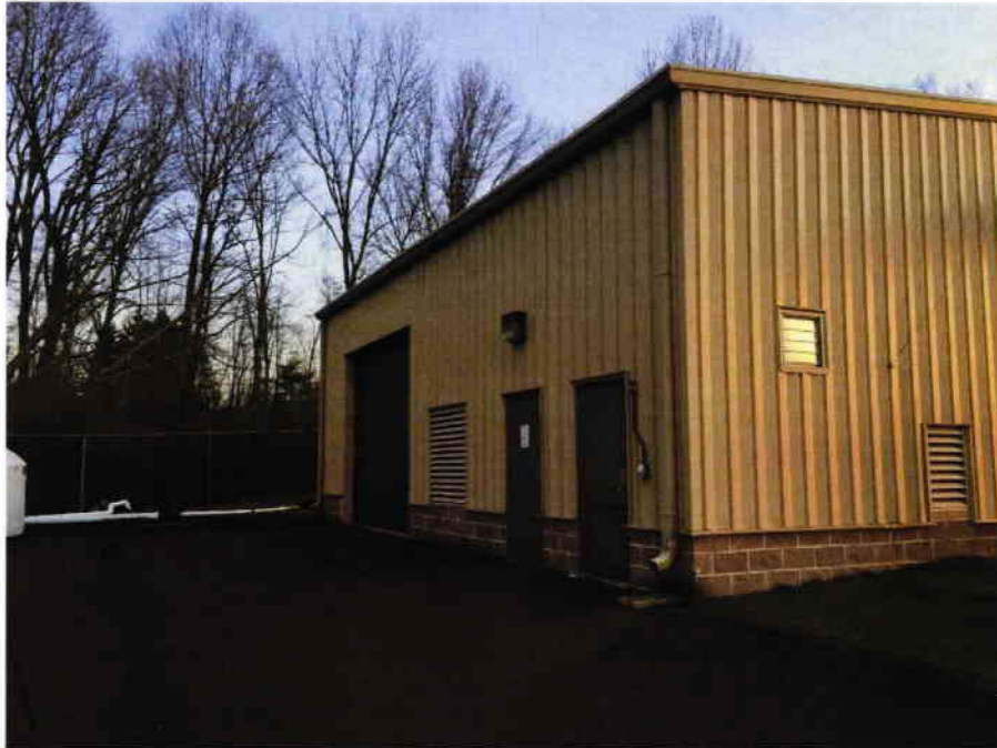
1 Possum Hollow WWTP- Building Entrance
