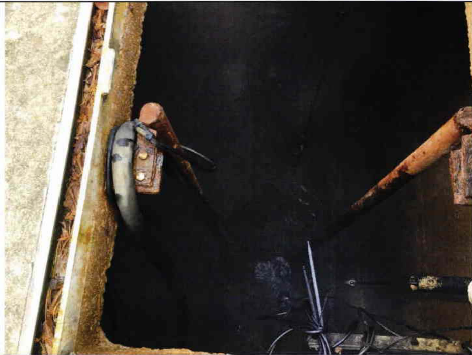
2 Pump Station #3 – Wet Well Interior.
