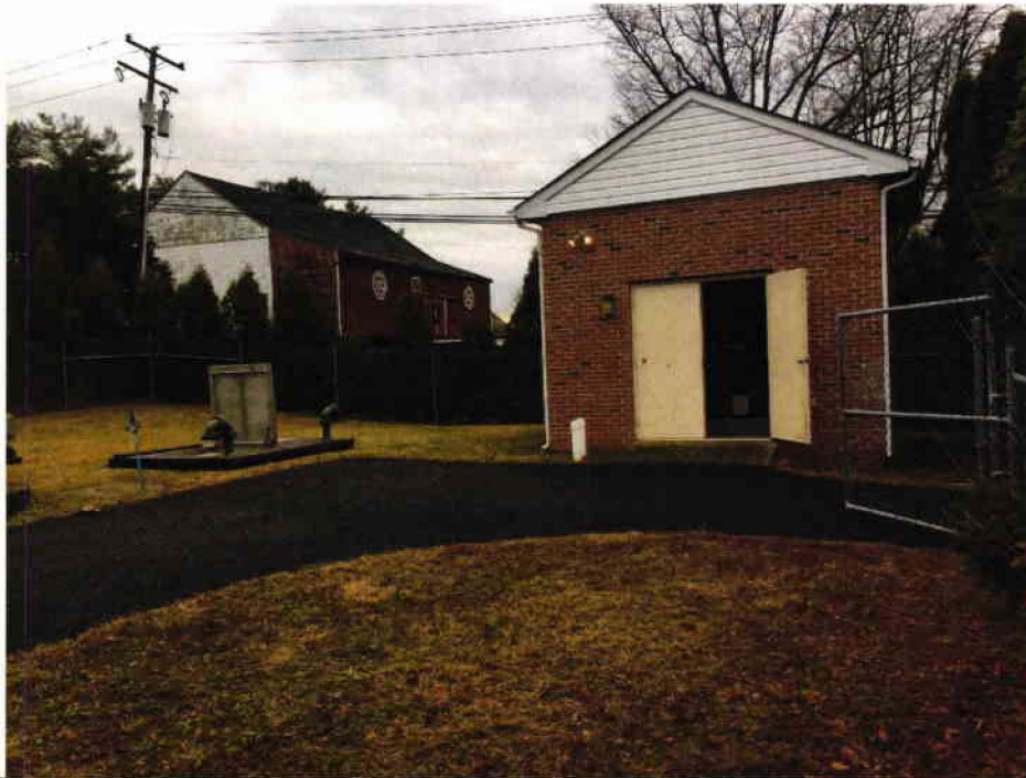
1 Pump Station #12 – Overall Site.
