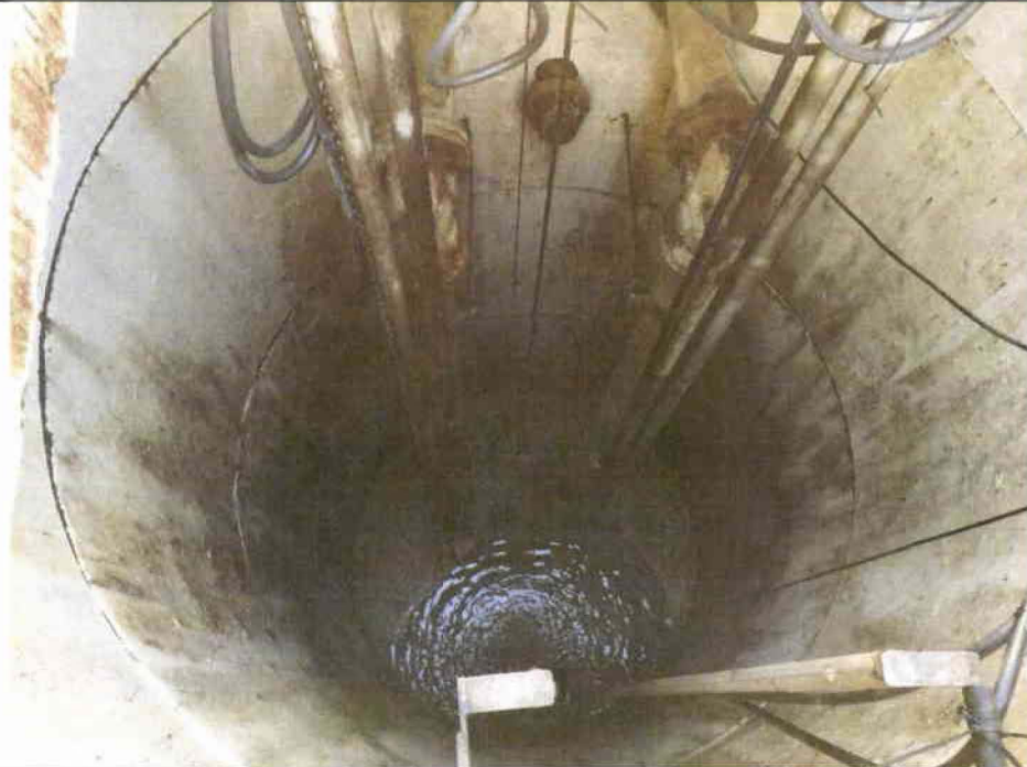
2 Pump Station #10 – Wet Well Interior.
