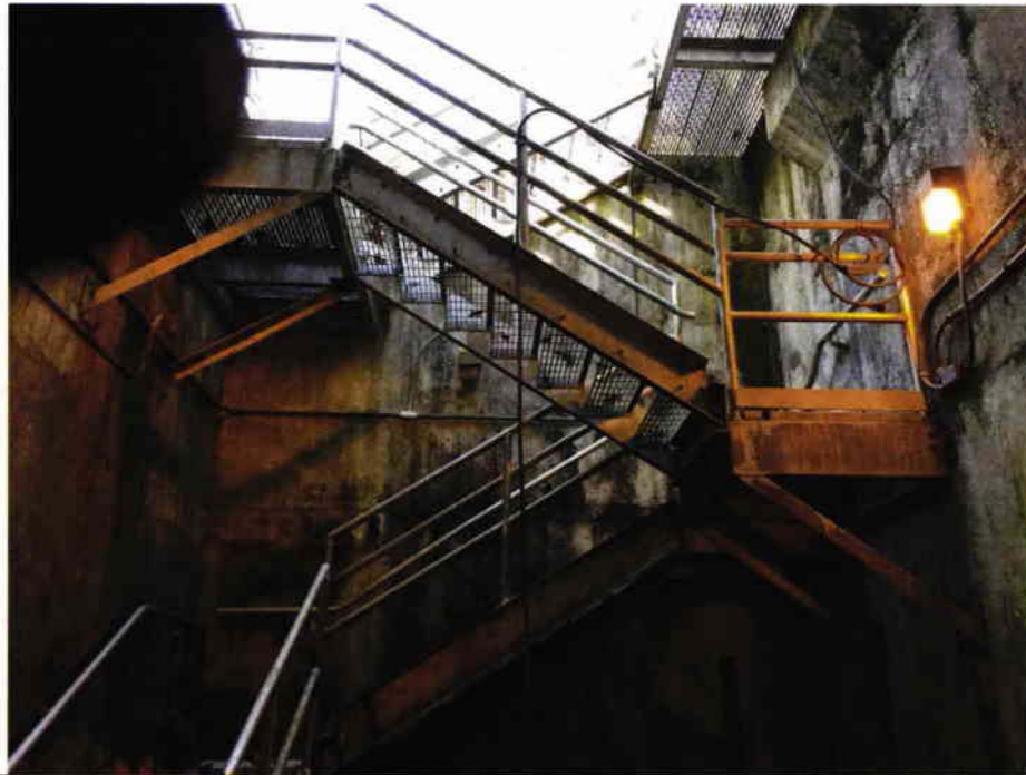
4 Pump Station #5 – Stairwell.
