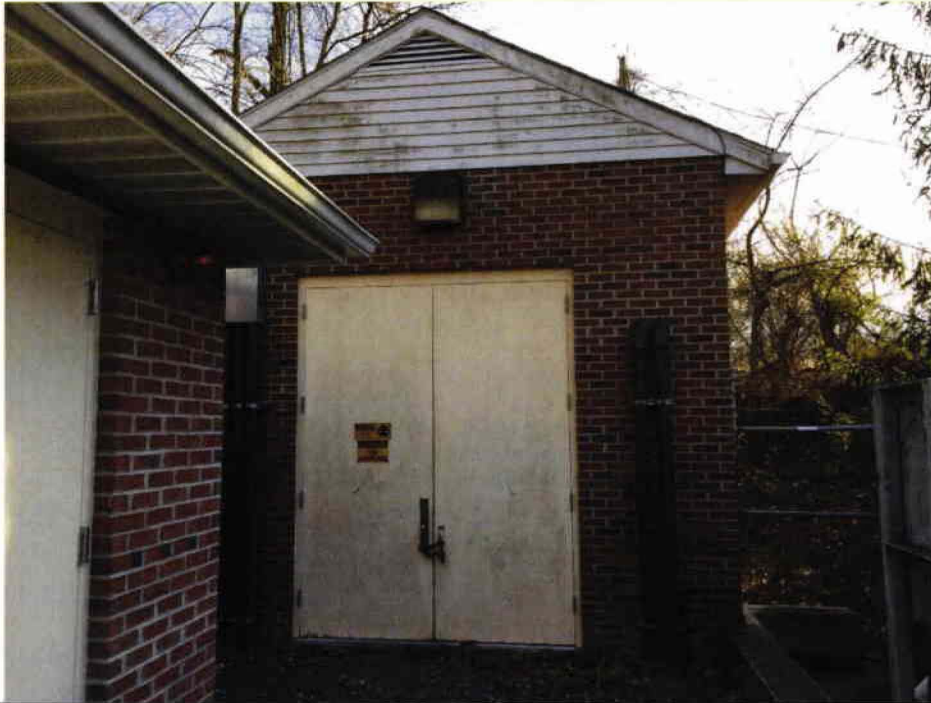
1 Pump Station #5 – Building Exterior.
