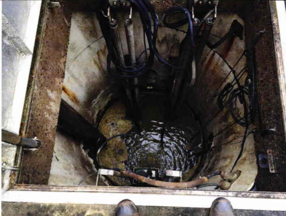
2 Pump Station #14 – Wet Well Interior.
