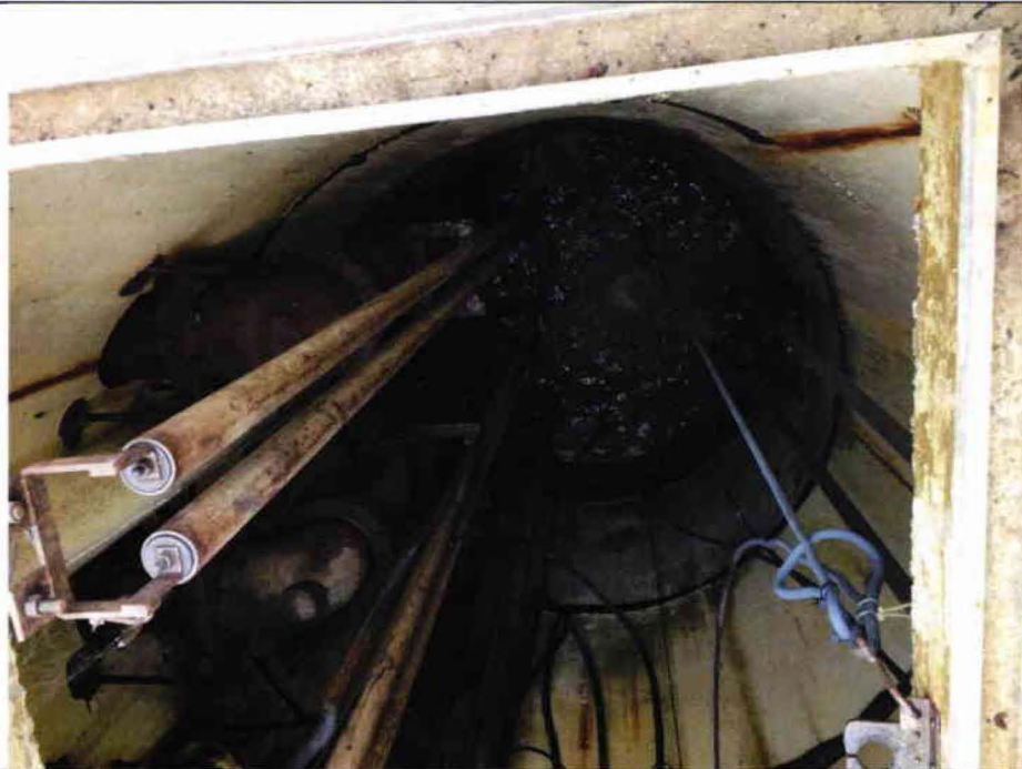
2 Pump Station #17 – Wet Well Interior.
