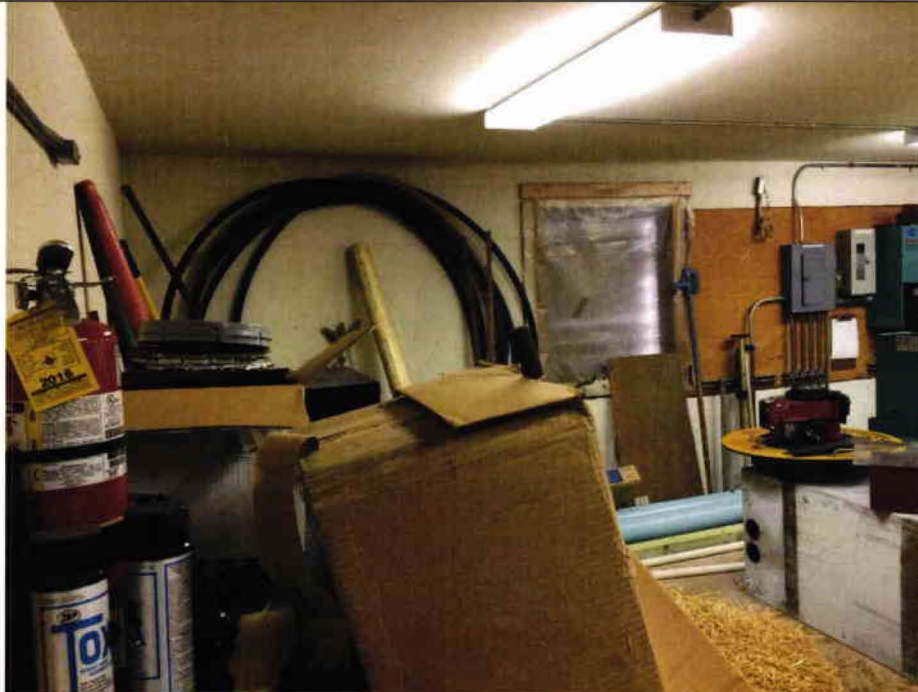
4 Pump Station #8 – Building Interior.
