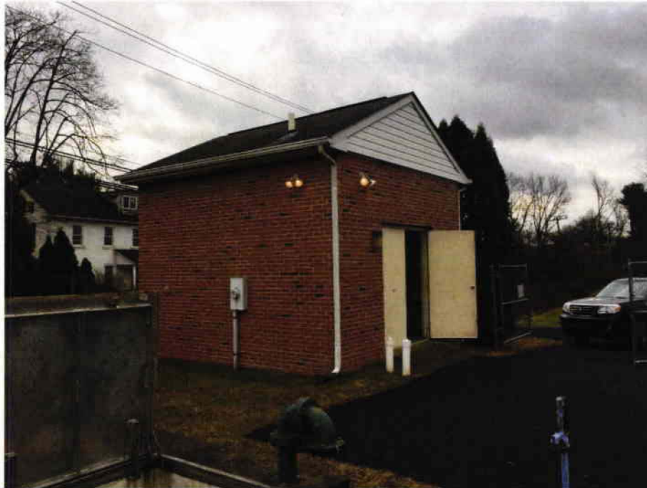
3 Pump Station #12 – Building Exterior
