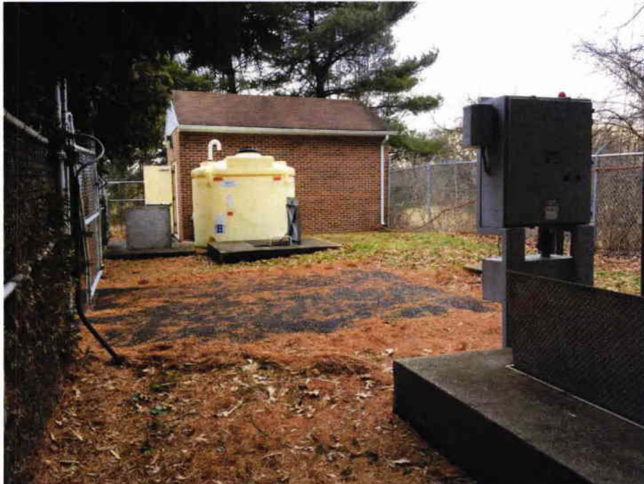
1 Pump Station #7 – Overall Site.
