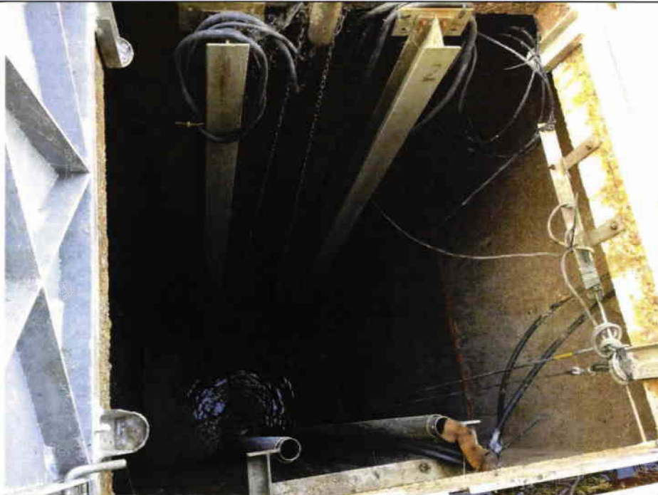
2 Pump Station #2 – Wet Well Interior.
