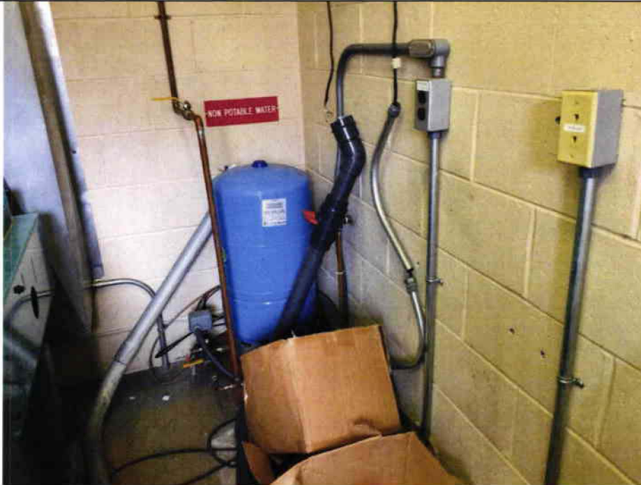
4 Pump Station #9 –Building Interior.
