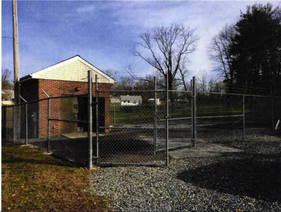
1 Pump Station #9 – Overall Site.
