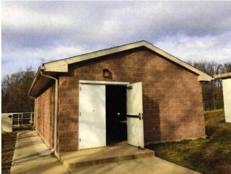
29 UV System Pump Building
