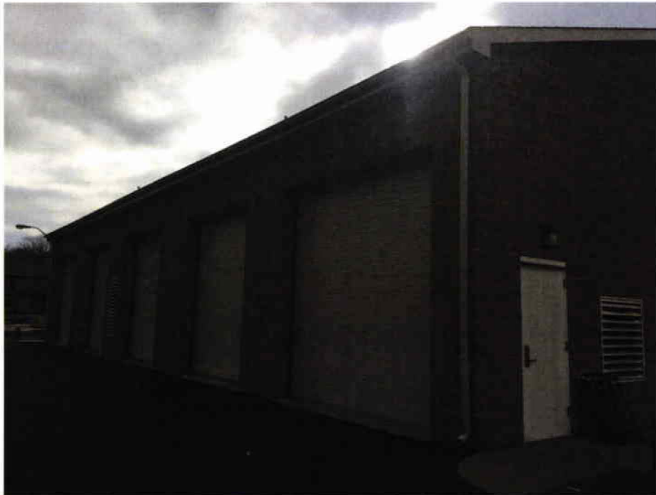
21 Maintenance Building Exterior
