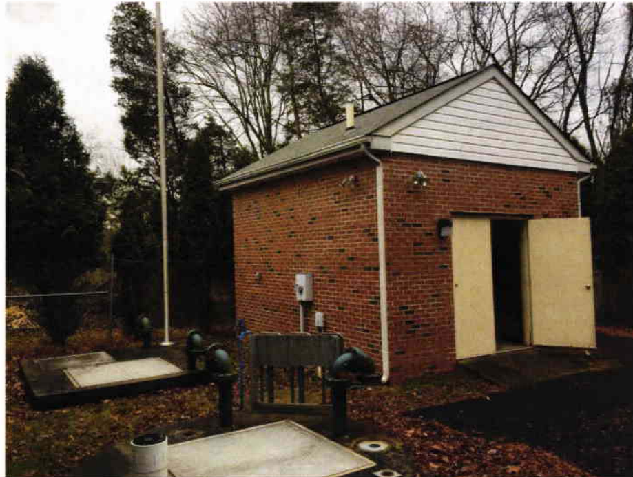
3 Pump Station #14 – Building Exterior.
