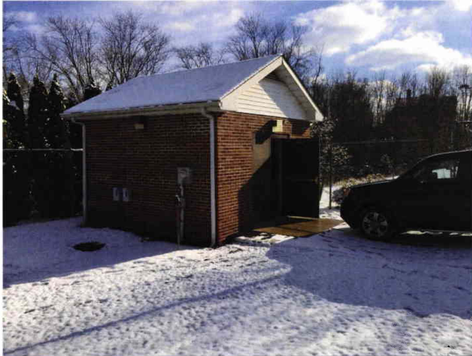
3 Pump Station #15 – Building Exterior.
