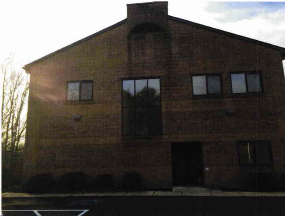
33 Office Building Exterior (Entrance Side)
