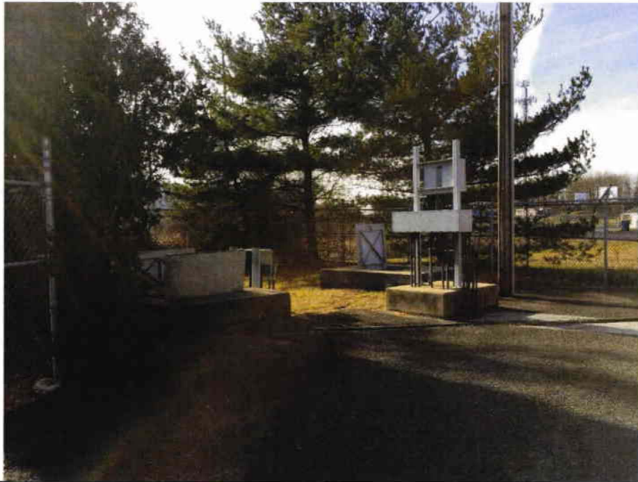
1 Pump Station #2 – Overall Site.
