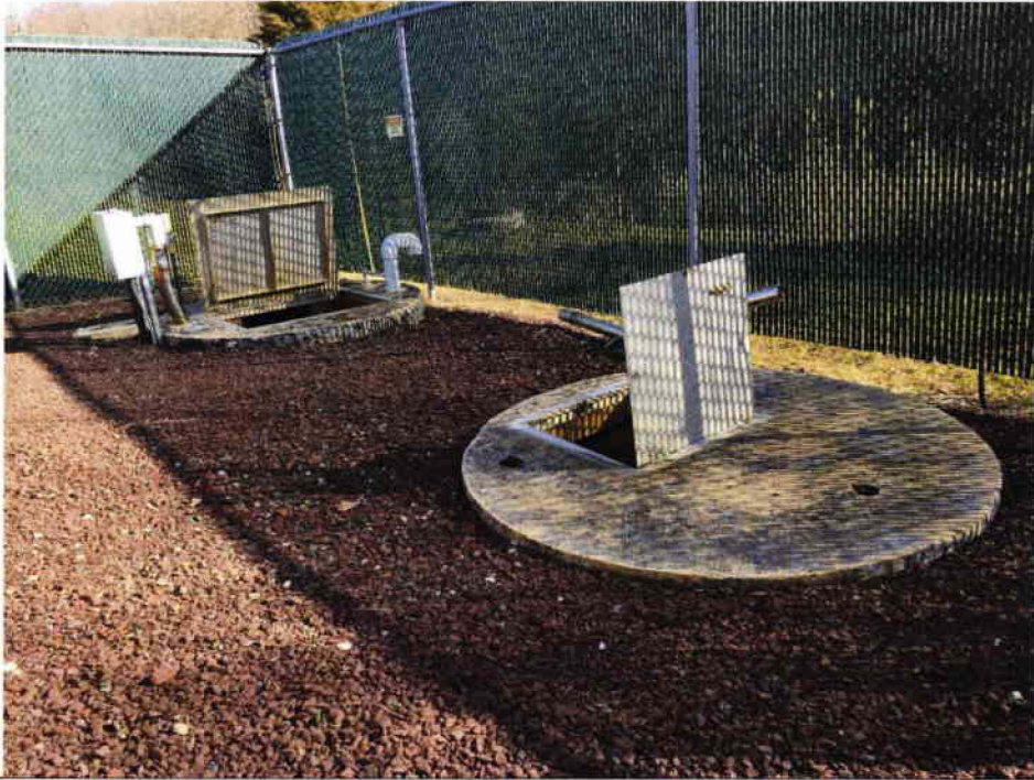
1 Pump Station #1 – Wet Well and valve chamber
