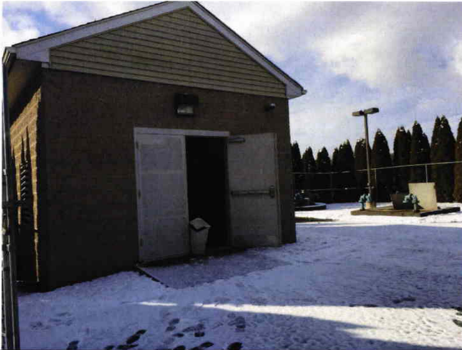
1 Pump Station #3 – Overall Site.
