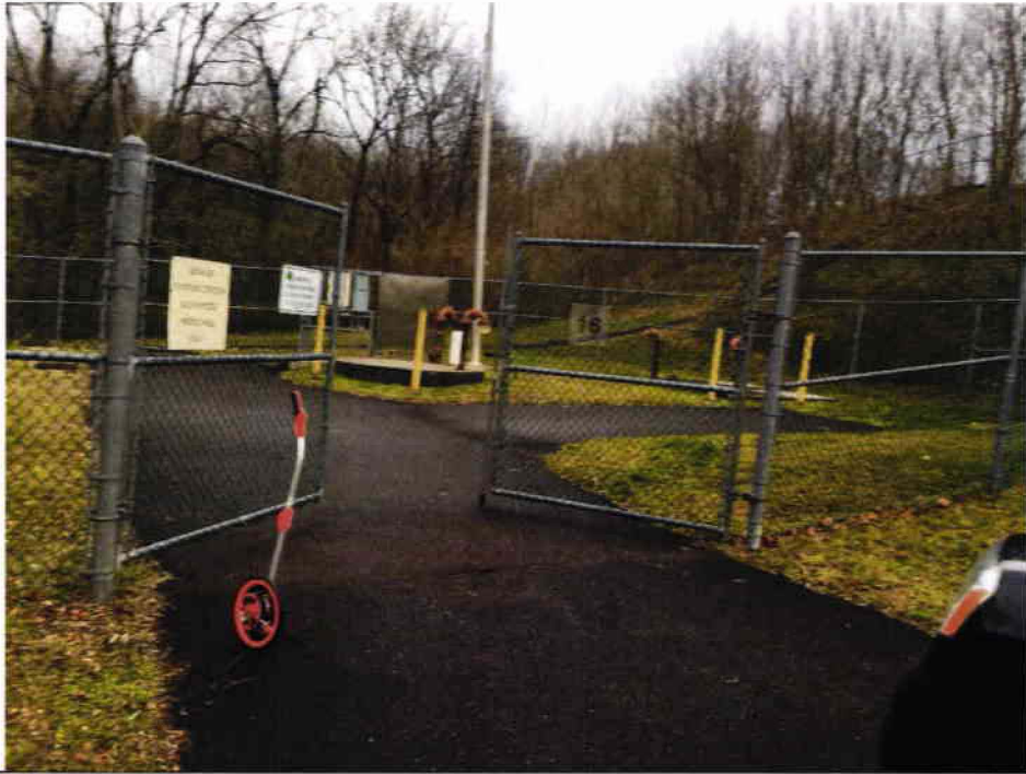
1 Pump Station #16 – Overall Site.
