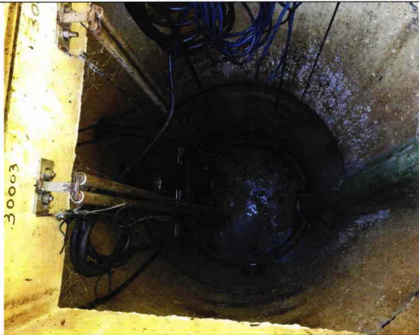
2 Pump Station #13 – Wet Well Interior.
