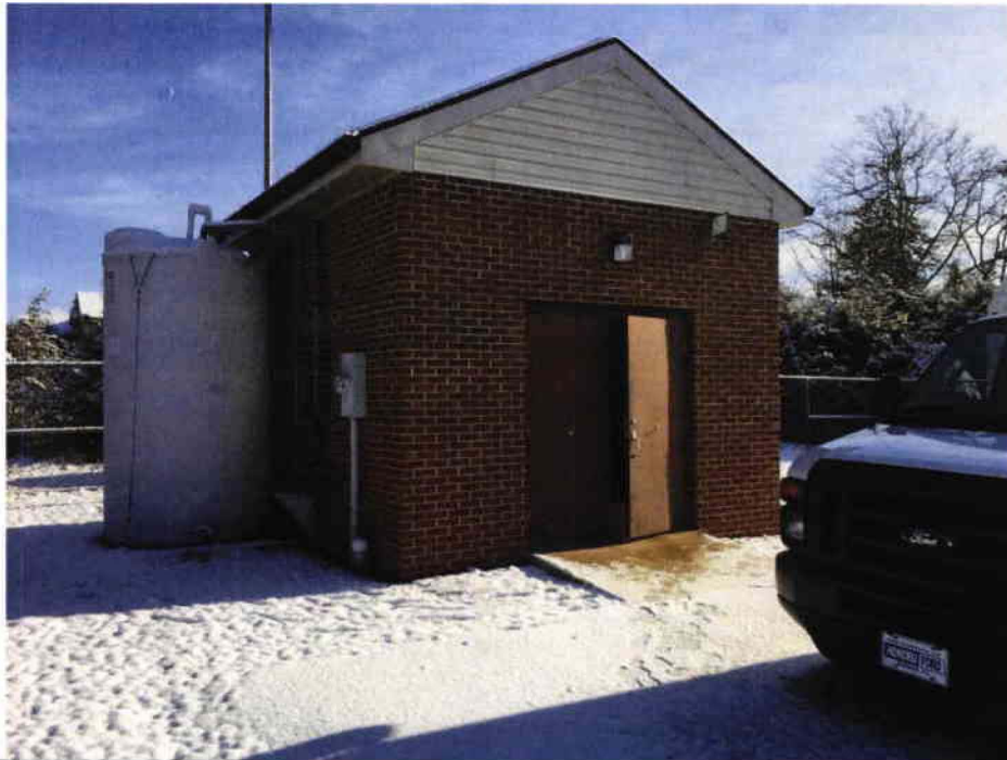
3 Pump Station #10 – Building Exterior.
