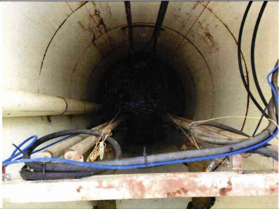
2 Pump Station #20 – Wet Well Interior.
