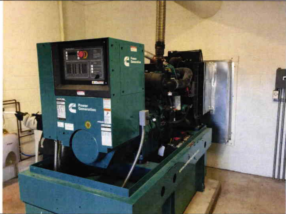
4 Pump Station #20 – Building Interior.
