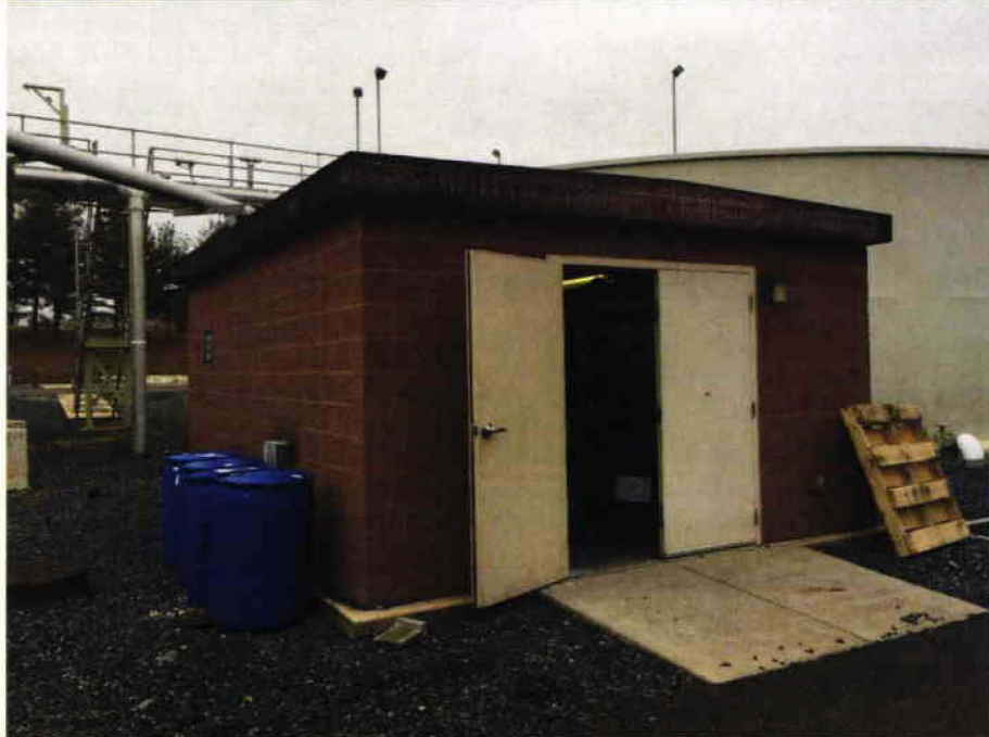
10 Sludge Thickener Building
