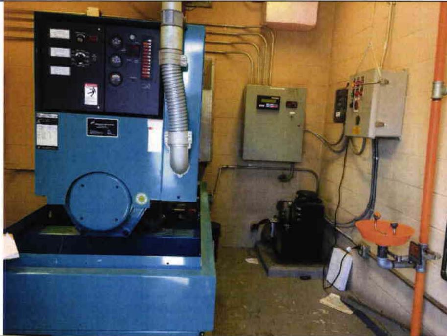
4 Pump Station #10 – Building Interior.
