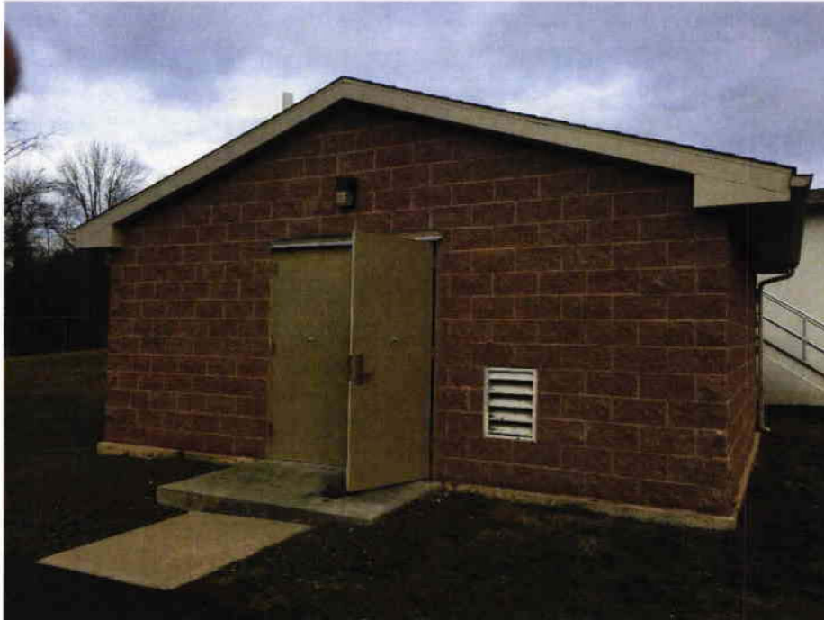
27 | WAS Sludge Pumping Building
