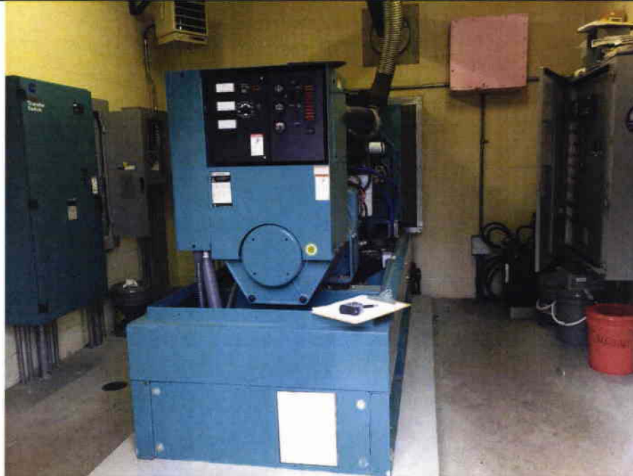
4 Pump Station #14 – Building Interior.
