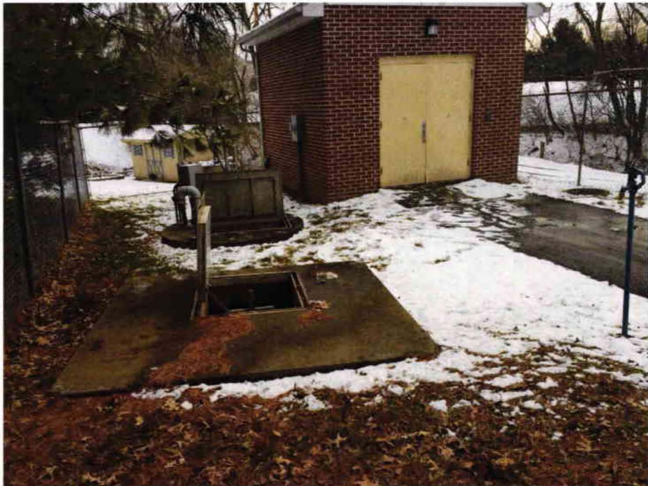
1 Pump Station #4 – Overall Site.
