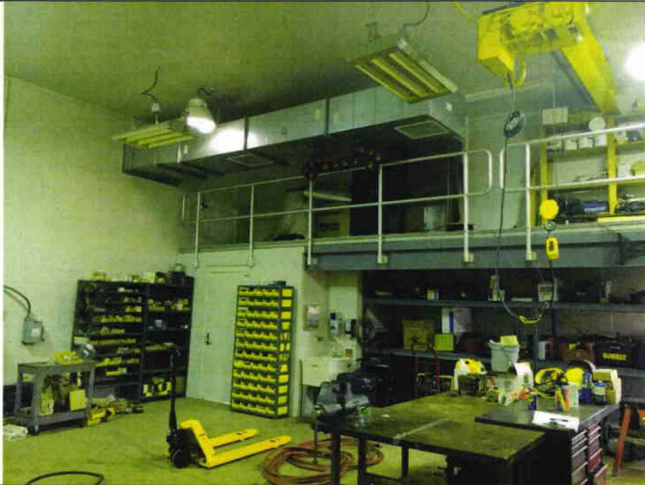
20 Maintenance Building Work Shop Area
