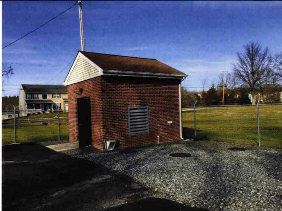
2 Pump Station #9 – Building Exterior.
