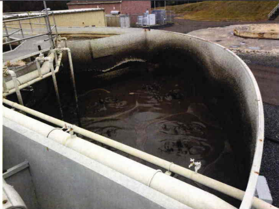
8 Aeration Chamber Sludge Holding Chamber
