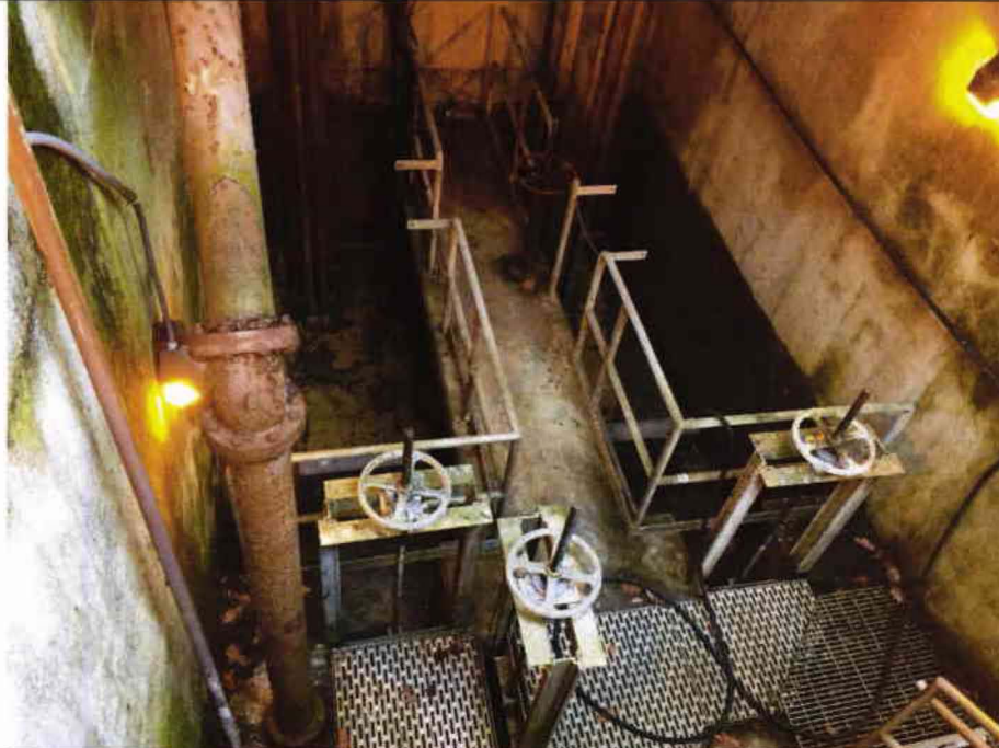
3 Pump Station #5 – Wet Well Interior.
