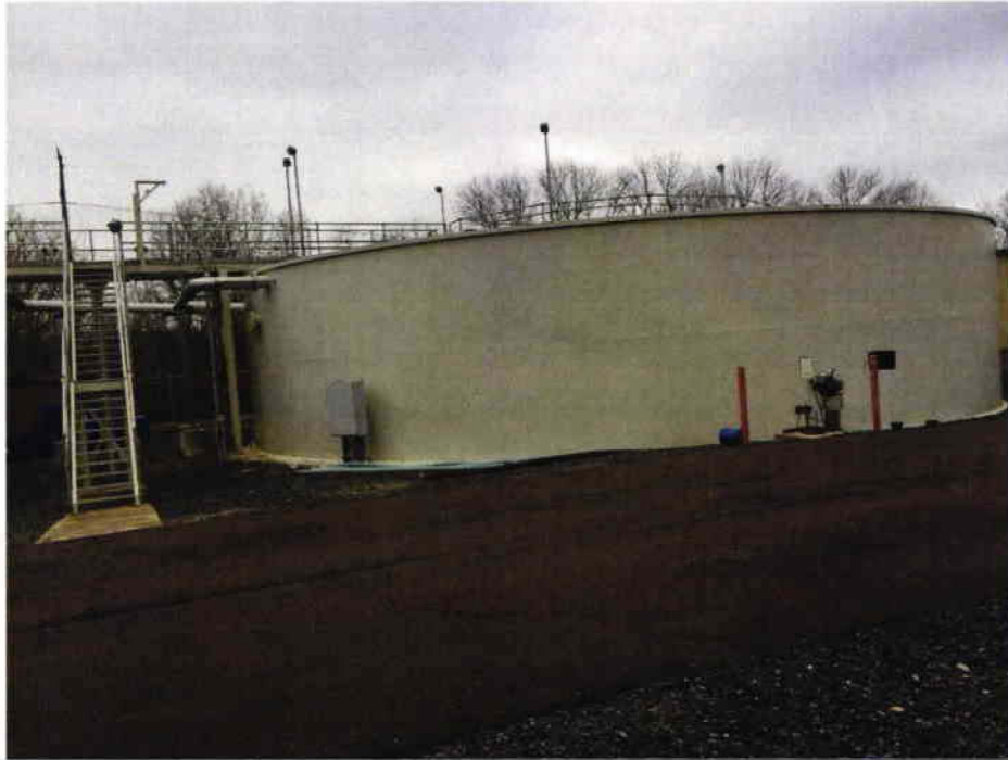
9 Sludge Digester
