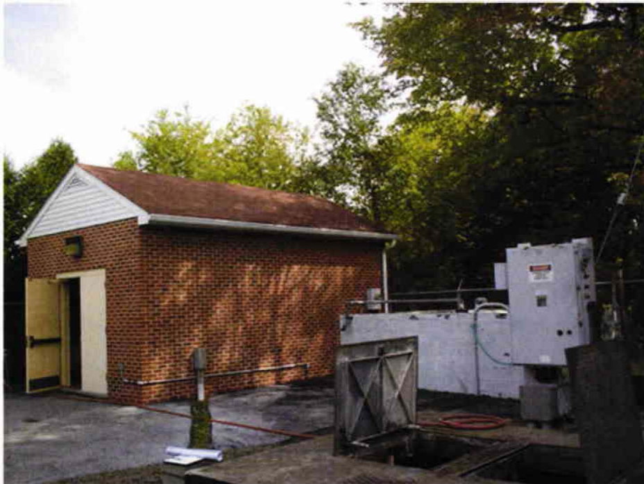
1 Pump Station #3 – Overall Site.
