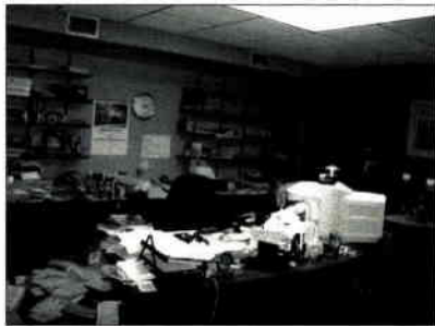
TICO BUILDING OFFICE DEMOLITION PHOTOGRAPH TB3-G REFERENCE PLAN TB2-A
