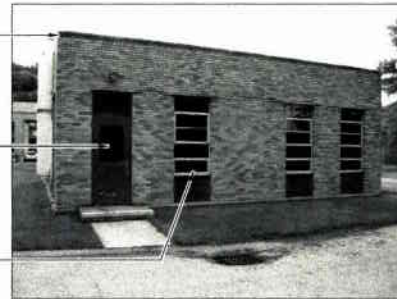
W.W.T.P. PUMP STATION SOUTH ELEVATION DEMOLITION PHOTOGRAPH PS5-B REFERENCE ELEVATION PS1-C
