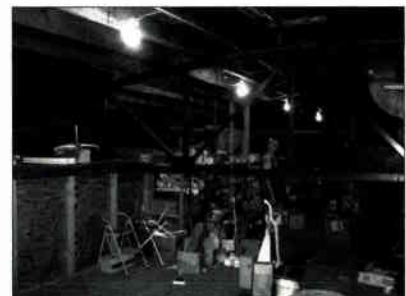
TICO BUILDING UPPER STORAGE ROOM DEMOLITION PHOTOGRAPH TB5-E REFERENCE PLAN TB5-A
