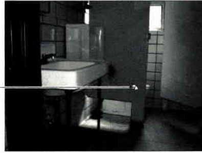
W.W.T.P. PUMP STATION FLOOR EL. 744.00 DEMOLITION PHOTOGRAPH PS6-B REFERENCE PLAN PS2-A
