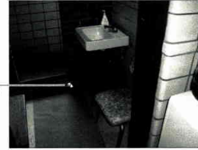
W.W.T.P. PUMP STATION FLOOR EL. 744.00 DEMOLITION PHOTOGRAPH PS6-C REFERENCE PLAN PS2-A
