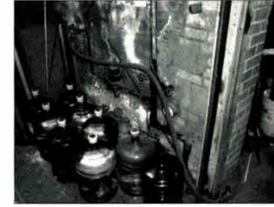
TICO BUILDING WATER MAIN DEMOLITION PHOTOGRAPH TB4-C REFERENCE PLAN TB2-A
