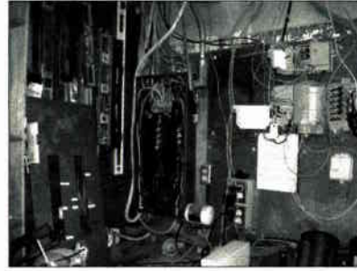
TICO BUILDING ELECTRICAL PANEL DEMOLITION PHOTOGRAPH TB4-B REFERENCE PLAN TB2-A
