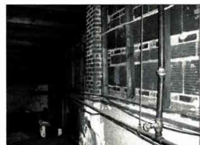
TICO BUILDING UPPER STORAGE ROOM DEMOLITION PHOTOGRAPH TB5-G REFERENCE PLAN TB5-A
