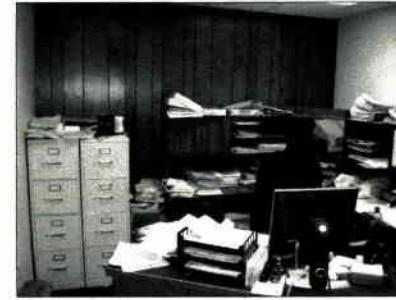
TICO BUILDING OFFICE DEMOLITION PHOTOGRAPH TB3-C REFERENCE PLAN TB2-A
