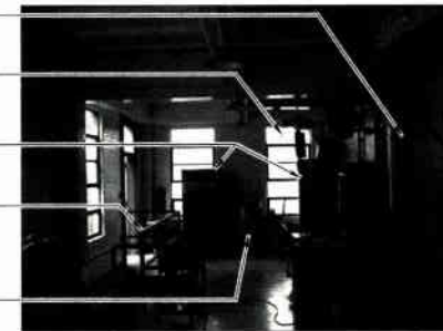
W.W.T.P. PUMP STATION FLOOR EL. 744.00 DEMOLITION PHOTOGRAPH PS5-F REFERENCE PLAN PS2-A
