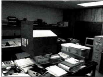
TICO BUILDING OFFICE DEMOLITION PHOTOGRAPH TB3-D REFERENCE PLAN TB2-A
