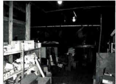
TICO BUILDING UPPER STORAGE ROOM DEMOLITION PHOTOGRAPH TB5-A REFERENCE PLAN TB5-A
