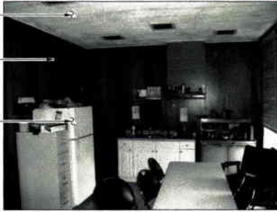
W.W.T.P. PUMP STATION FLOOR EL. 744.00 DEMOLITION PHOTOGRAPH PS6-A REFERENCE PLAN PS2-A
