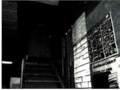
TICO BUILDING STORAGE STAIRS DEMOLITION PHOTOGRAPH TB4-A REFERENCE PLAN TB2-A
