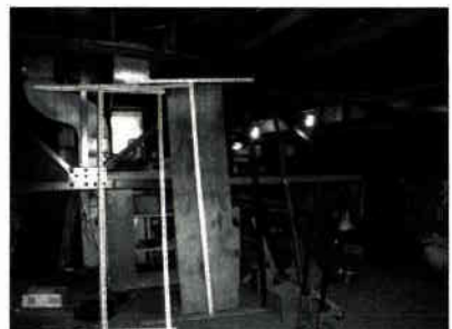
TICO BUILDING UPPER STORAGE ROOM DEMOLITION PHOTOGRAPH TB5-D REFERENCE PLAN TB5-A
