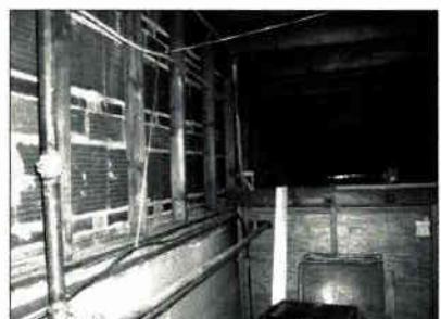
TICO BUILDING UPPER STORAGE ROOM DEMOLITION PHOTOGRAPH TB5-F REFERENCE PLAN TB5-A
