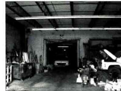
TICO BUILDING STORAGE ROOM DEMOLITION PHOTOGRAPH TB3-J REFERENCE PLAN TB2-A
