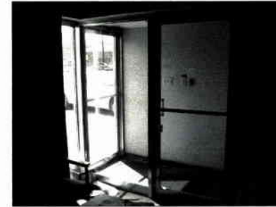
TICO BUILDING LOBBY DEMOLITION PHOTOGRAPH TB3-F REFERENCE PLAN TB2-A
