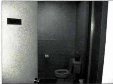
TICO BUILDING WOMENS ROOM DEMOLITION PHOTOGRAPH TB4-G REFERENCE PLAN TB2-A
