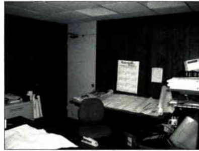
TICO BUILDING OFFICE DEMOLITION PHOTOGRAPH TB3-B REFERENCE PLAN TB2-A
