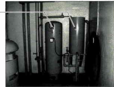
W.W.T.P. PUMP STATION (DRY WELL) FLOOR EL. 718.59 DEMOLITION PHOTOGRAPH PS6-J REFERENCE PLAN PS3-A
