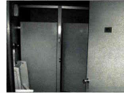
TICO BUILDING MENS ROOM DEMOLITION PHOTOGRAPH TB4-F REFERENCE PLAN TB2-A
