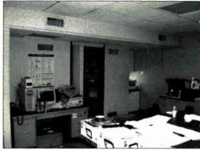
TICO BUILDING KITCHEN DEMOLITION PHOTOGRAPH TB3-A REFERENCE PLAN TB2-A
