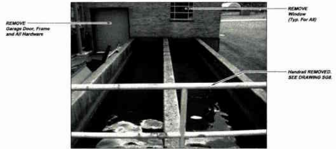
SCREEN/ GRIT BUILDING EXTERIOR DEMOLITION PHOTOGRAPH AE5-E REFERENCE ELEVATION AE4-C
