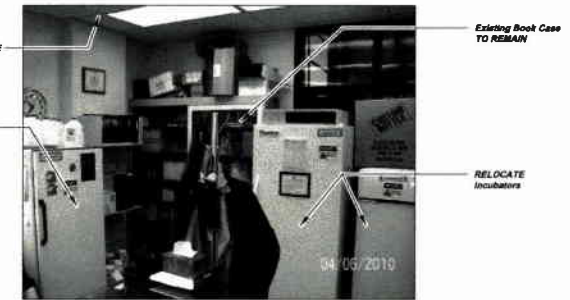
INTERIOR LABORATORY (LOOKING WEST) DEMOLITION PHOTOGRAPH LA3-F REFERENCE PLAN LA1-A
