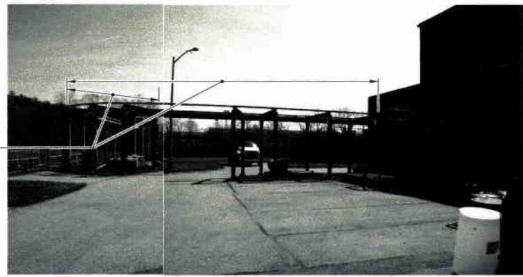
DEMOLITION PHOTOGRAPH C11-D REFERENCE PLAN C11-A
