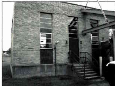
SCREEN/GRIT BUILDING EXTERIOR DEMOLITION PHOTOGRAPH SG3-A
