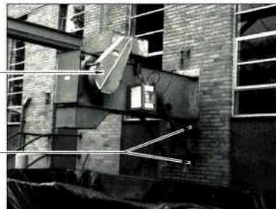
SCREEN/GRIT BUILDING EXTERIOR DEMOLITION PHOTOGRAPH SG3-B
