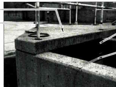
SCREEN/GRIT BUILDING EXTERIOR DEMOLITION PHOTOGRAPH SG3-E
