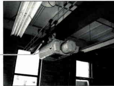
CHLORINE ROOM DEMOLITION PHOTOGRAPH C13-J
