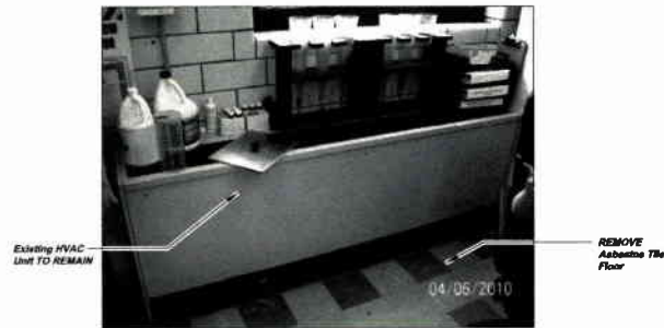
INTERIOR LABORATORY (LOOKING SOUTH) DEMOLITION PHOTOGRAPH LA3-D REFERENCE PLAN LA1-A
