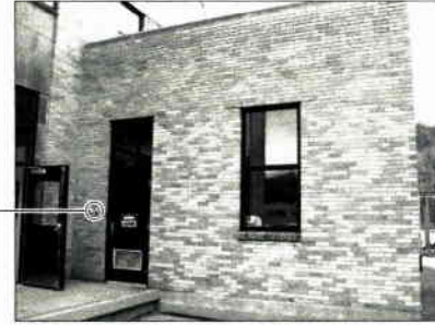
CHLORINE ROOM DEMOLITION PHOTOGRAPH C13-F
