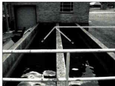
SCREEN/GRIT BUILDING EXTERIOR DEMOLITION PHOTOGRAPH SG3-D
