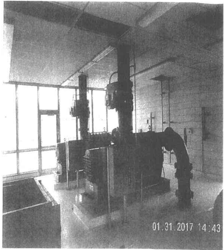
Blower Building / Secondary Pump Station
