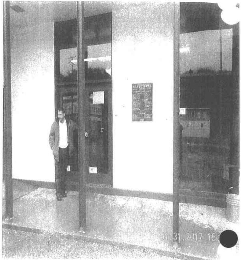
Dravosbury Treatment Plant 0.5 mgd
