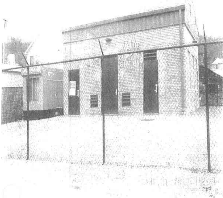
28 th Avenue Pump Station
