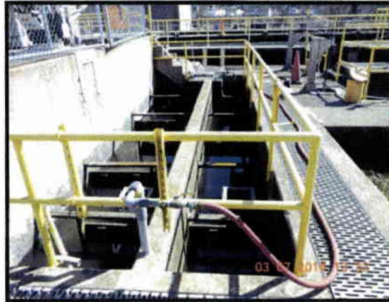
Chlorine Contact Tank Photograph 6.4
