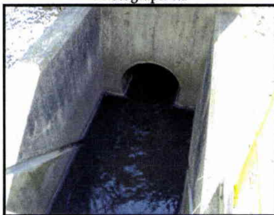
Influent Channel Photograph 6.1
