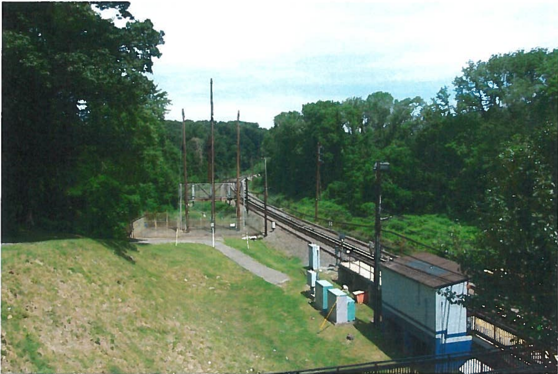
VIEW LOOKING NORTH FROM U. S. ROUTE 1, AT THE WEST OVERBROOK STATION, SOUTH END OF THE LINE.
