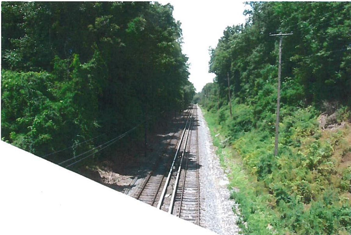
VIEW LOOKING NORTH AT THE GULPH ROAD OVERPASS.
