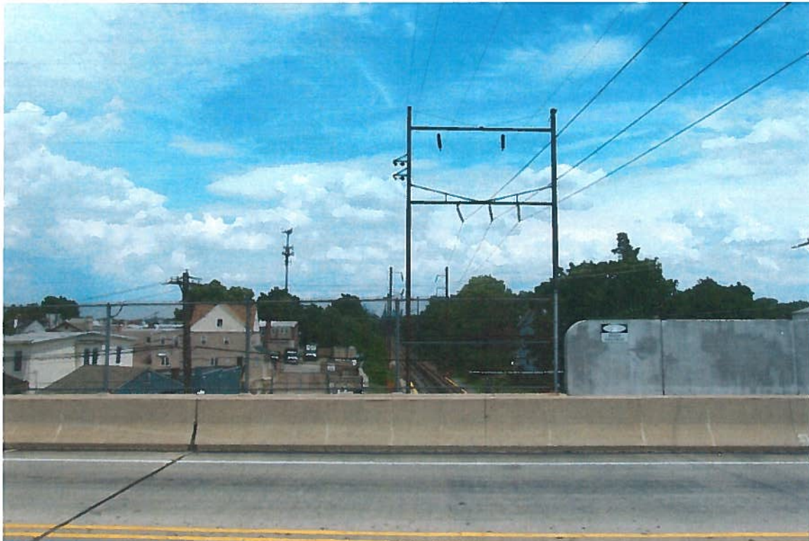
VIEW LOOKING EAST AT THE CHURCH STREET ELEVATED OVERPASS.
