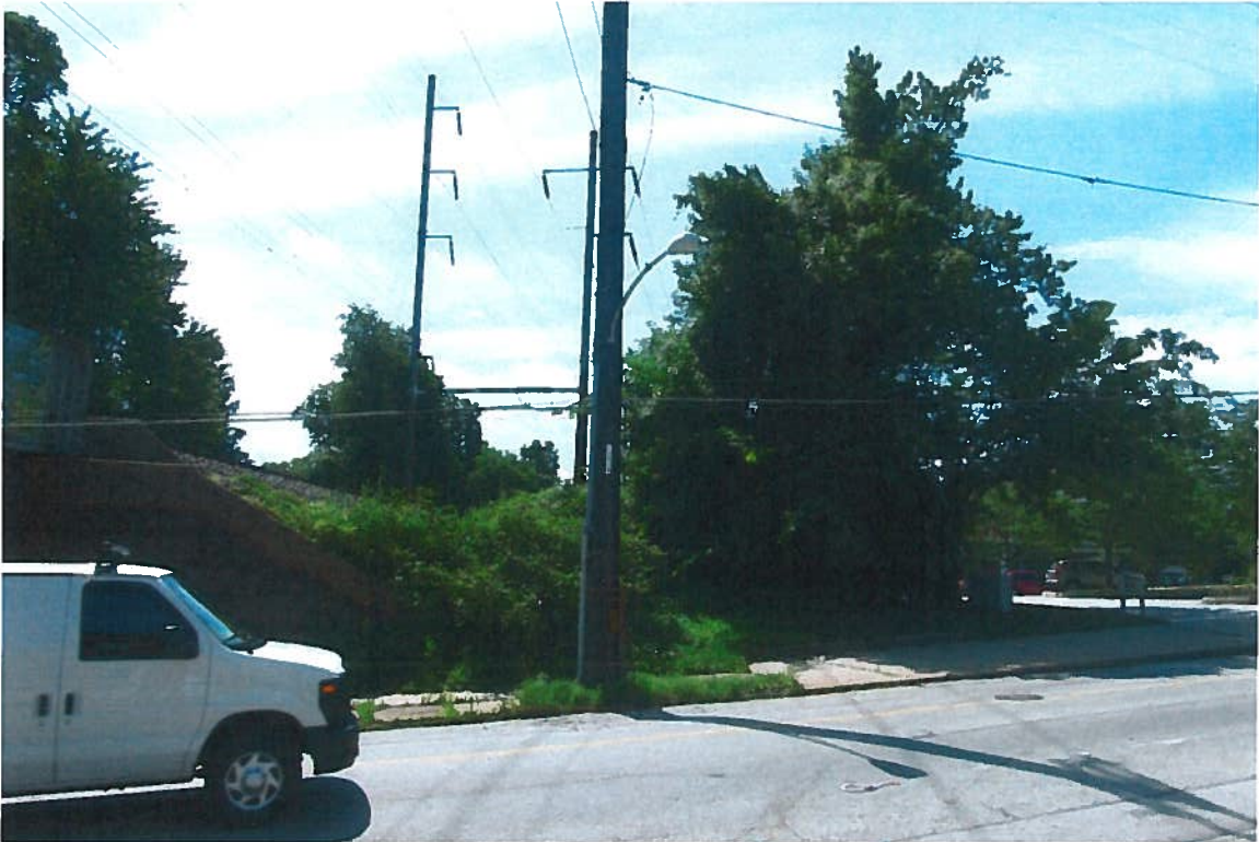
VIEW LOOKING SOUTH FROM MT. PLEASANT AVENUE CROSSING.
