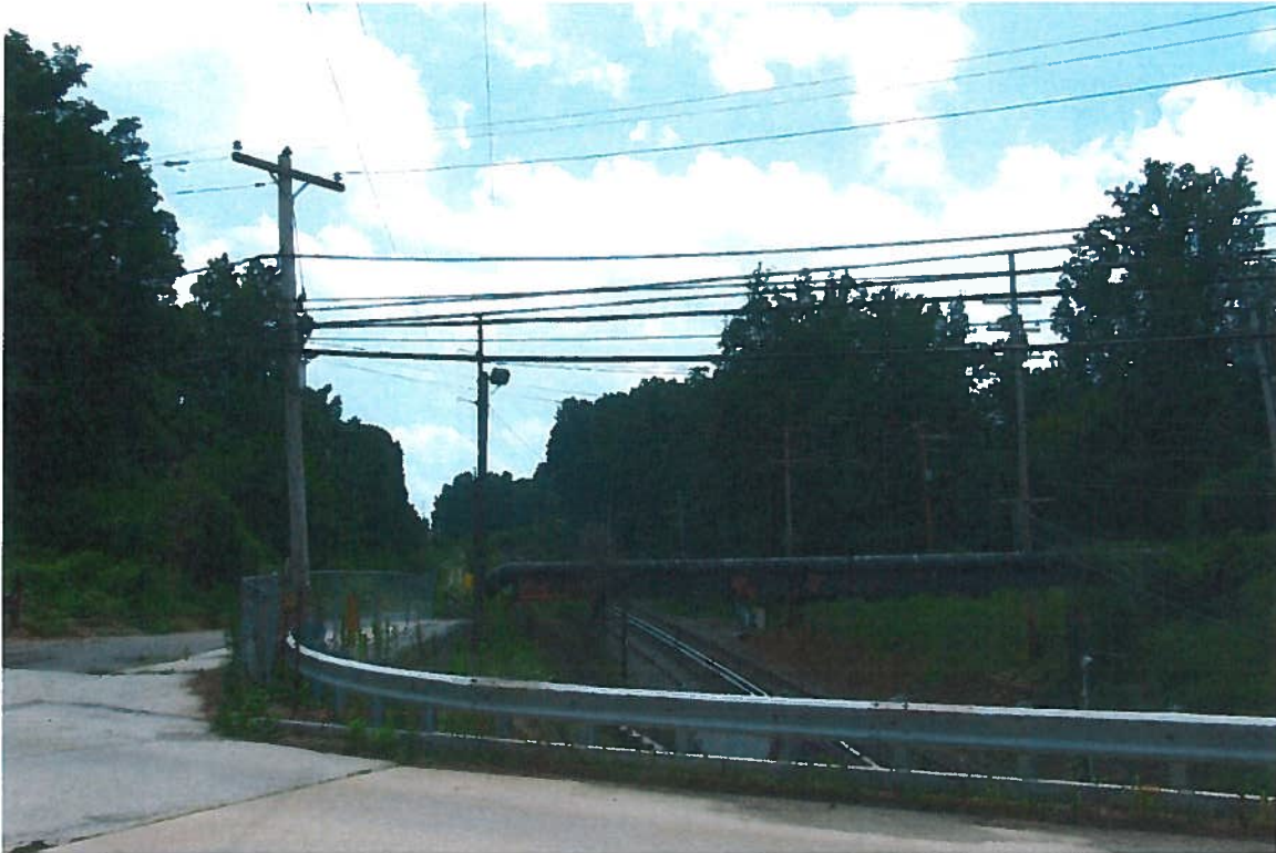
VIEW LOOKING SOUTH AT THE COUNTY LINE ROAD OVERPASS.
