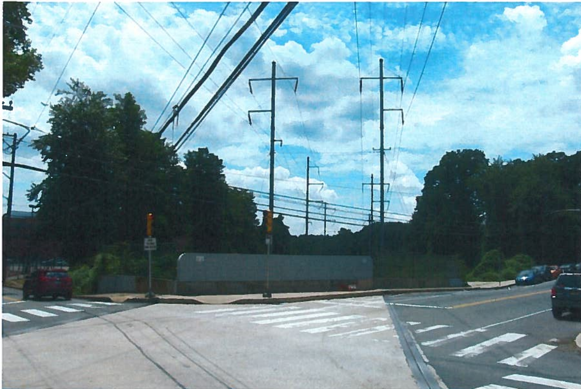
VIEW LOOKING SOUTH AT THE QUEEN LANE OVERPASS.
