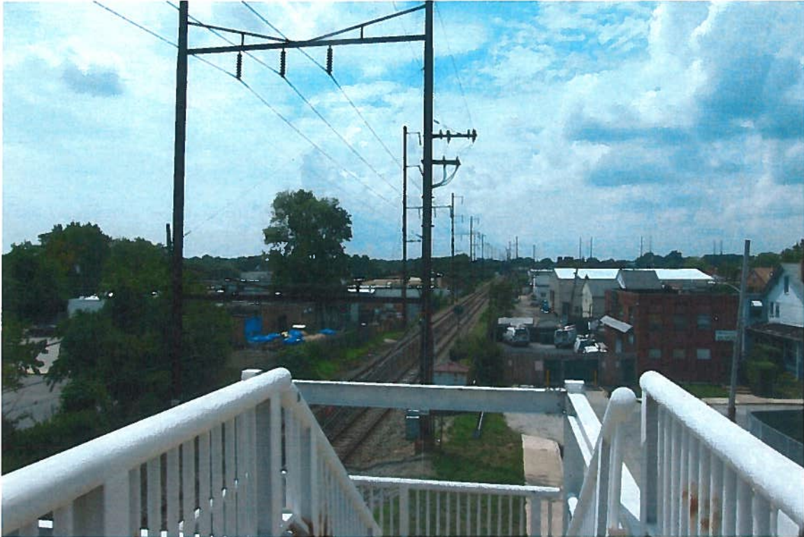
VIEW LOOKING WEST AT THE CHURCH STREET ELEVATED OVERPASS.
