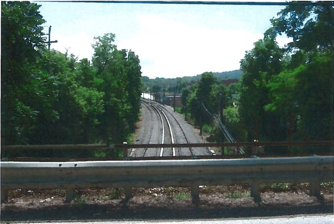
VIEW LOOKING NORTH AT THE CHURCH ROAD OVERPASS.
