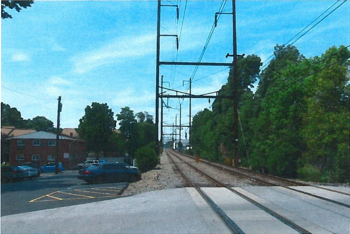
VIEW LOOKING WEST AT THE AMOSLAND ROAD CROSSING.
