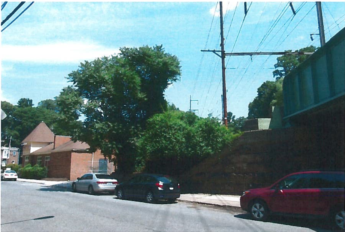
VIEW LOOKING NORTH AT THE GREENE STREET OVERPASS.
