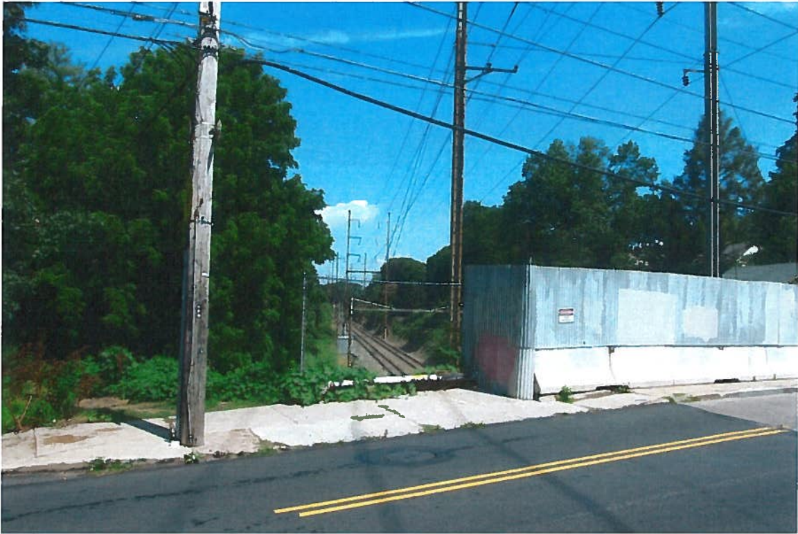
VIEW LOOKING NORTH FROM ALLENS LANE CROSSING.
