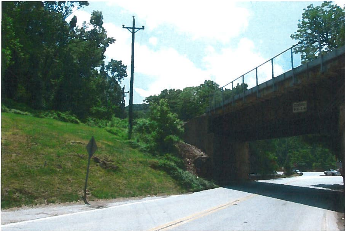
VIEW LOOKING SOUTH AT THE HOLSTEIN ROAD OVERPASS.
