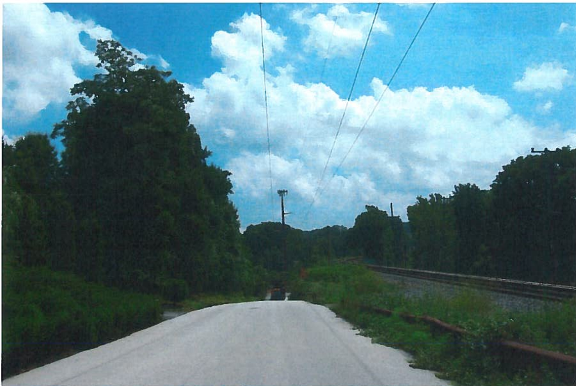
VIEW LOOKING SOUTH ALONG REBEL HILL ROAD. BEGINNING SECTION OF THE HIGH TENSION LINE, IN ADITION TO POLE LINE.
