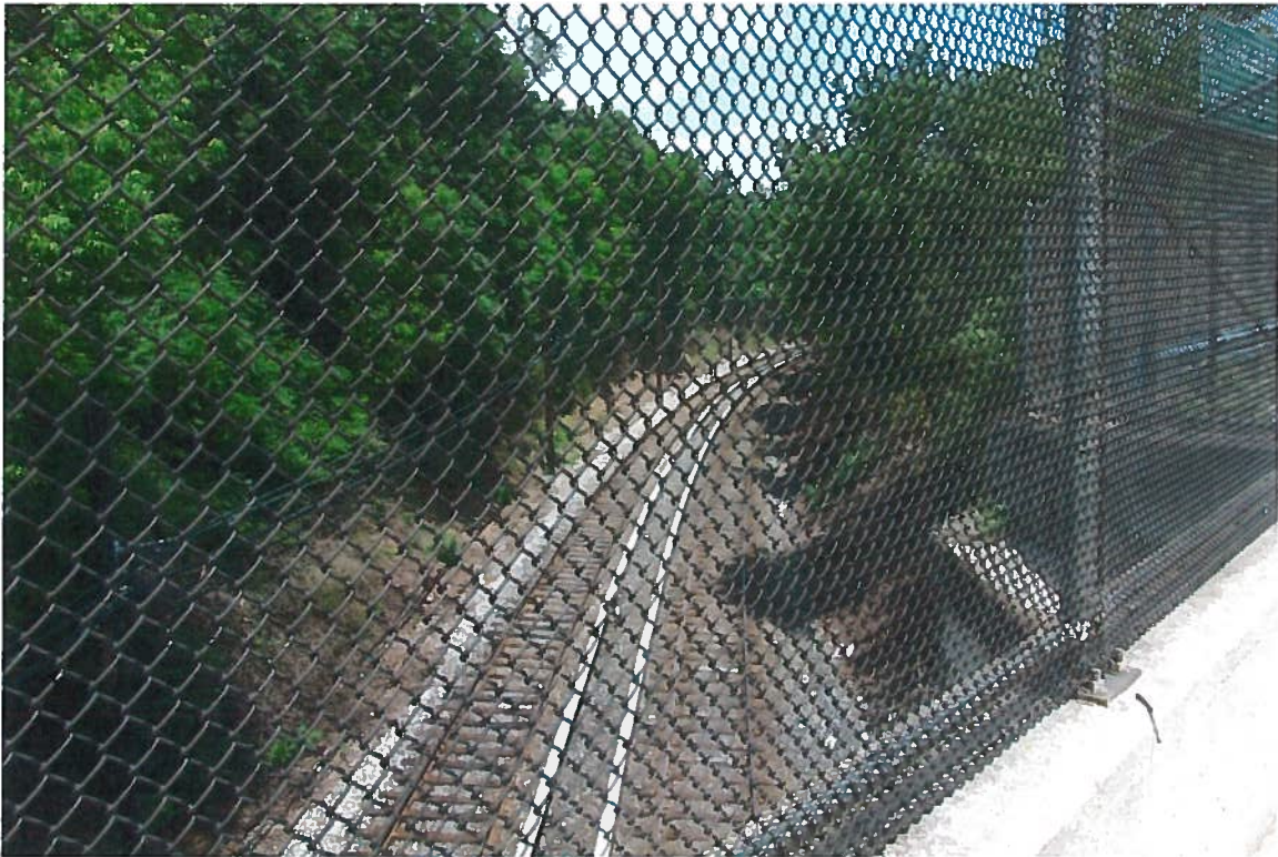
VIEW LOOKING NORTH FROM DEKALB PIKE TOWARD THE NORTH END.
