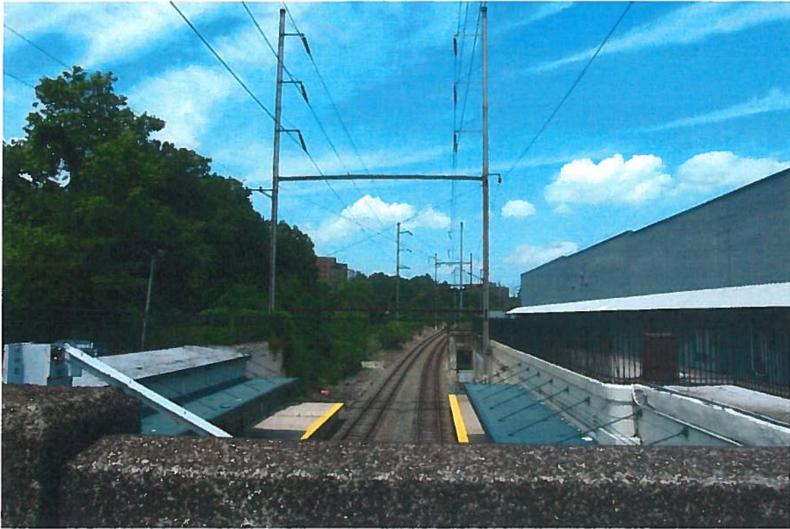
VIEW LOOKING NORTH AT THE CHELTEN AVENUE OVERPASS.
