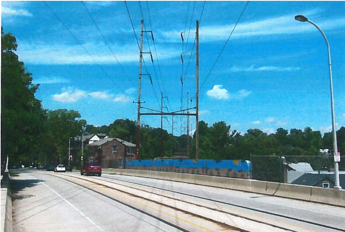
VIEW LOOKING NORTH AT THE WAYNE AVENUE OVERPASS.
