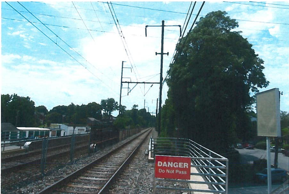
VIEW LOOKING WEST AT THE SPRINGFIELD ROAD OVERPASS.
