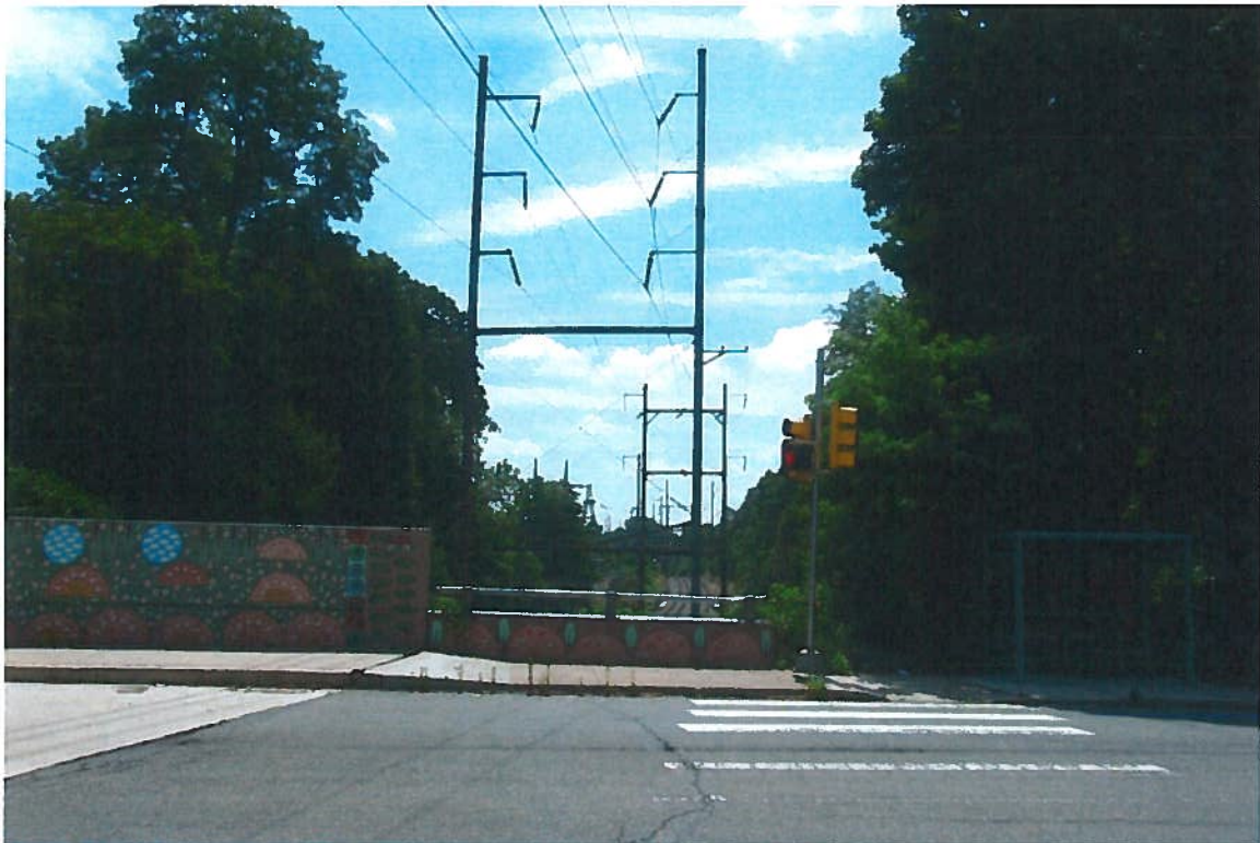
VIEW LOOKING SOUTH AT THE W. WALNUT LANE OVERPASS.
