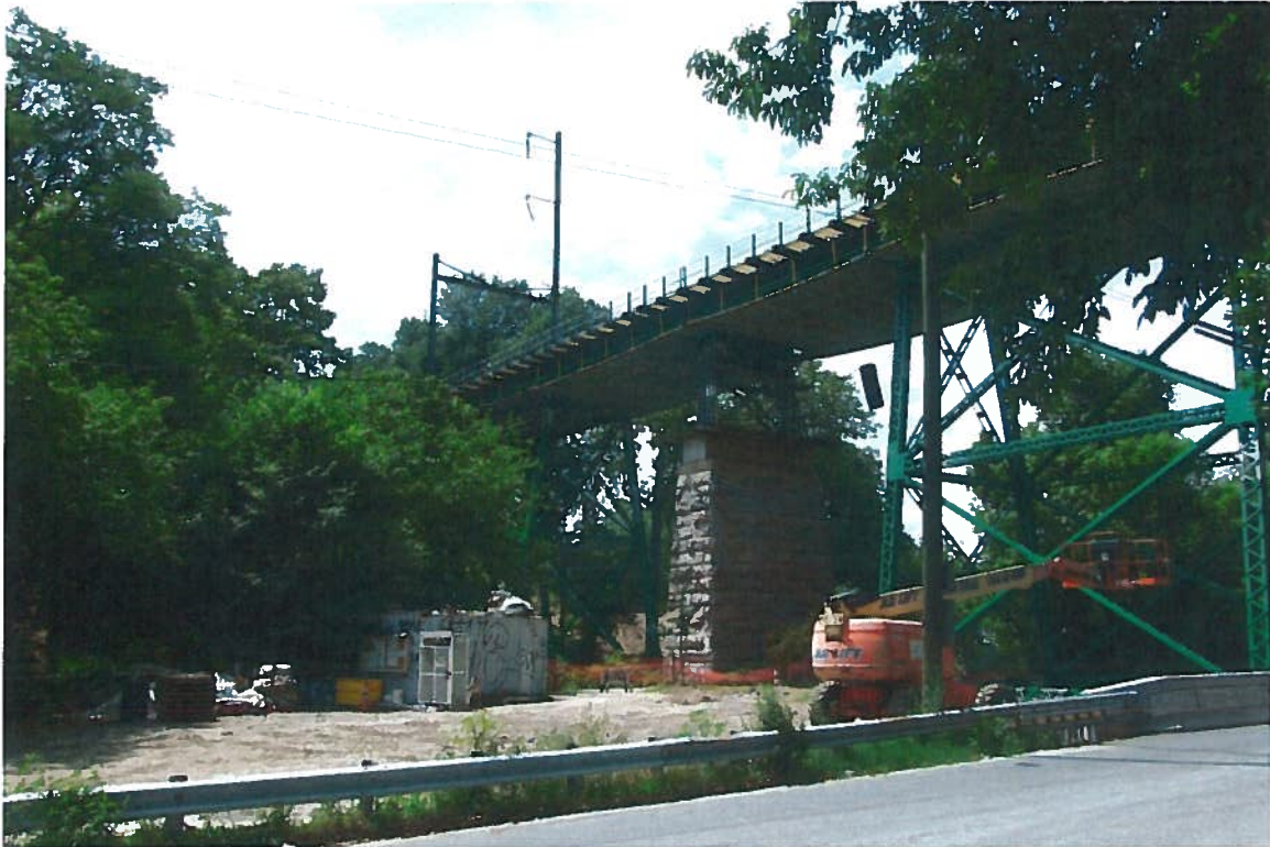
VIEW LOOKING WESTWARD AT THE SCOTTDALE AVENUE ELEVATED OVERPASS.
