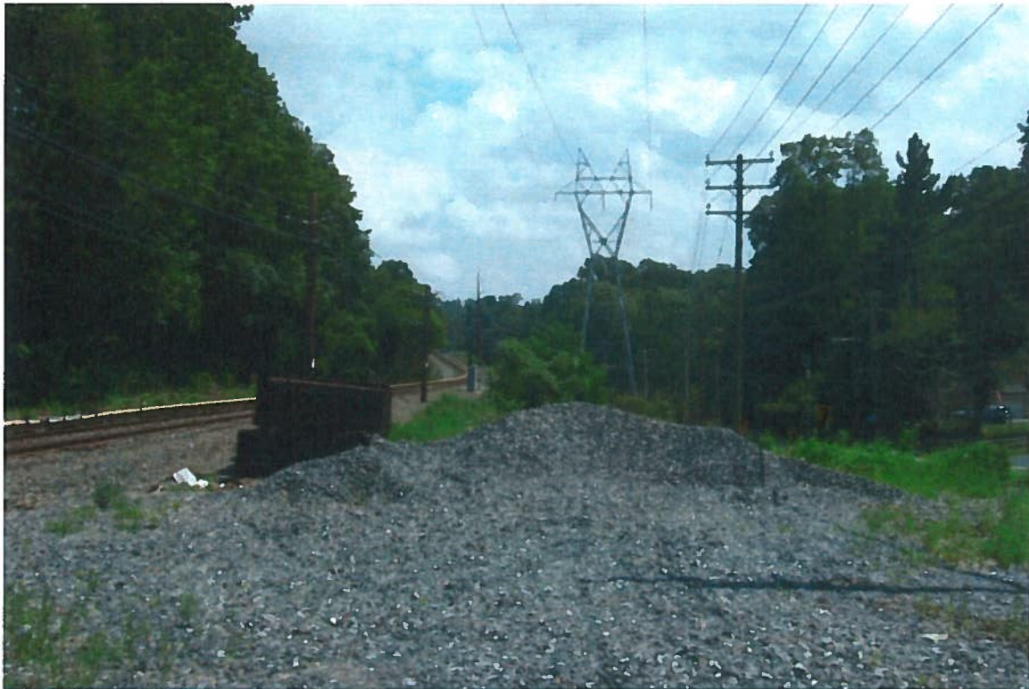
VIEW LOOKING SOUTH JUST NORTH OF THE CONESTOGA ROAD OVERPASS.
