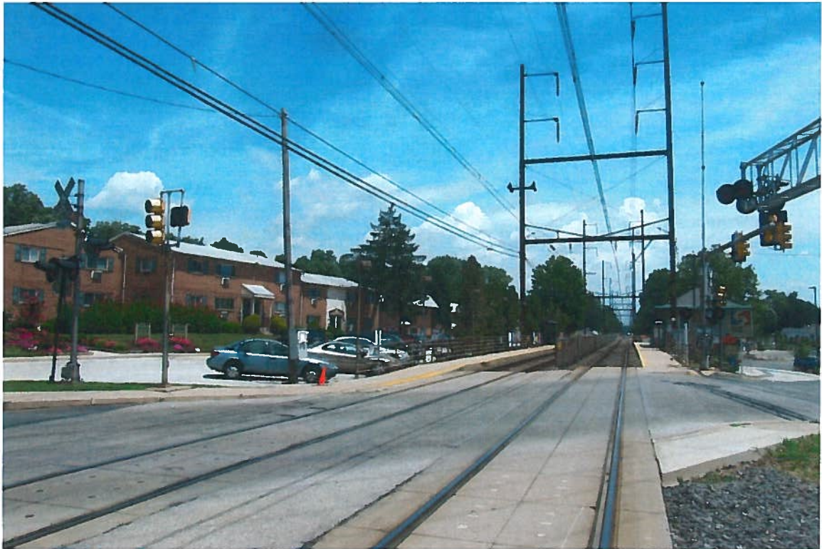
VIEW LOOKING EAST AT THE SOUTH AVENUE/PROVIDENCE ROAD CROSSING.
