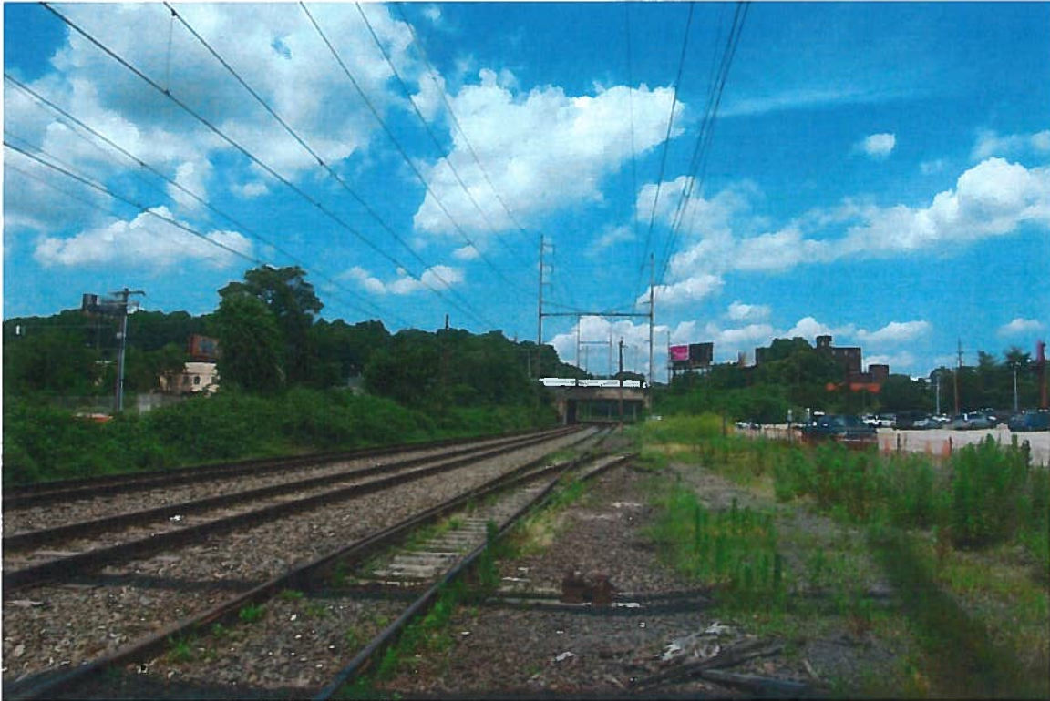
VIEW LOOKING NORTH FROM SOUTH OF THE US ROUTE 1 EXPRESSWAY.
