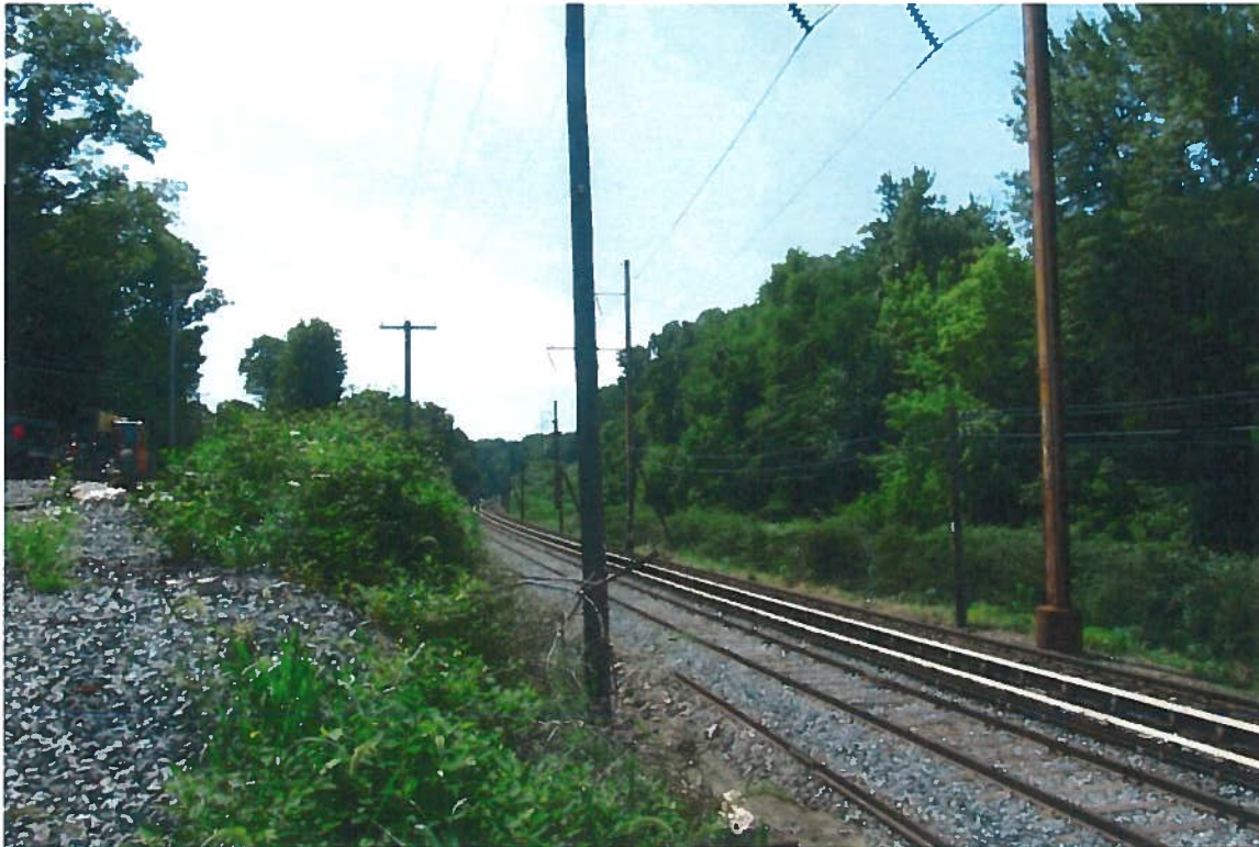
VIEW LOOKING SOUTH FROM JUST SOUTH OF EAGLE ROAD.
