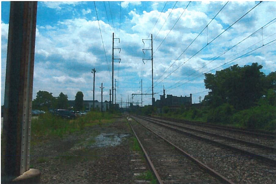
VIEW LOOKING SOUTH FROM JUST NORTH OF ROBERTS AVENUE, NEAR THE SOUTH END OF THE LINE.
