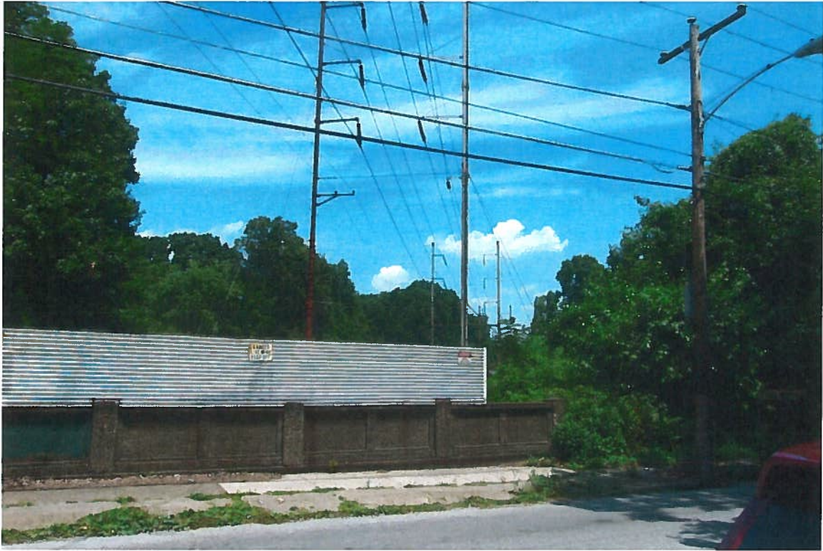
VIEW LOOKING NORTH AT THE JOHNSON STREET OVERPASS.
