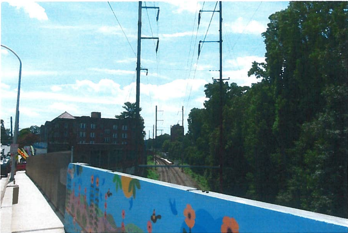
VIEW LOOKING SOUTH AT THE WAYNE AVENUE OVERPASS.
