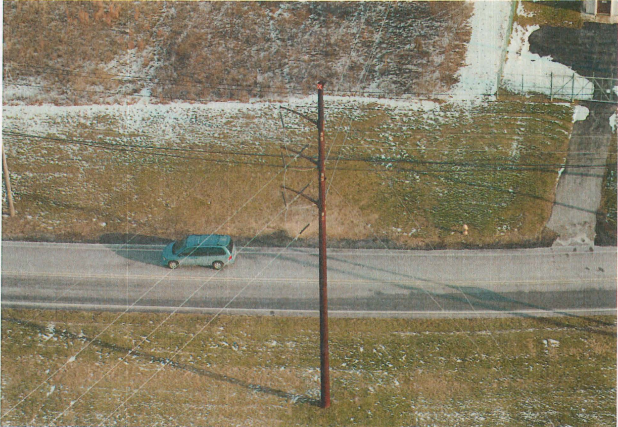
FIGURE 5 – TYPICAL 138/69 kV ANGLE POLE
