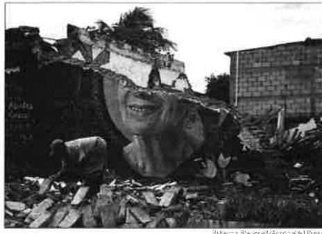
A man recovers bricks from a building destroyed in Thursday's magnitude 8.1 earthquake, in Union Hidalgo, Oaxaca state, Mexico on Sunday.
