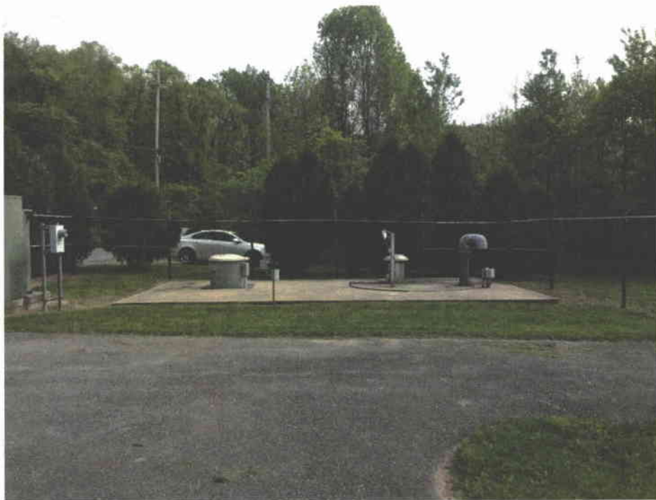
Valve Pit and Wet Well
