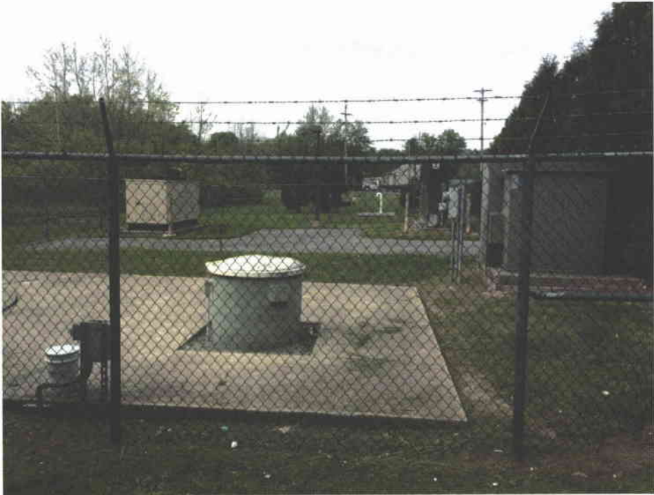
Access to Valve Pit
