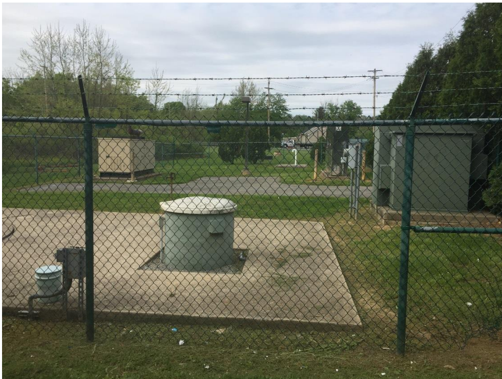
Access to Valve Pit
