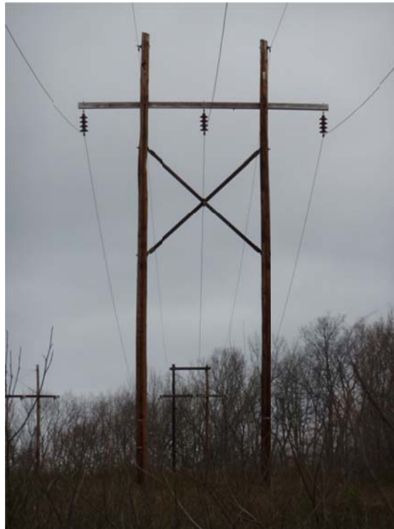
Photo 1 – Typical wood h-frame structure
