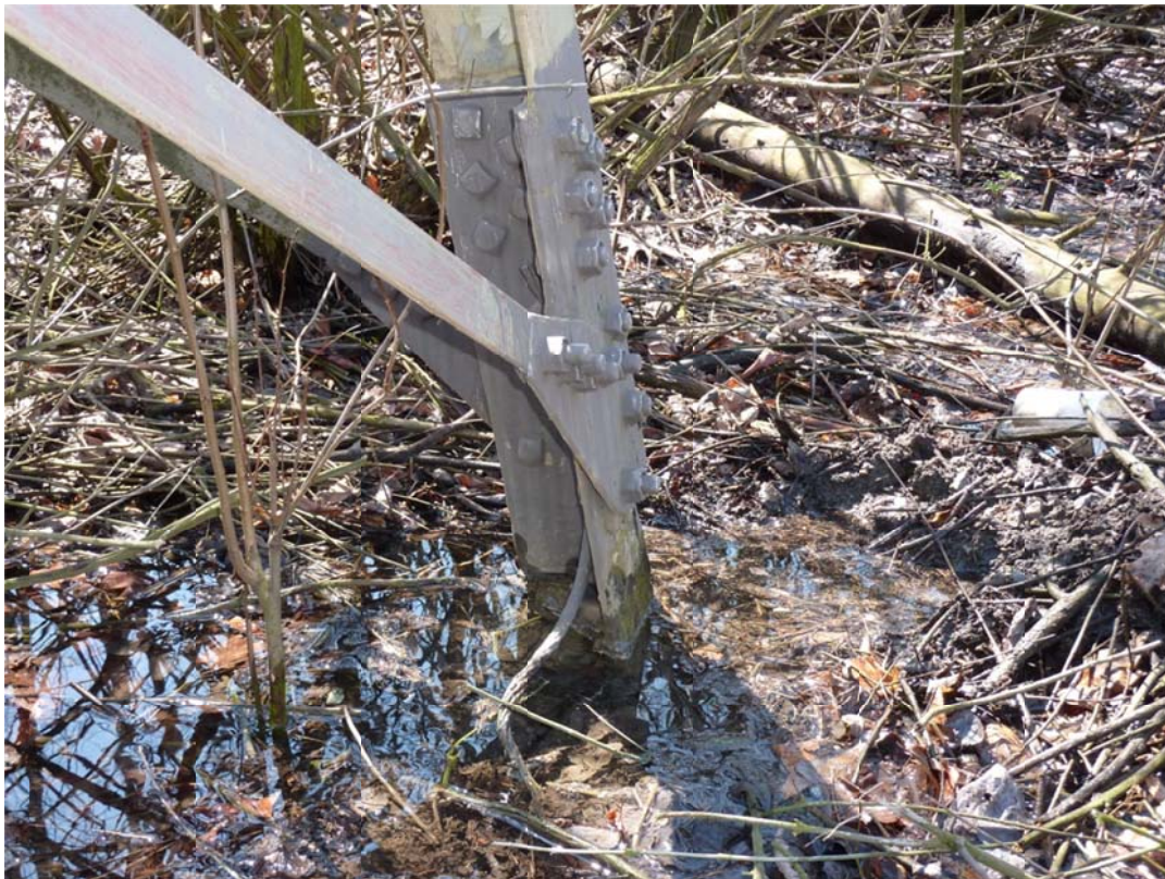
Photo 9 – Submerged Concrete Foundation (Structure Inspection No. 70)
