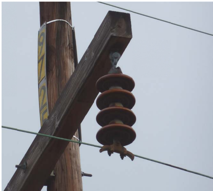
Photo 6 – Typical suspension insulator string
