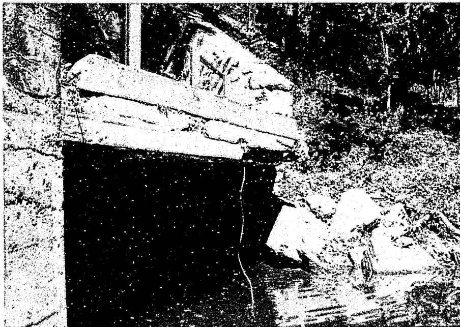
3. South end of east abutment. Abutment failure. Note that the stringers are unsupported.
