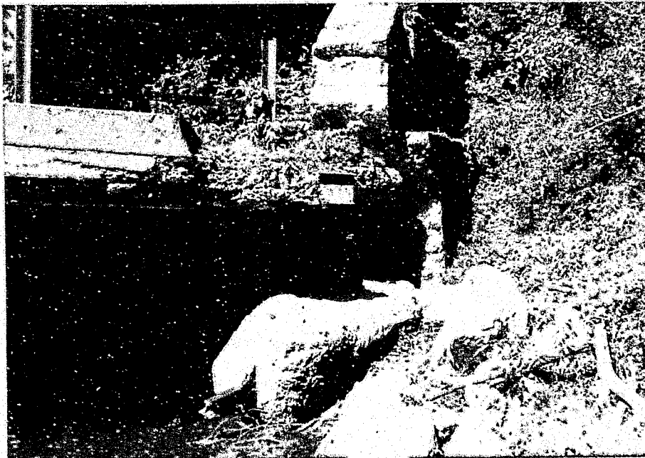
3. South end of east abutment. Abutment failure. Note that the stringers are unsupported.
