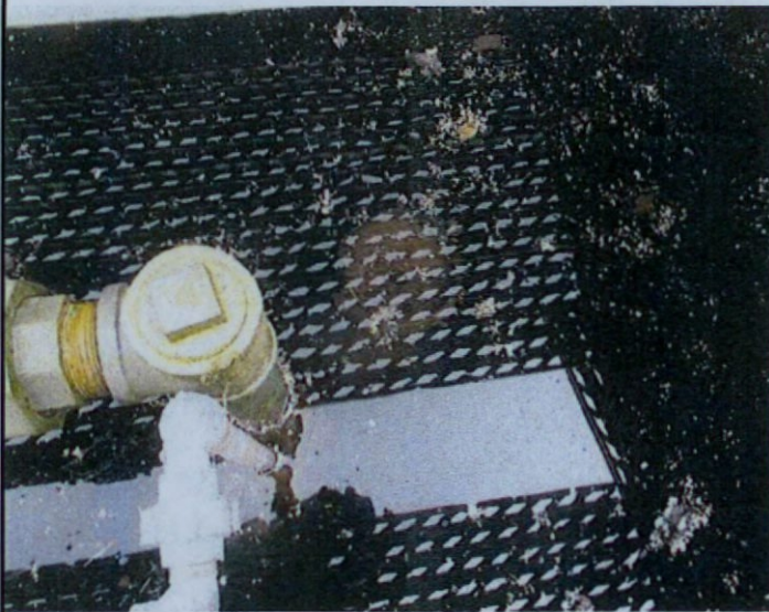
Image 3: Photo taken by Michael Benham on 6/21/18. Shows RH train's clarifier skimmer. Skimmer was blocked with scum and algae.
