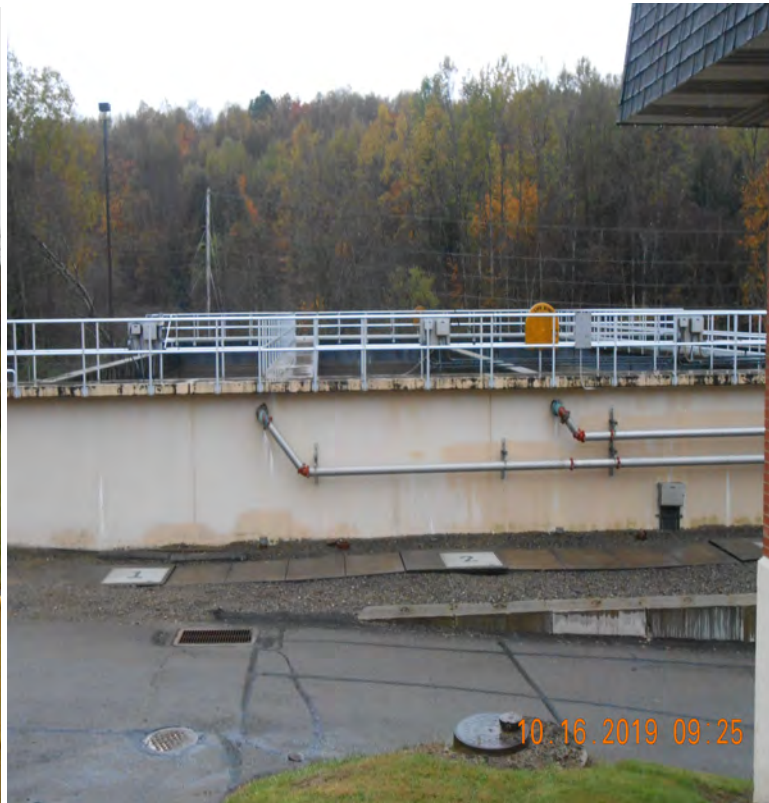
Pine St. WWTP – SBR Tanks
