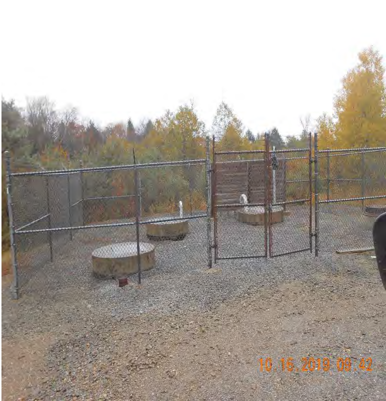
(Northwest) Zooks Pump Station Flows to Pine St. WWTP
