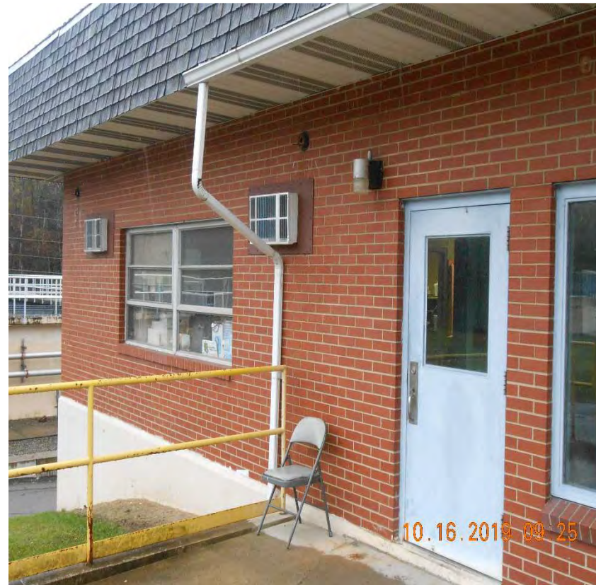
Pine St. WWTP – Office/Central Building
