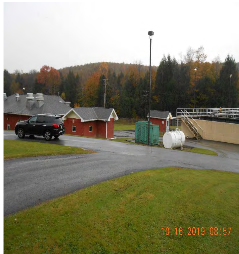
SBR Treatment – Office/Central Building
