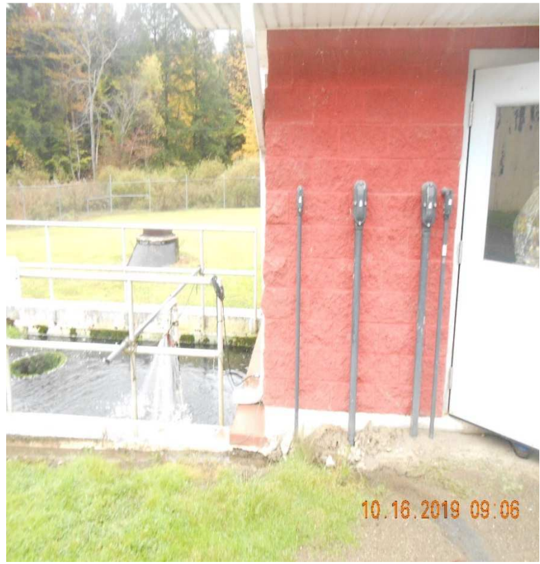
Kinzua WWTP - Effluent Building
