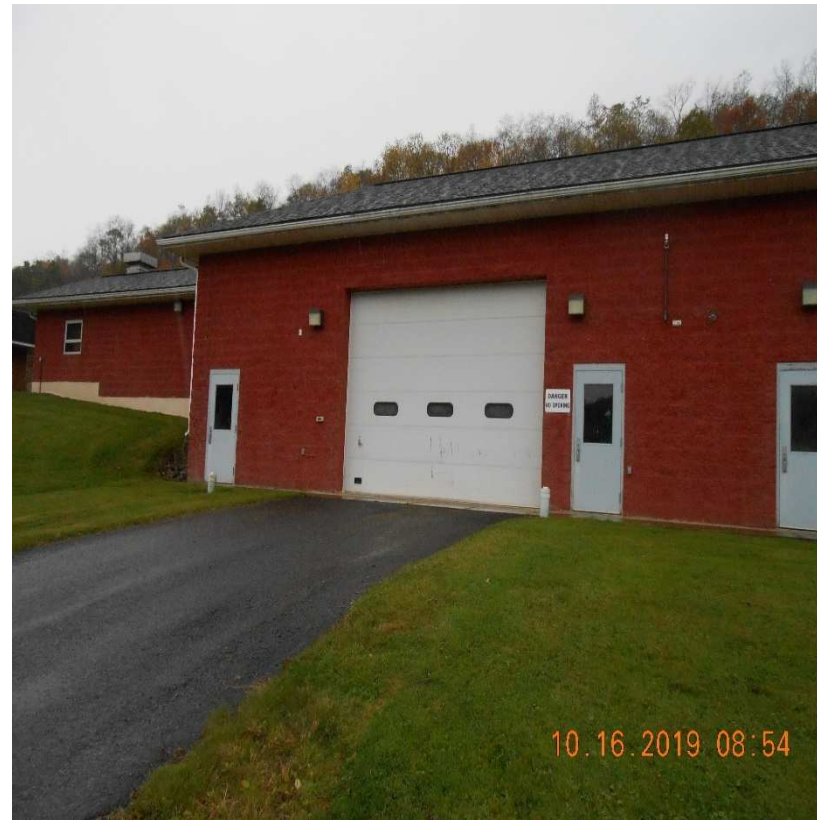
Kinzua WWTP – PTS Building
