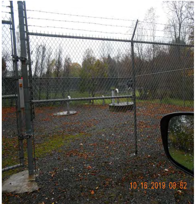
West Kane Pump Station Flows to Pine St. WWTP
