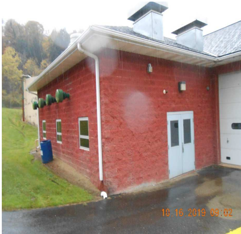
Kinzua WWTP - Blower Building
