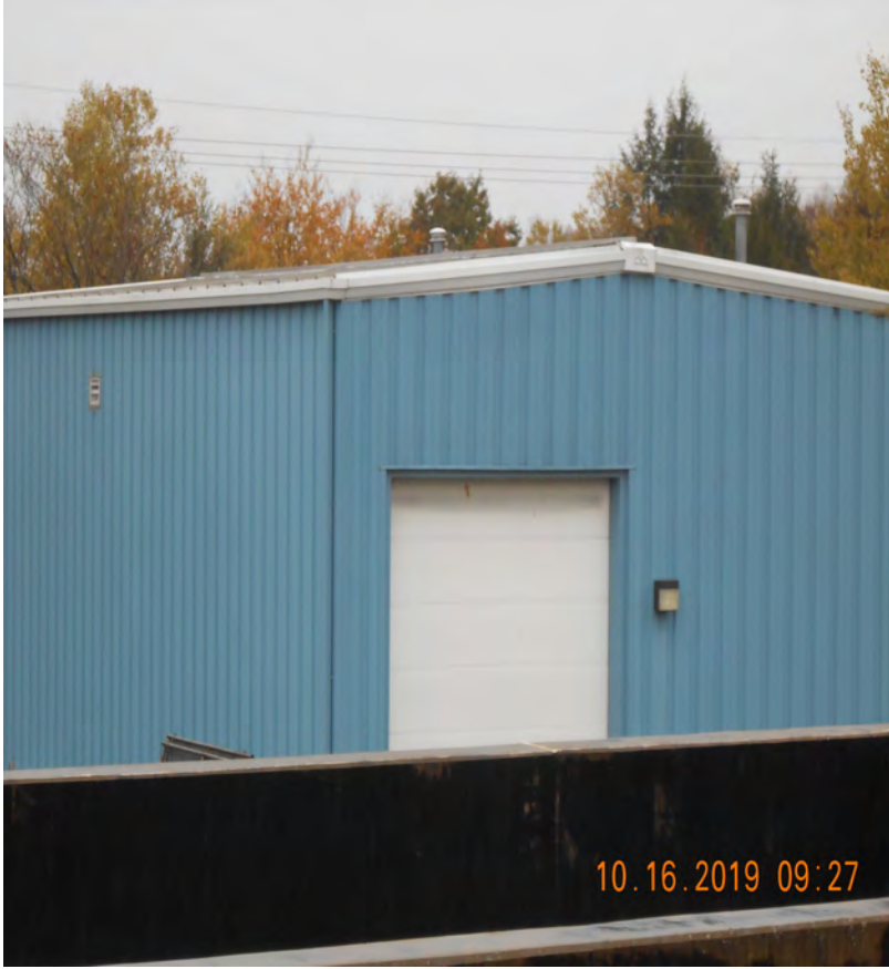
Pine St. WWTP – Storage/Garage Building
