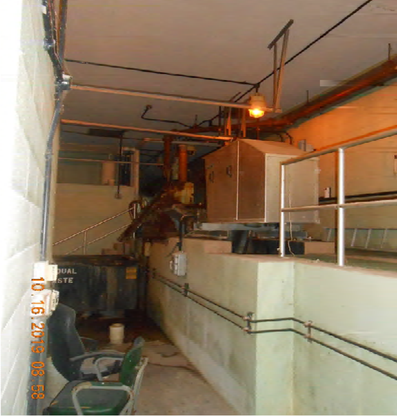
Kinzua WWTP – PTS Building
