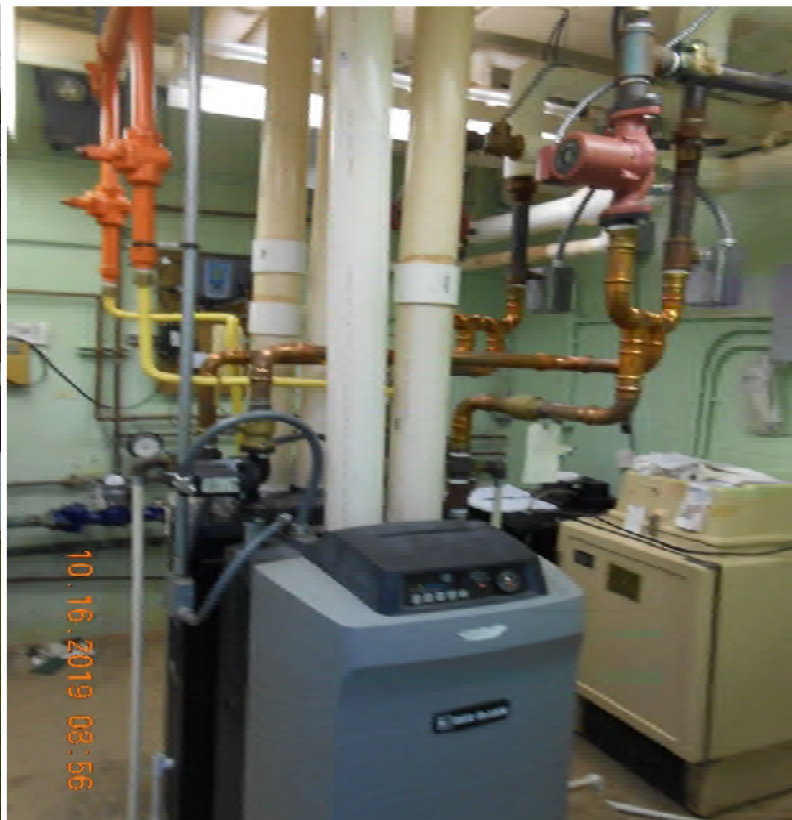
Kinzua WWTP – PTS Building
