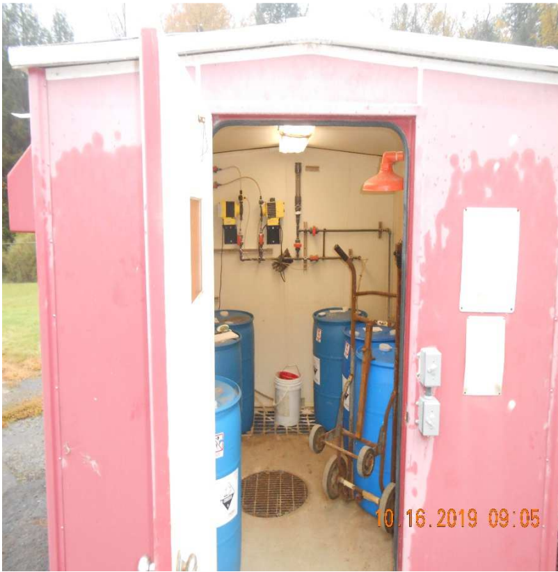
Kinzua WWTP - Chemical Building
