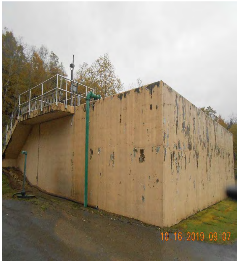
Kinzua WWTP - Digesters
