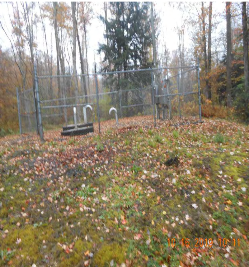
West Wind Pump Station Flows to Pine St. WWTP
