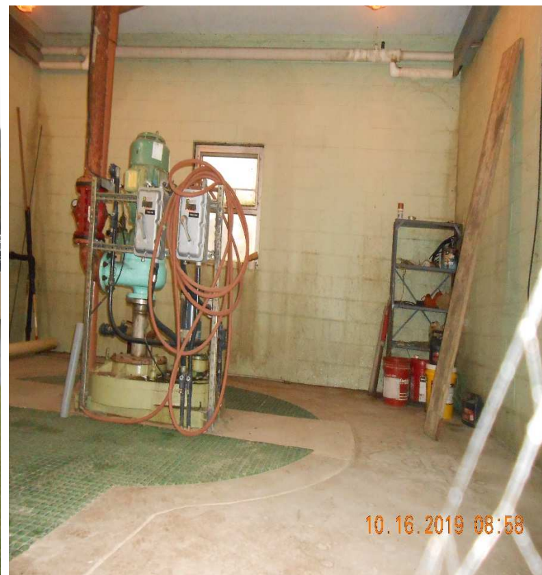
Kinzua WWTP – PTS Building
