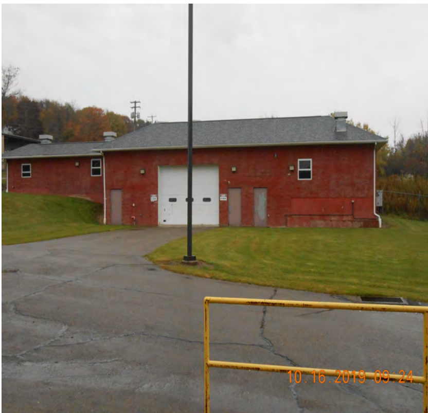
Pine St. WWTP – PTS Building
