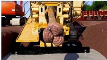
Horizontal directional drilling is a steerable, trenchless method used when installing pipelines that minimizes impact on the environment and communities.
