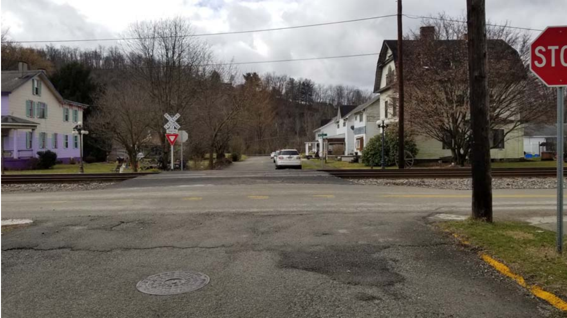
Griscom Street crossing looking from the north side of crossing.
