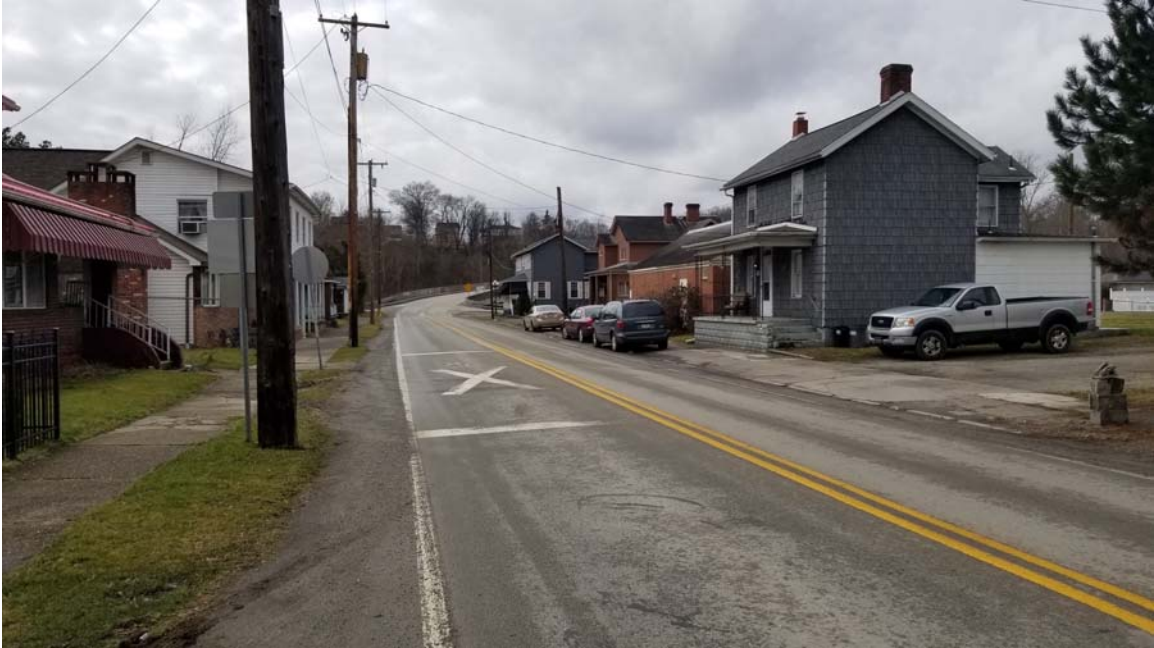
Laughlin Street (SR 0819) crossing pavement markings on south side of crossing.
