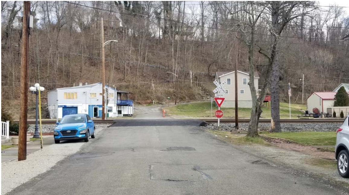
Crossing signs at Strickler Street on the south side of crossing.
