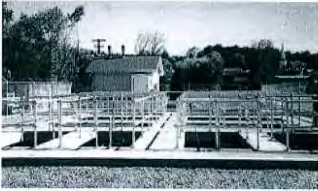
130,000 GPD tertiary filter stream discharge Valley Green Development, Montgomery County, PA
