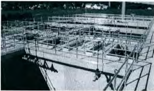
240,000 GPD stream discharge Salisbury Township, Lancaster County, PA
