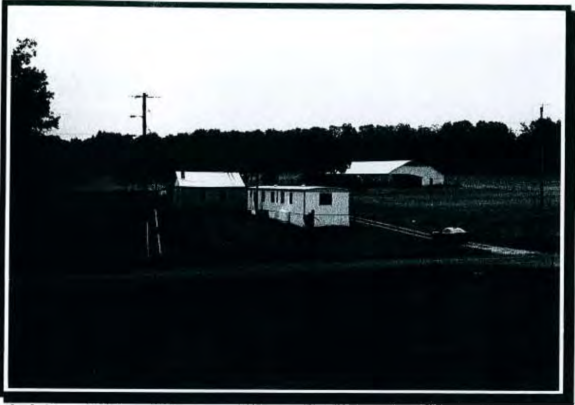
PHOTO #13 – Existing mobile home, CMU and frame sheds on north side of Martin Road
