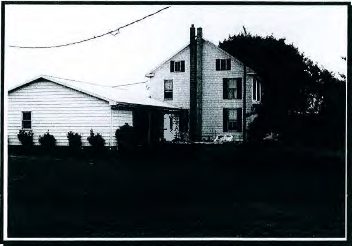
PHOTO #4 – South elevation of existing 2-1/2 story dwelling and frame garage
