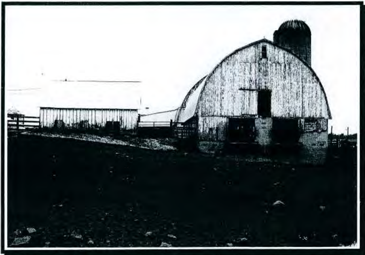
PHOTO #8 – North elevation of northern livestock barn
