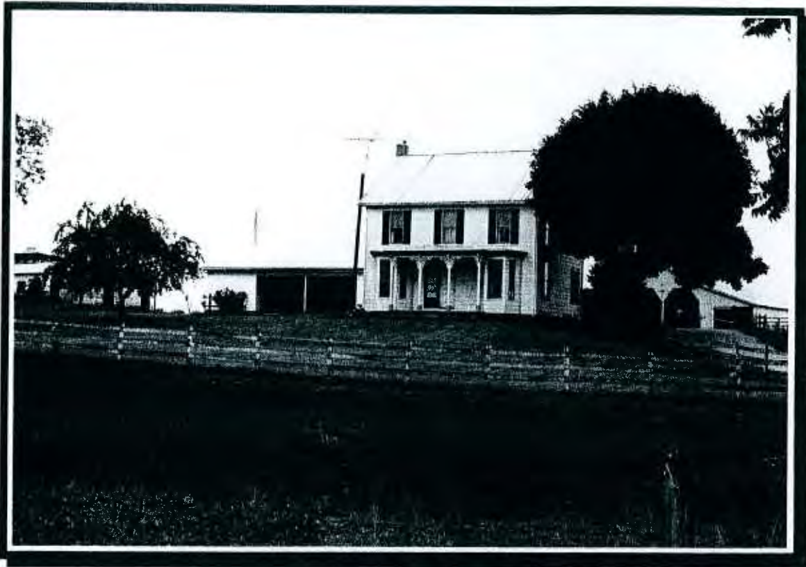
PHOTO #1 – East elevation of existing 2-1/2 story frame dwelling
