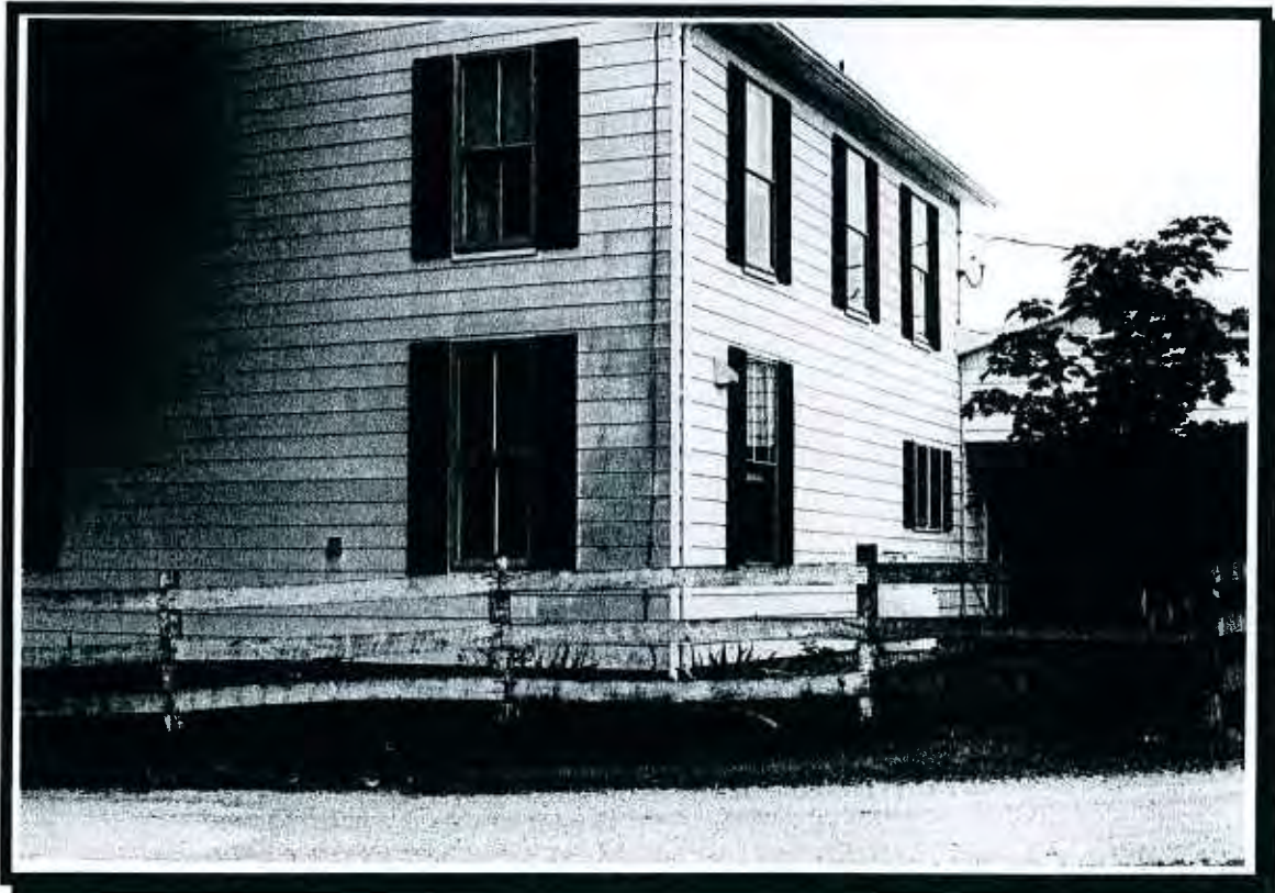
PHOTO #6 - Northwest corner of existing 2-1/2 story frame dwelling
