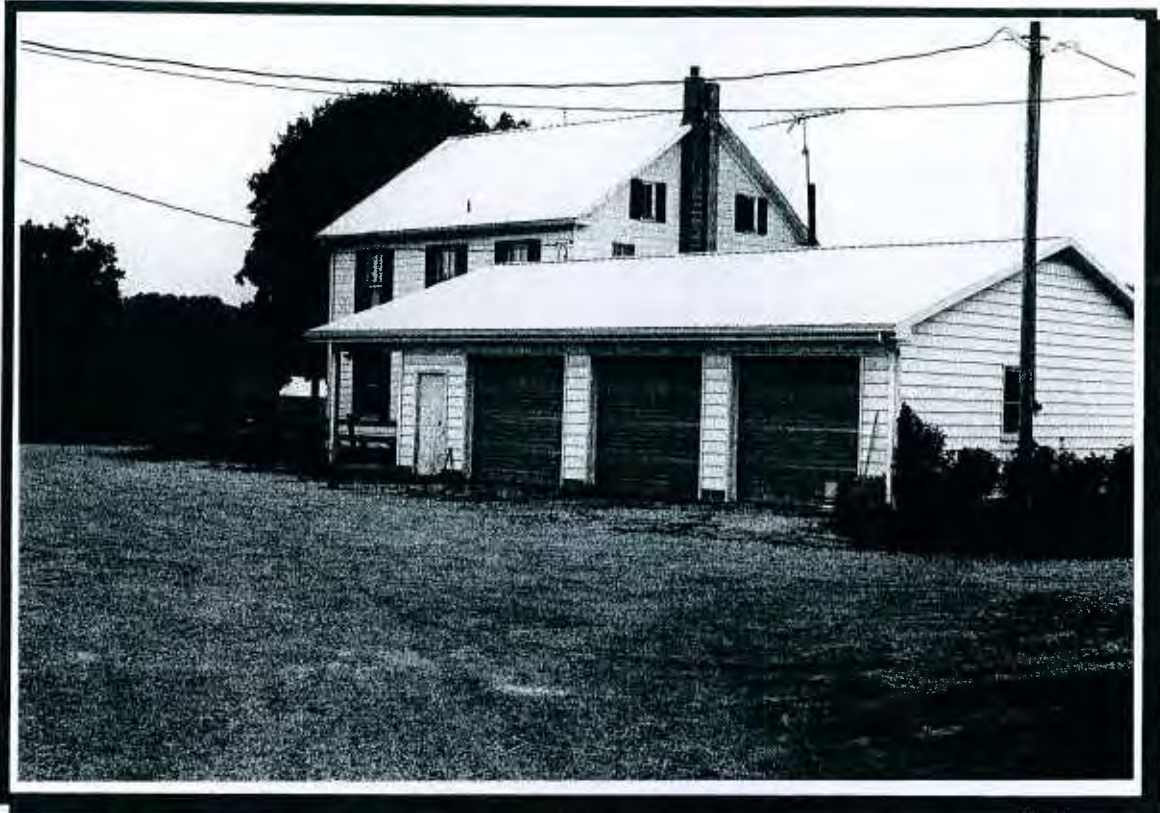
PHOTO #3 – West elevation of existing 2-1/2 story dwelling and frame garage
