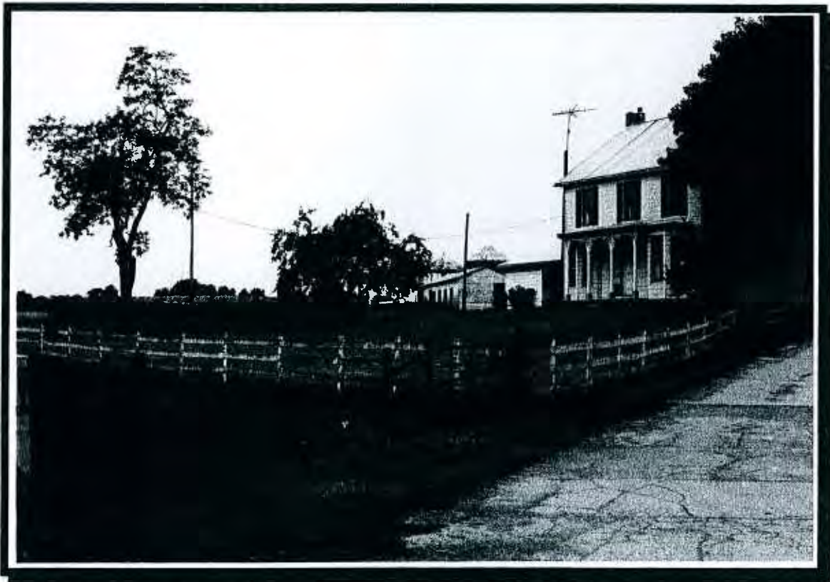
PHOTO #2 – East elevation of existing 2-1/2 story dwelling and miscellaneous out buildings
