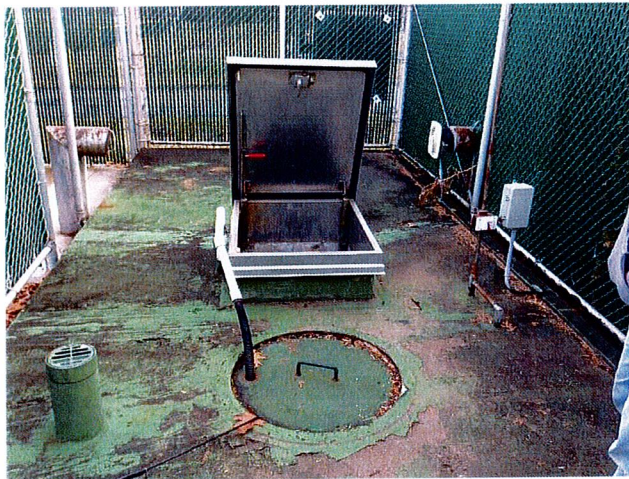
Figure 3 – Dry Pit Entry Hatchway
