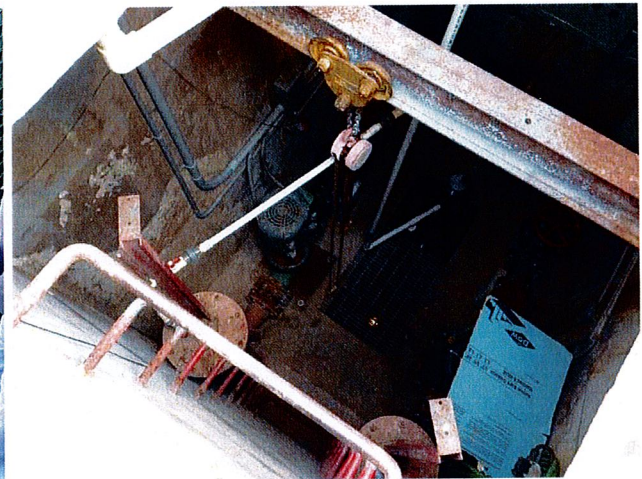
Figure 4 – View into Dry Pit from above
