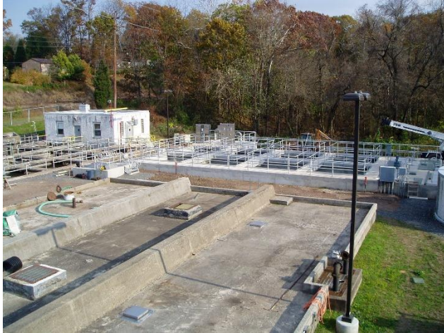
Figure 1 – Lab Building, Secondary Settling Tanks #2 & #3, Sludge Storage Tanks
