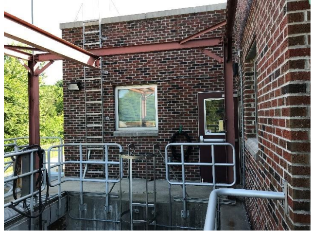
Figure 6 – Office entrance and wetwell
