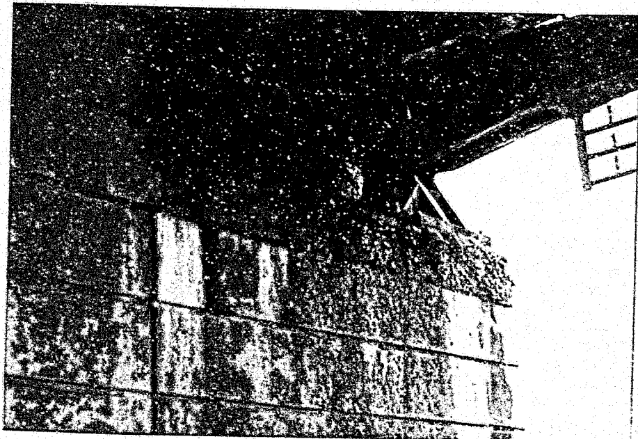
EAST CORNER SPALLING AT NORTH ABUTMENT
