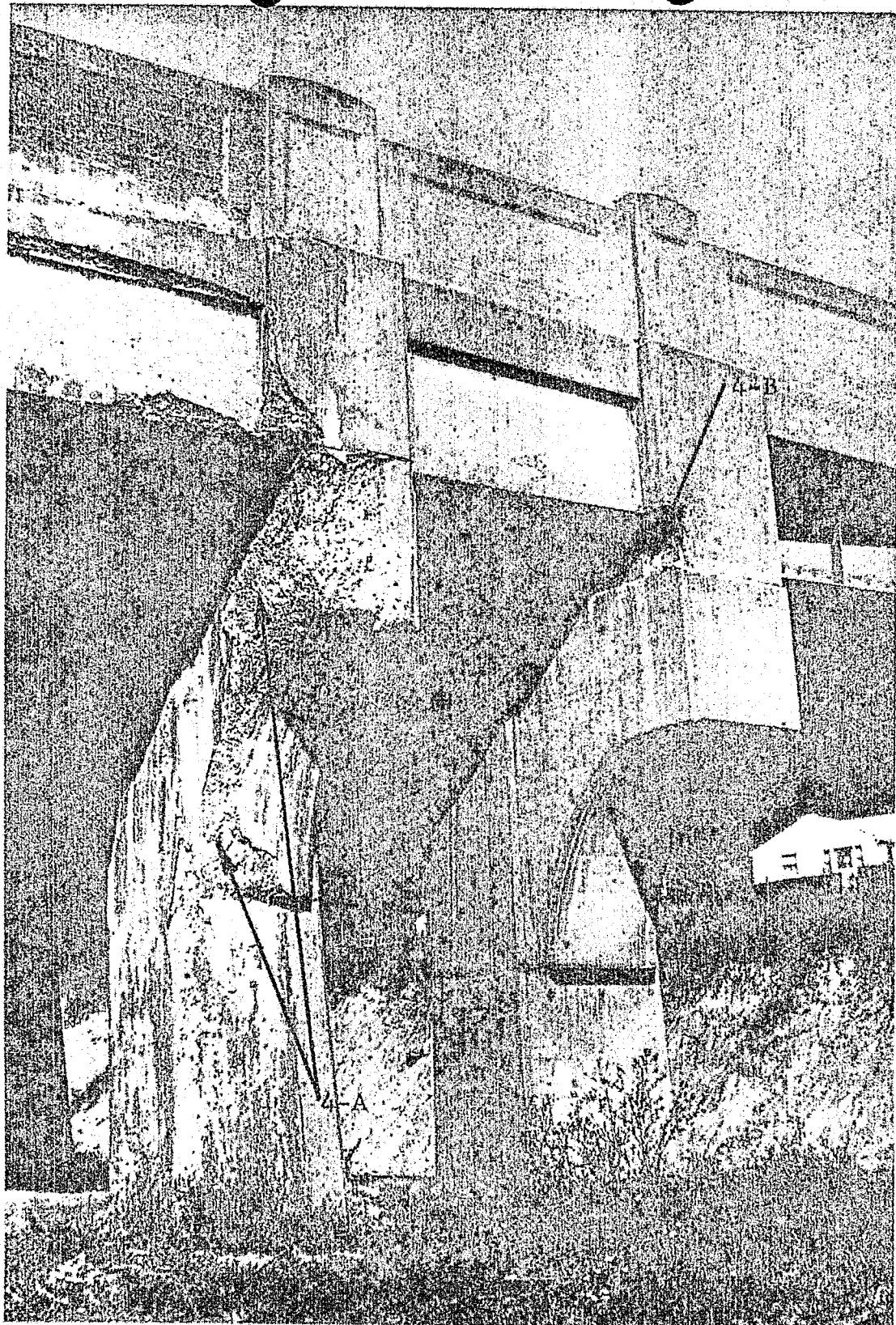
East sides of Pier "0" and Pier "1", looking northwest
