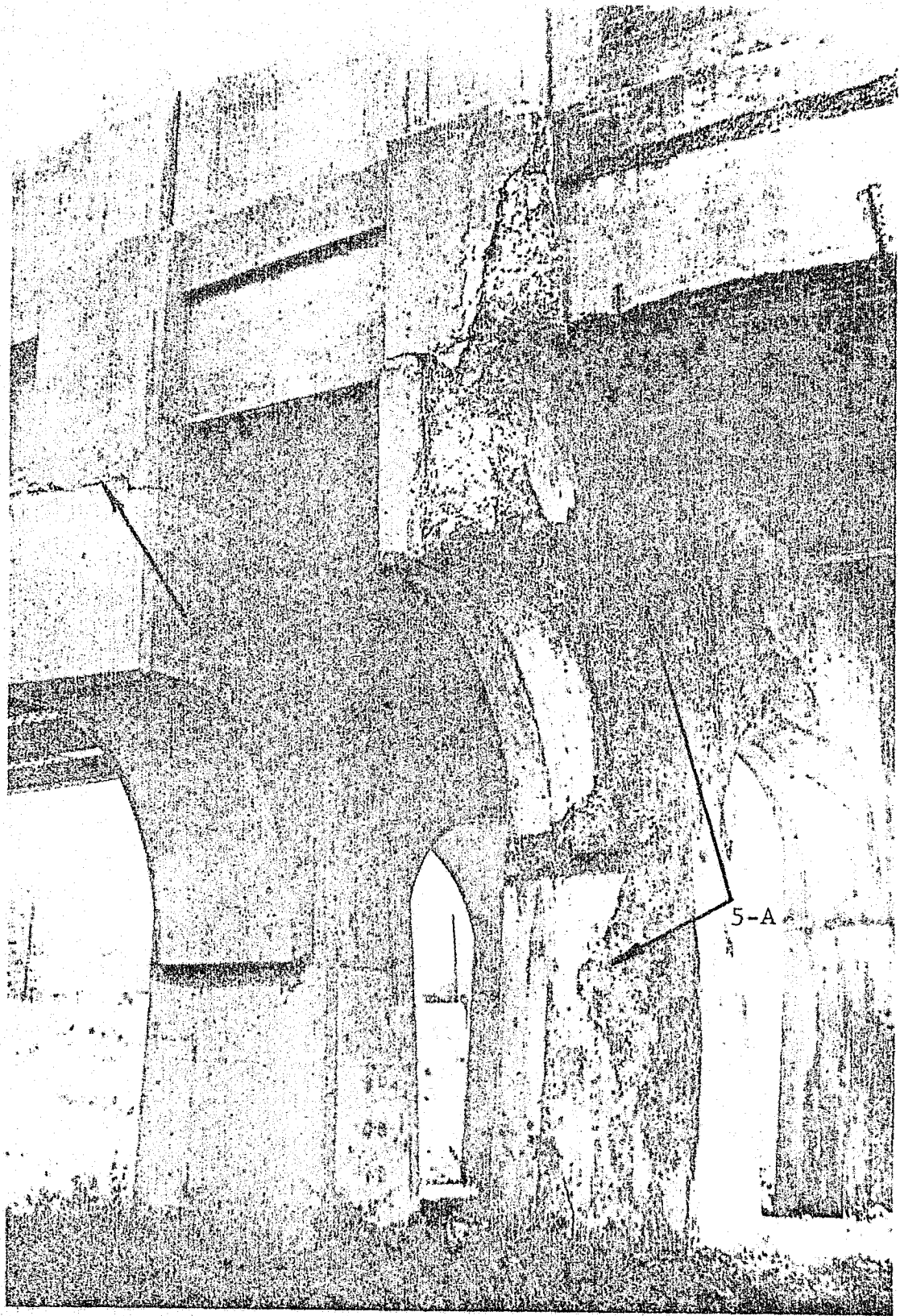
West sides of Pier "0" and Pier "1", looking northeast
