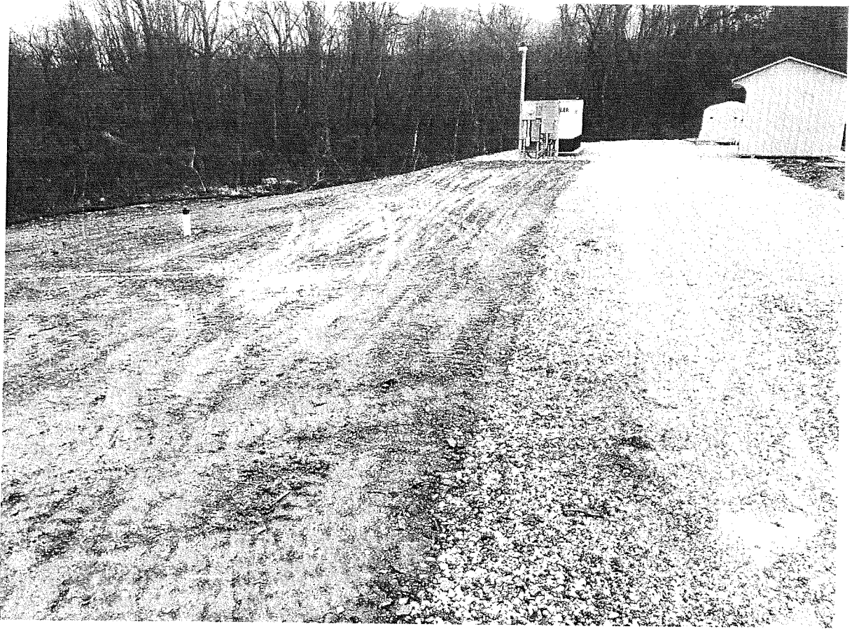
Location of Former Wastewater Treatment Facility (New Pumping Station and Generator Shown in Background) Date of Photo: February 10, 2020
