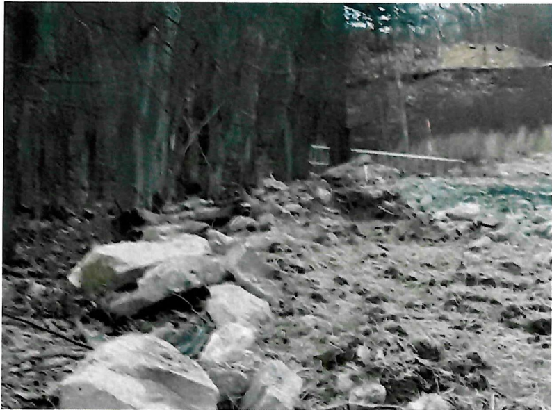
Excavation off the ROW west of the Pole 75 Crane Pad, and well beyond the earth disturbance limits cited in the E & S Plans, Attachment 114.
