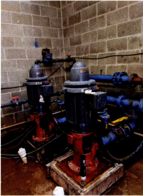
Figure 5 – WTP, booster pumps
