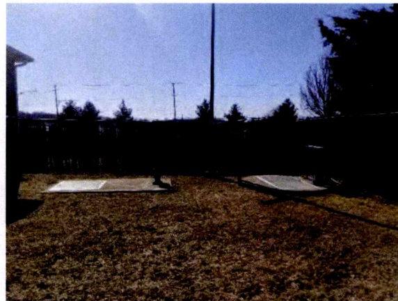
Figure 2 – Wet Well Exterior
