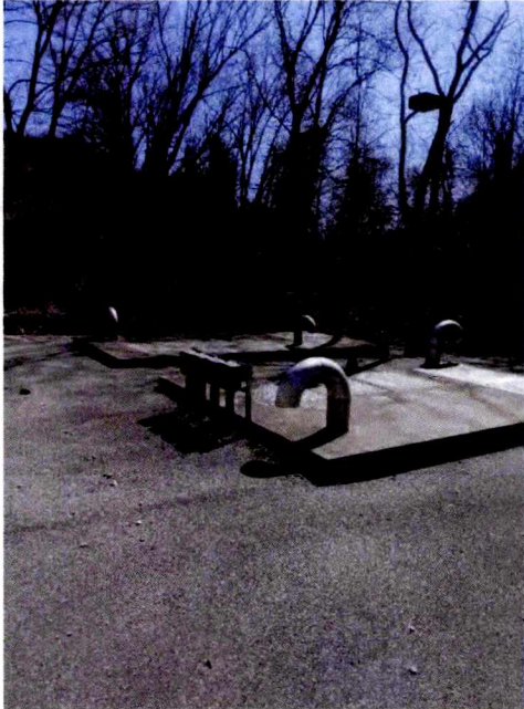
Figure 1 – Wet Well Exterior
