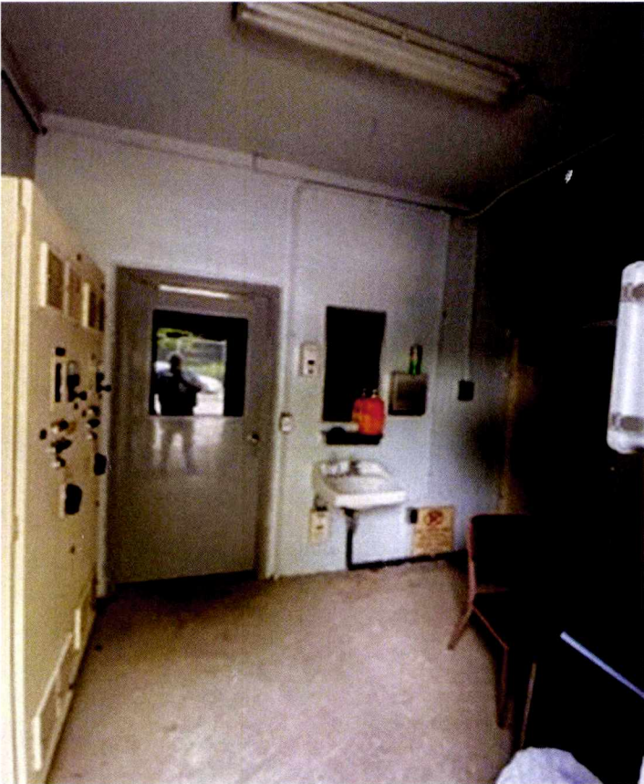
Rock Run Sewer Pump Station
