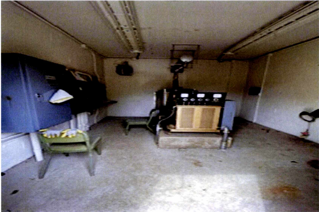
Country Ridge Sewer Pump Station
