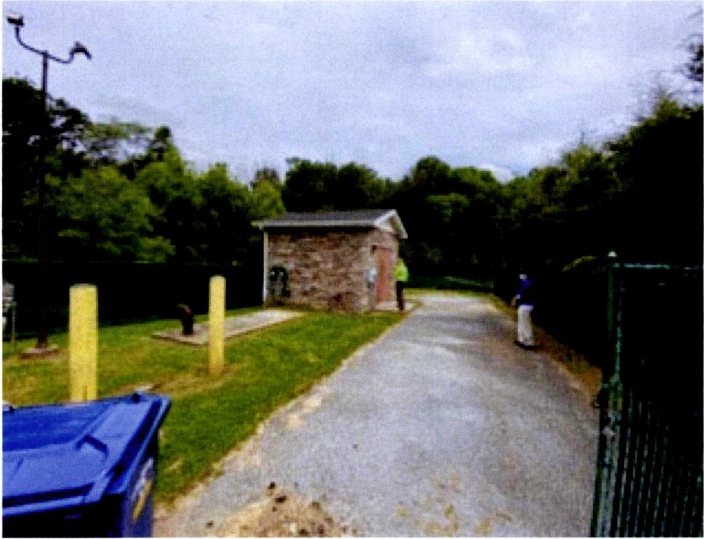
Round Hill #1 Sewer Pump House
