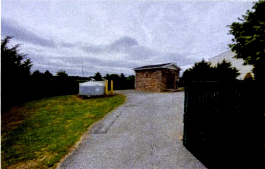
Round Hill #2 Sewer Pump Station
