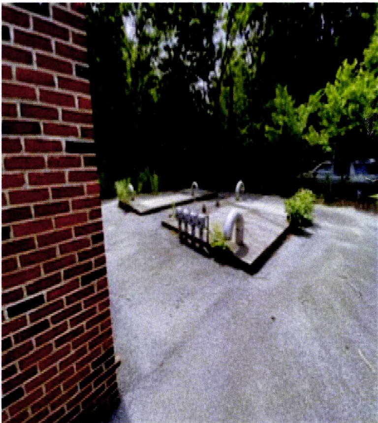
Rock Run Sewer Pump Station
