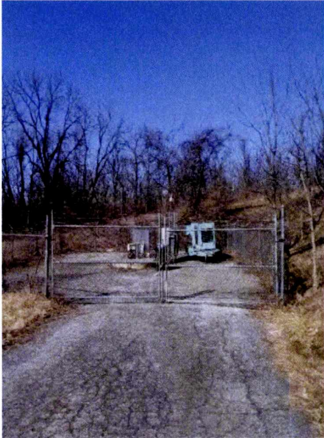
Figure 1 – Pump Station Site
