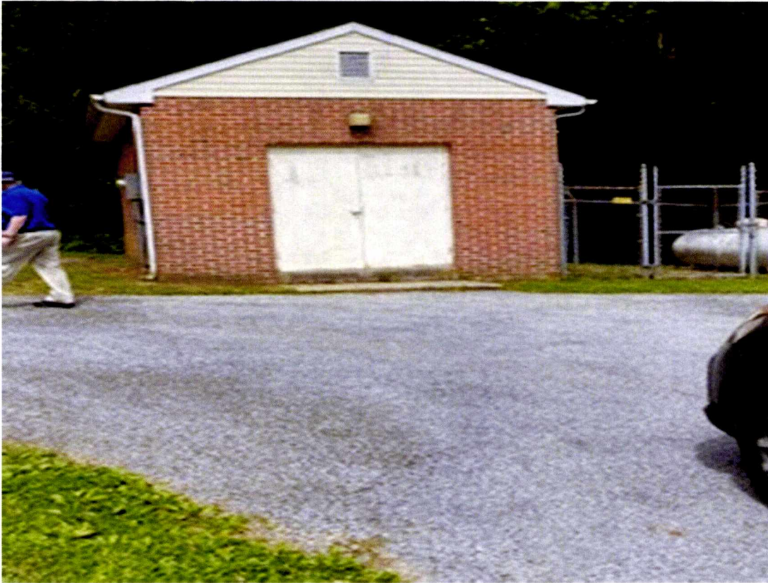
Country Ridge Sewer Pump Station
