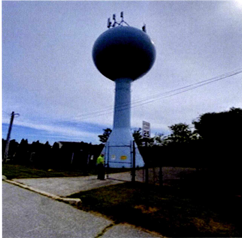
Valley Springs Water Tank
