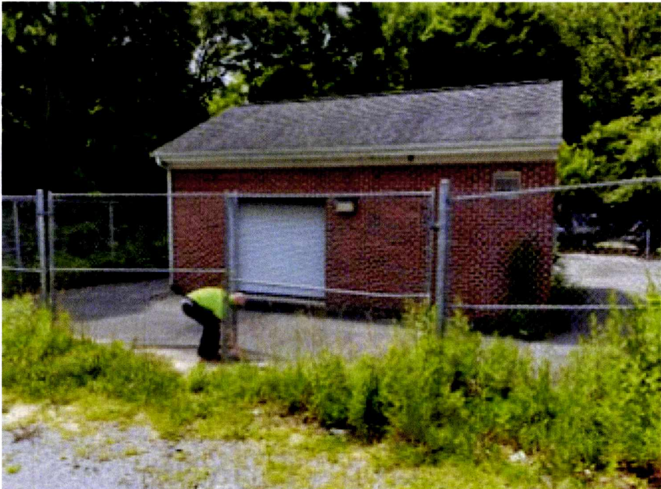
Rock Run Sewer Pump Station
