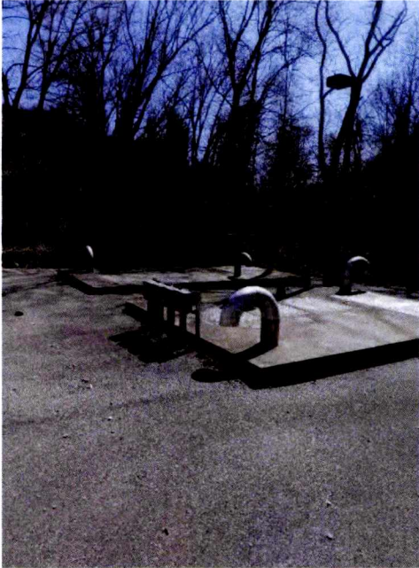
Figure 1 – Wet Well Exterior
