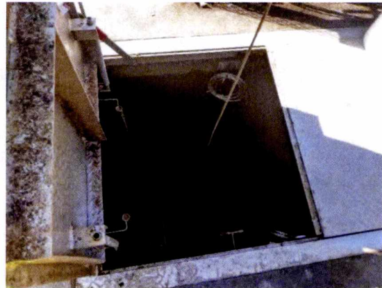
Figure 2 – Wet Well Interior
