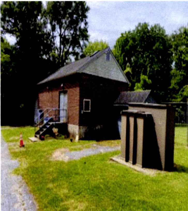
Mineral Springs Water Treatment Plant
